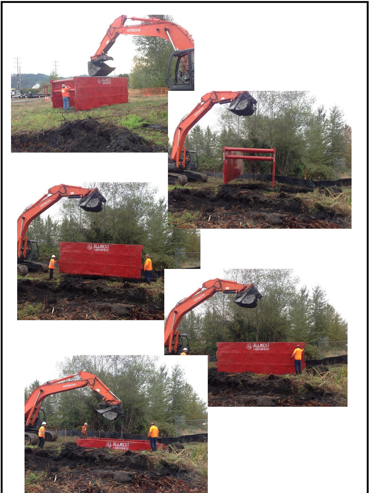
Photo 9-13 – Setting trench box sequence.
