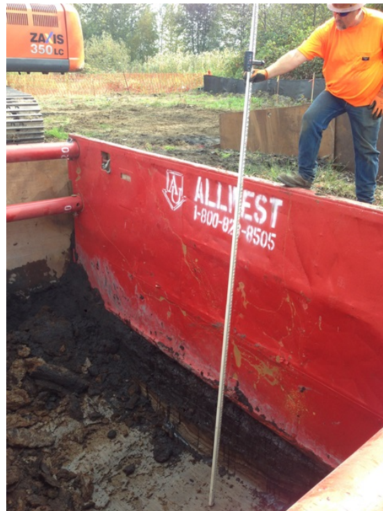
Photo 8 – Vertical control of excavation subgrade with preset grade laser and rod.
