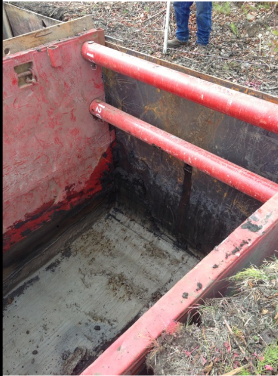
Photo 19 – Excavation subgrade. Note native gray silt – distinct from darker overlying soils.
