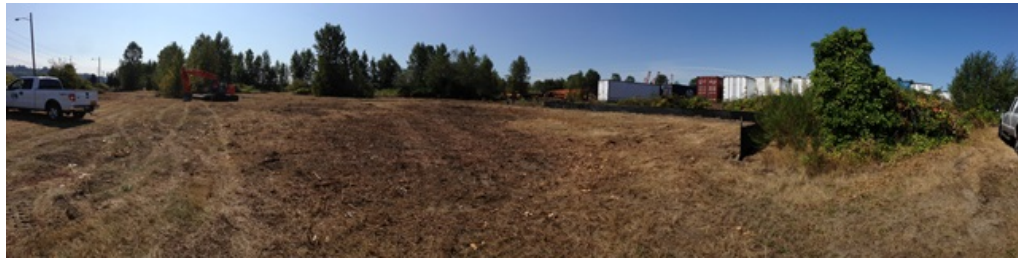
Photo 1 – View to the west of cleared and grubbed work site.
