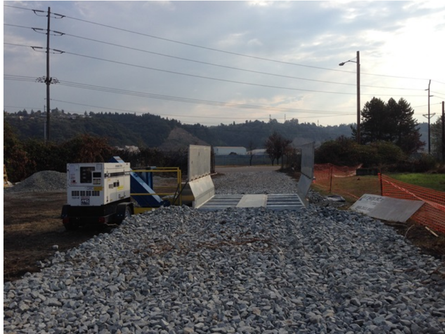
Photo 4 – Haul road and wheel wash.
