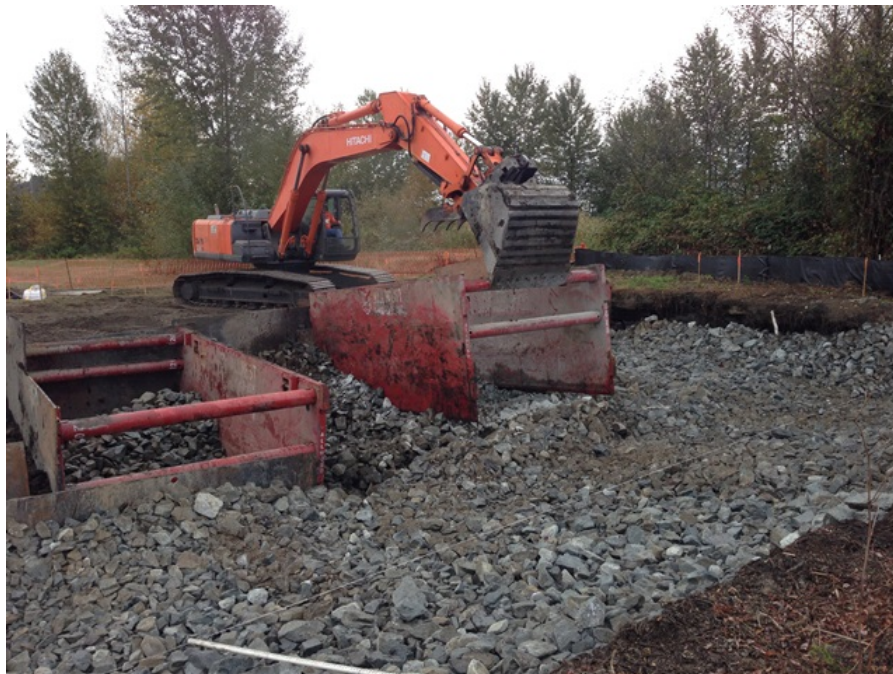
Photo 21 – Backfilling with quarry spalls.
