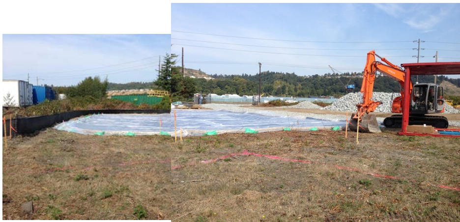
Photo 5 – Laydown and staging area.
