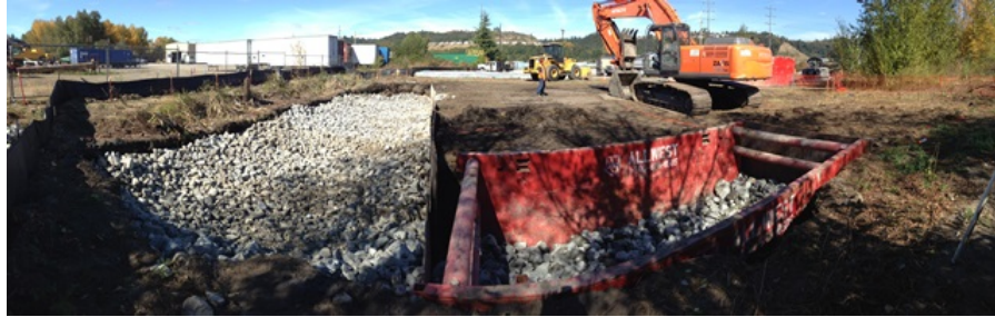
Photo 23 – General progress photo looking east.
