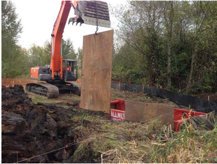
Photo 14 – Setting shoring sheets.
