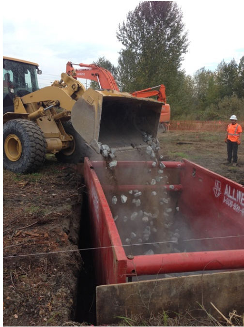
Photo 21 – Backfilling with quarry spalls.
