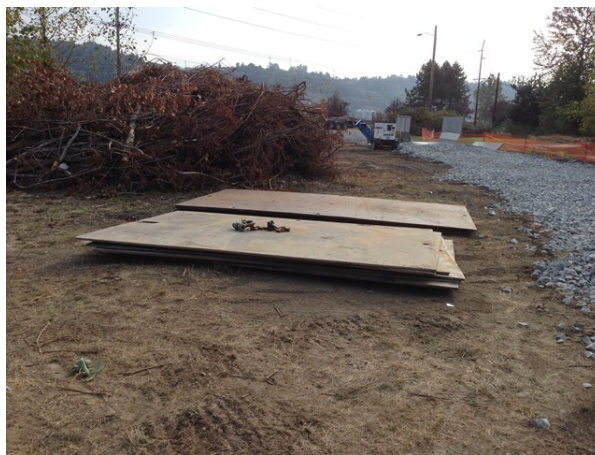
Photos 2, 3 – Trench box and plates used for excavation shoring.
