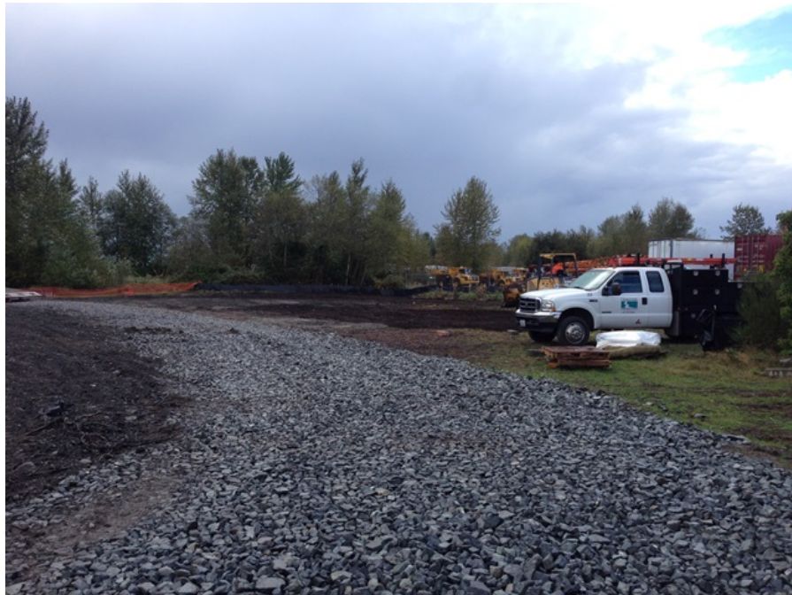
Photo 24 – completed backfill with topsoil looking west.
