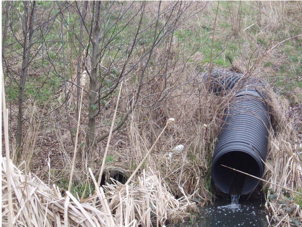
Photograph 4: City of Burien storm drain outfall and adjacent concrete outfall.
