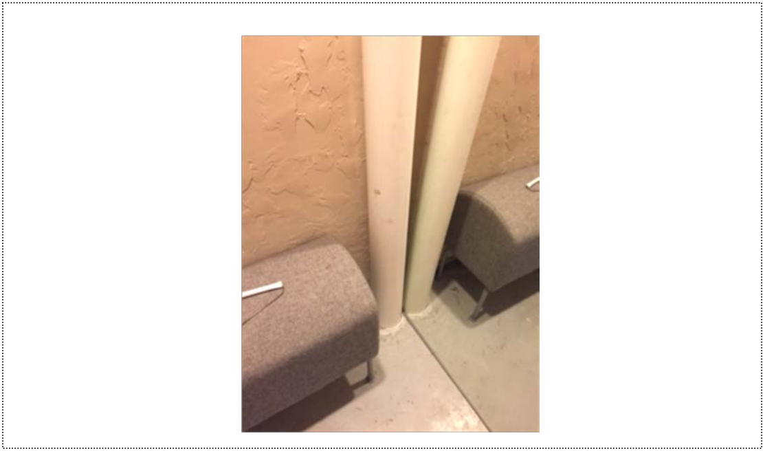
Photograph 3 – Sub-slab suction pit (VE-SS) riser outside of equipment area in Morrell's Dry Cleaners.
