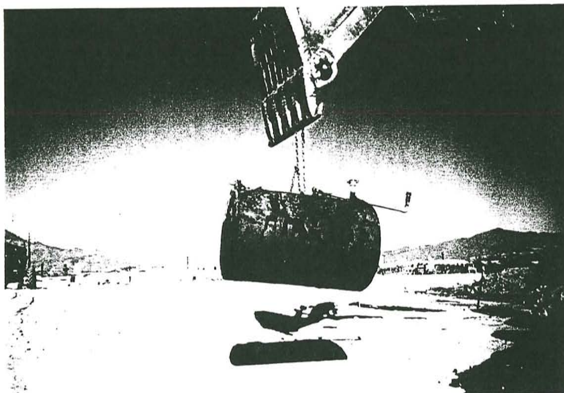
Photo 2 Former UST removed.
