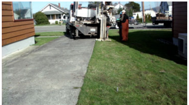
Photo #6: Close-up view of subsurface investigation at boring B-3. Note the top of a gray PVC screen at boring B-2, in the foreground. (view looking to the north).
