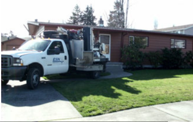
Photo #7: View of direct push probe drilling at boring B-4, inferred downgradient north-northeast of former fuel tank (looking to the south).
