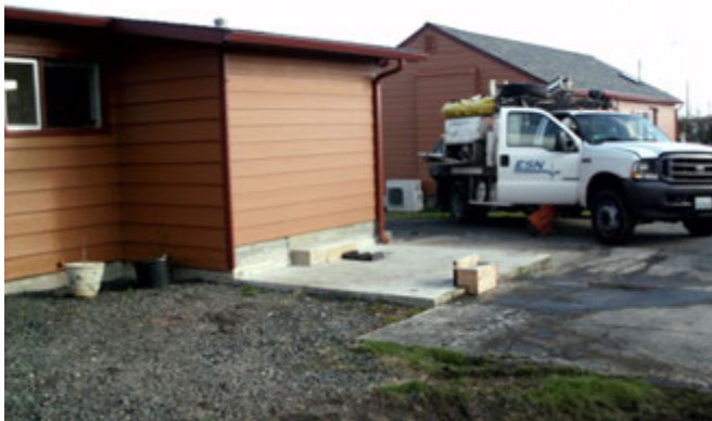
Photo #3: View of direct push probe drilling at boring B-2, inferred downgradient east of former fuel tank (looking to the east).
