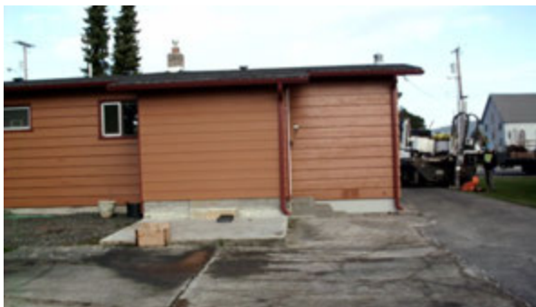
Photo #5: View of direct push probe drilling at boring B-3, inferred downgradient northeast of former fuel tank (looking to the northeast).
