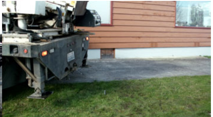
Photo #4: View of attempt to collect groundwater at boring B-2 via leaving a temporary PVC screen in the subsurface for at least 3 hours.
