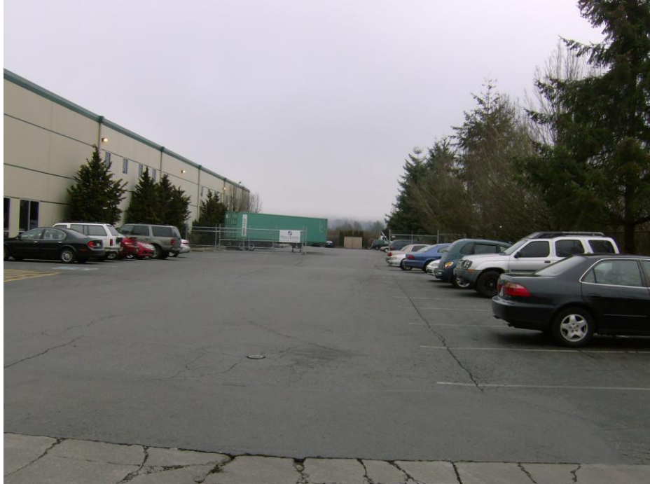
Photo 5. SW corner of MITCO building, looking at entrance to the east
