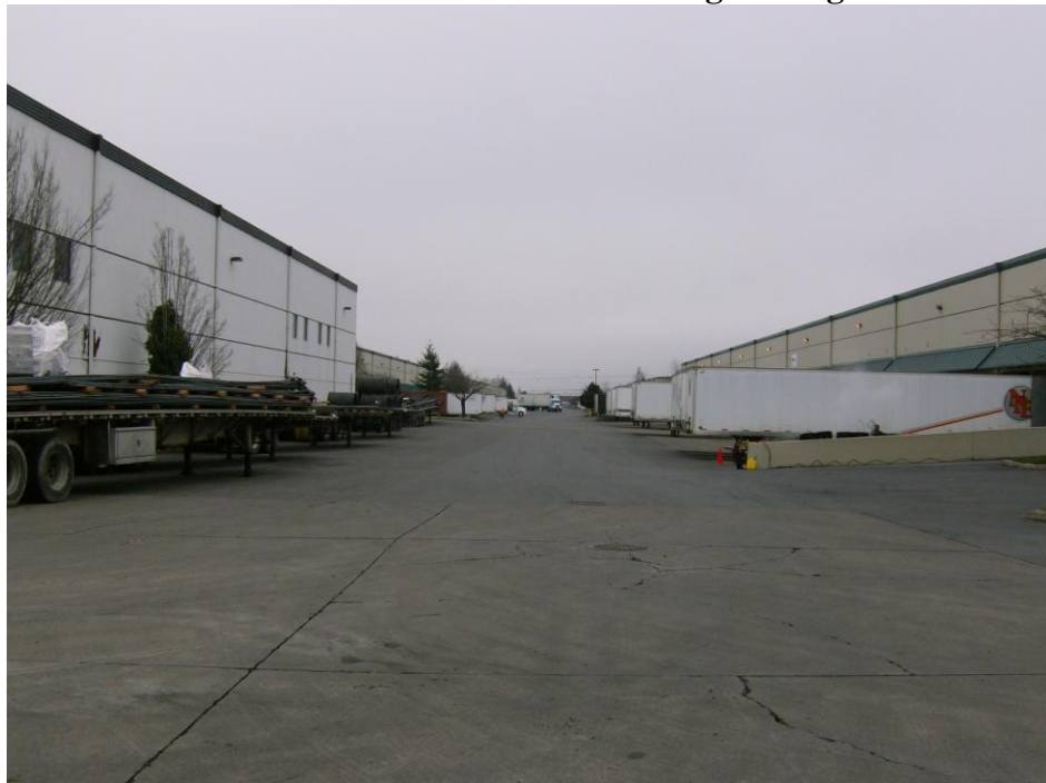
Photo 6. SW corner of MITCO building looking north.
