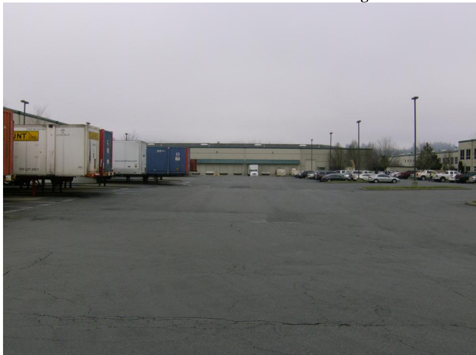
Photo 4. NE corner of MITCO lot looking west
