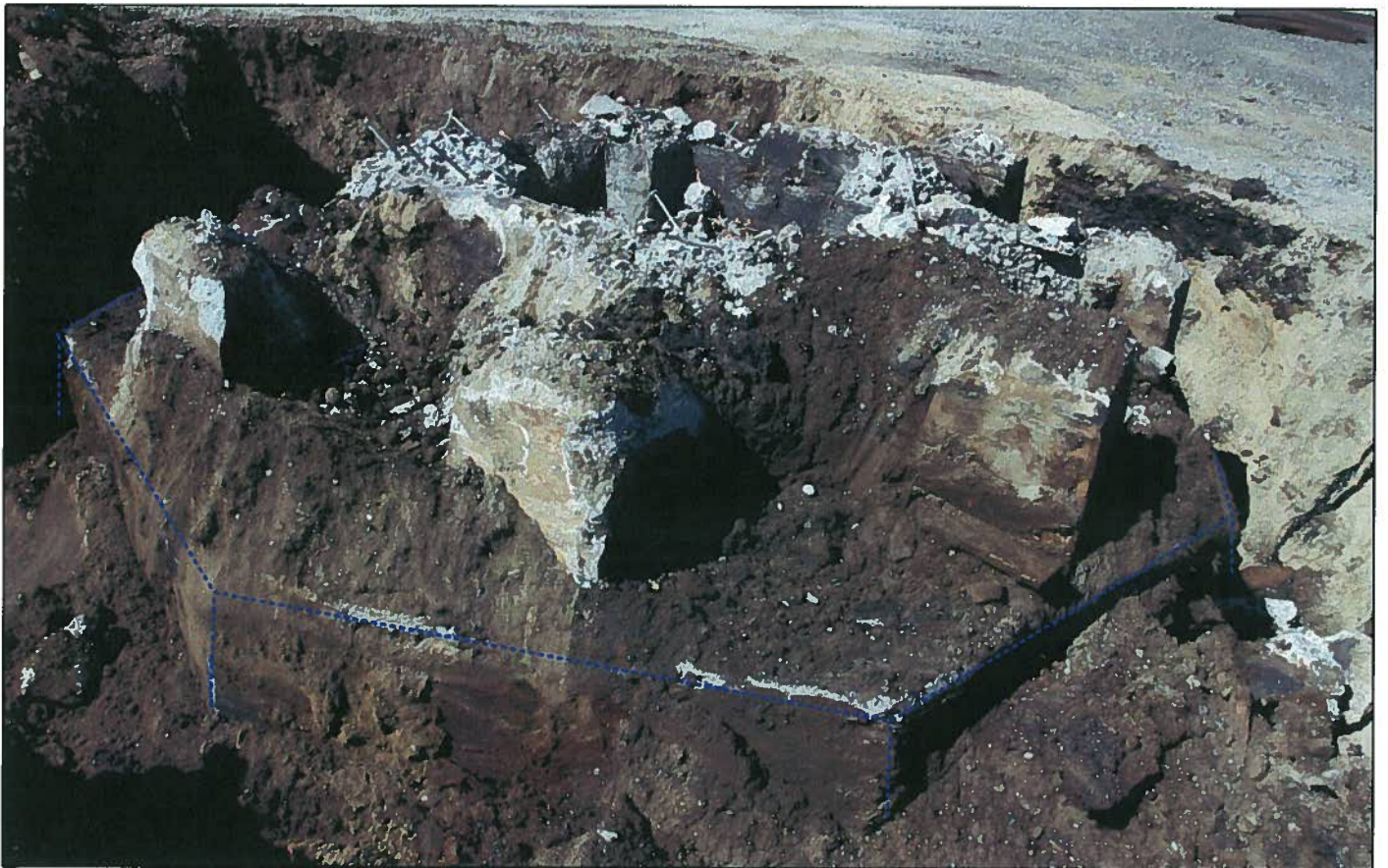
Photograph 4. Partially demolished vault structure and exposed octagonal foundation.
