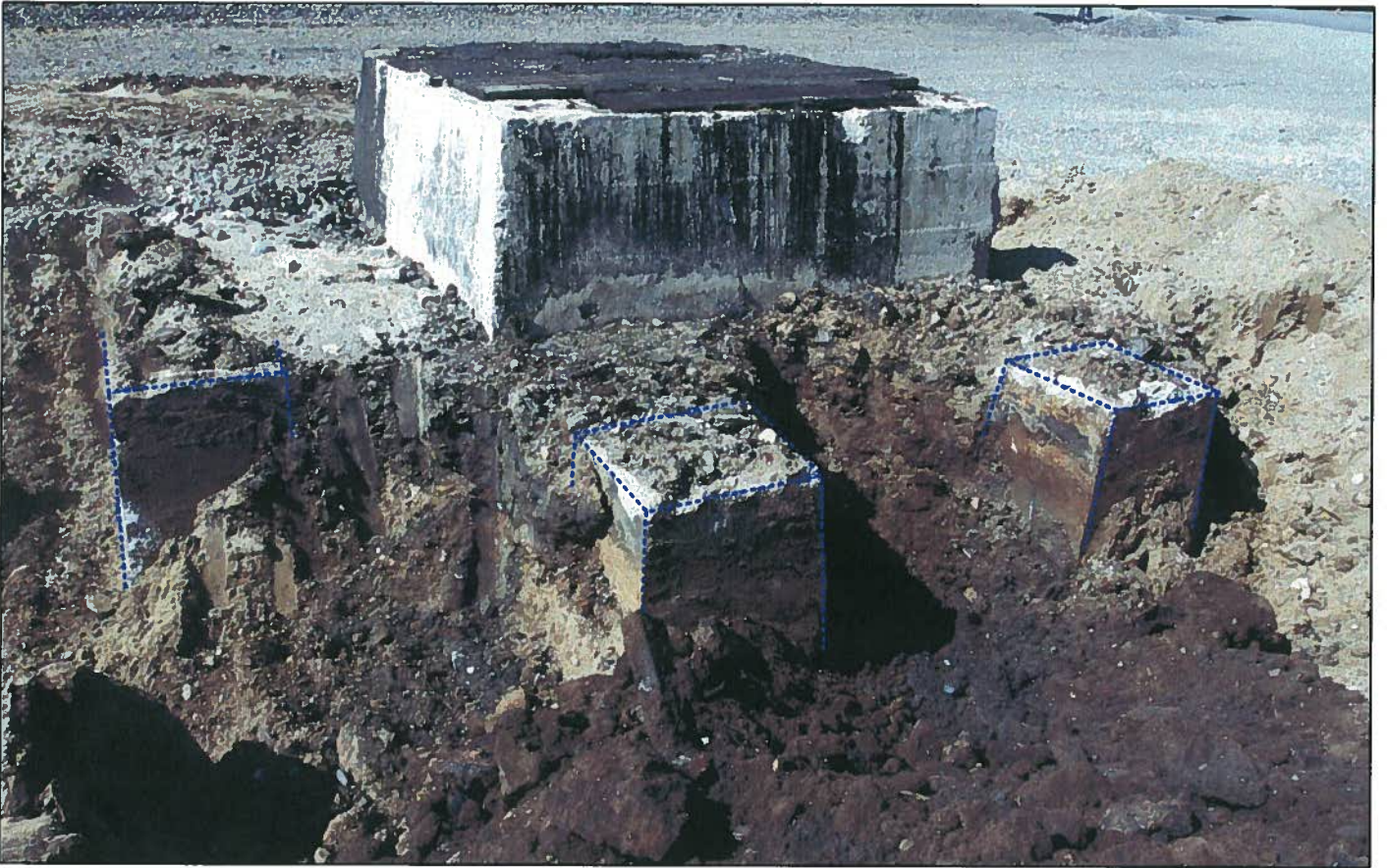
Photograph 3. Concrete vault structure and exposed support posts.
