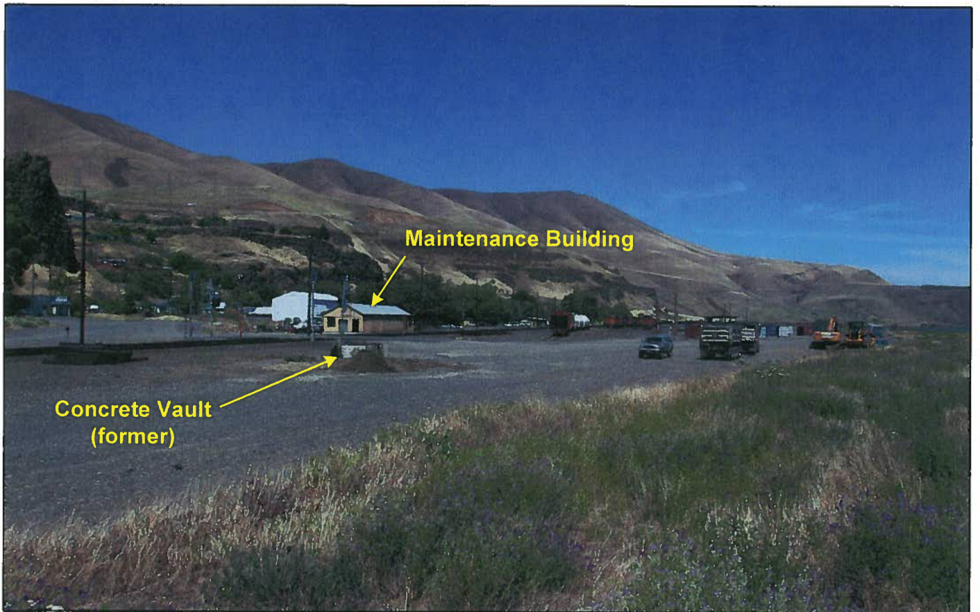
Photograph 2. Vault excavation work area overview, view to the northeast.
