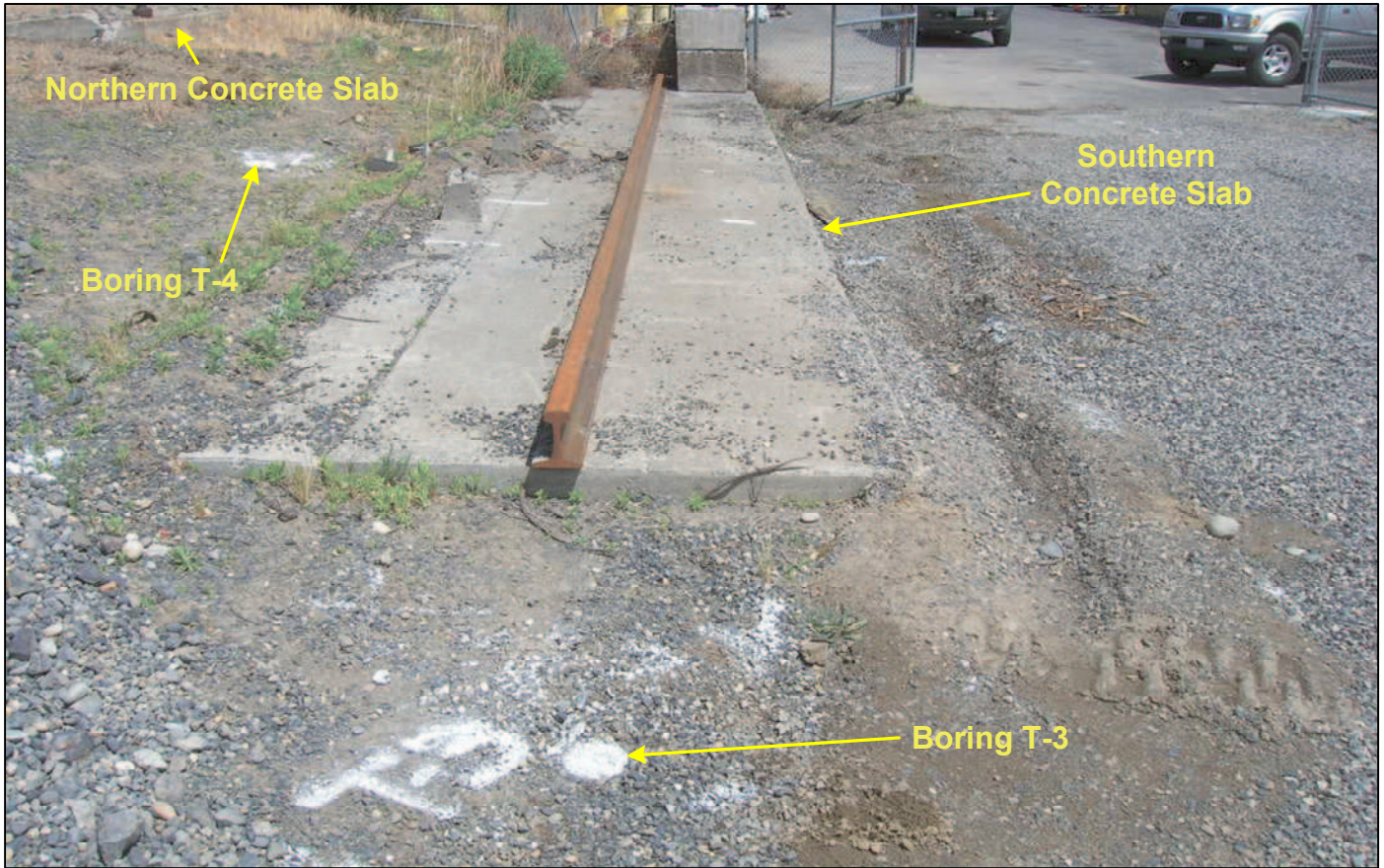
Photograph 3. Southern slab and T-3 / T-4 area, view to the east.
