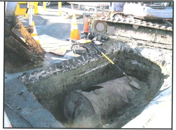
**Description:** View of UST after having been uncovered, triple-rinsed, and inerted.
