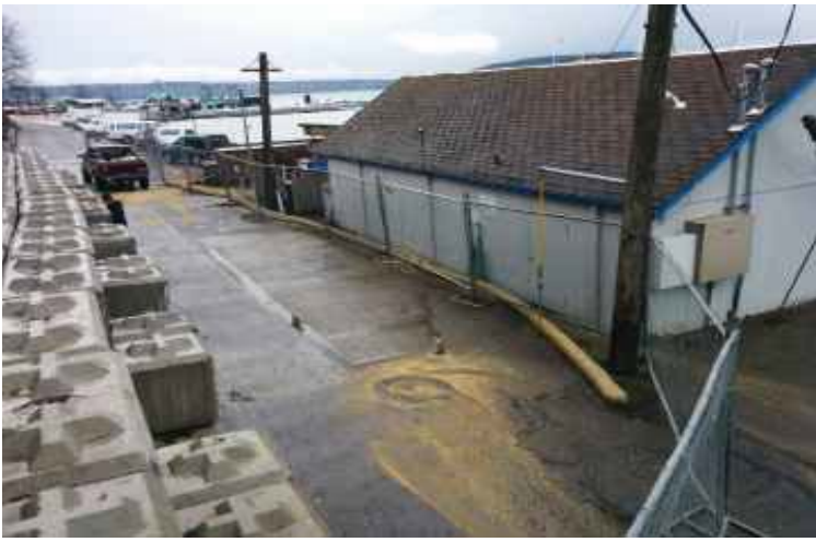
Photograph 01: UST Locations - View North west
