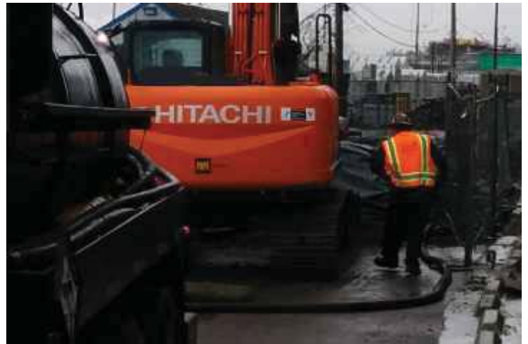
Photograph 14: Pumping impacted water from Excavation
