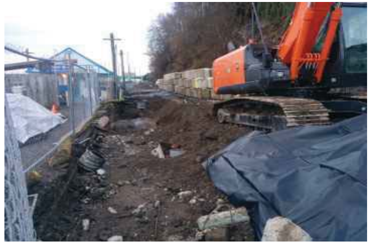
Photograph 08: Removal of 3000 gallon UST three - View South east
