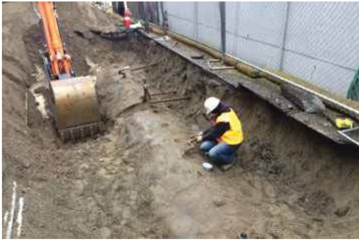
Photograph 03: Preparing USTs for Removal - View North west
