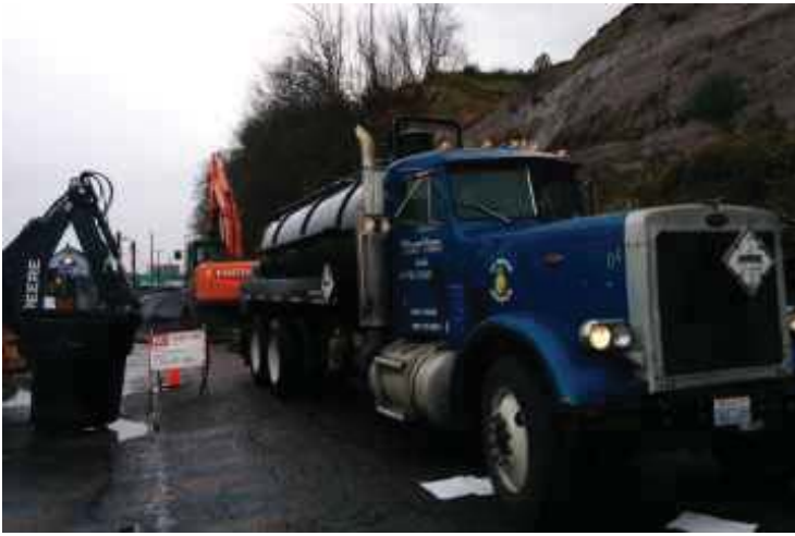
Photograph 13: Pumping impacted water from UST Excavation
