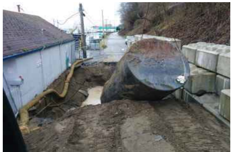
Photograph 05: Removal of 3000 Gallon UST One - View South east
