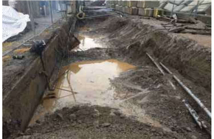
Photograph 16: Excavation area following dewatering activities - View South
