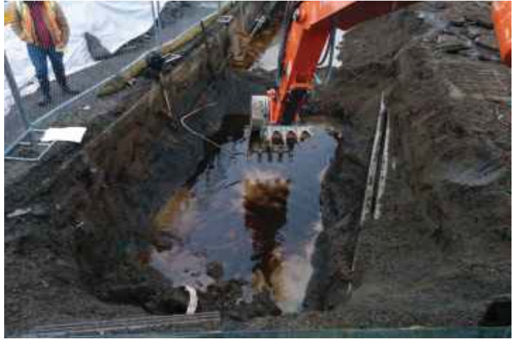
Photograph 12: UST four and five excavation following UST removal - View South
