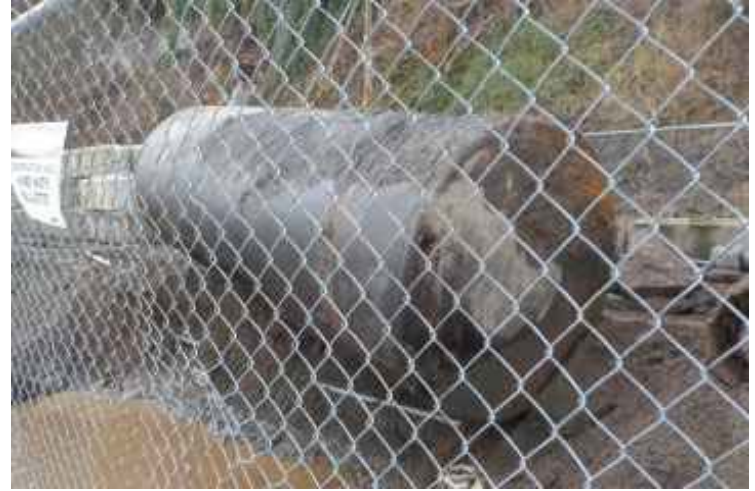
Photograph 10: Removal of 8000 gallon UST four - View East
