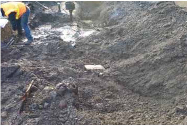
Photograph 07: Preparing UST three for removal - View South east
