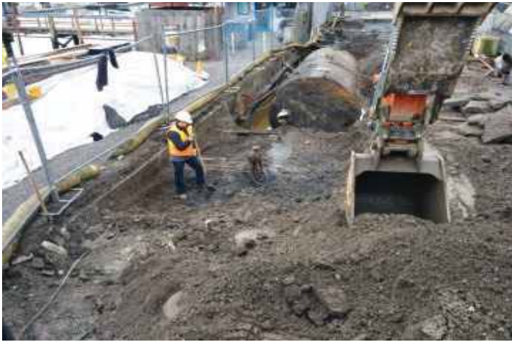
Photograph 09: Excavation of USTs four and five - View South
