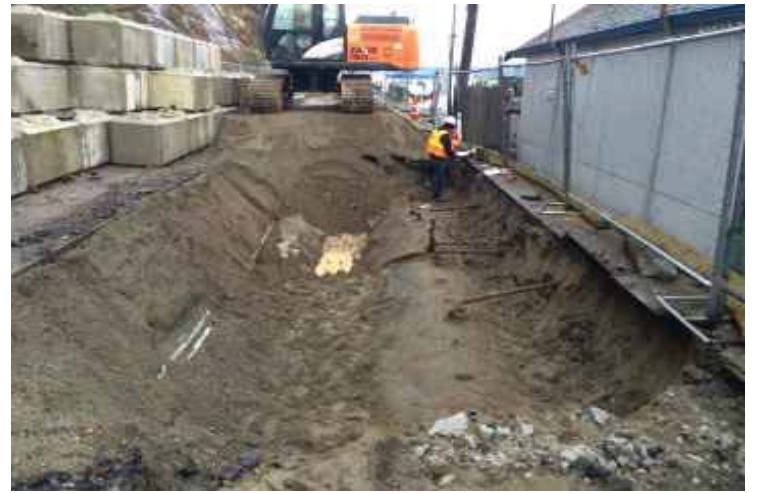
Photograph 04: Preparing USTs for Removal - View North west
