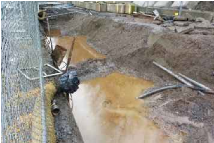
Photograph 15: Continued pumping of impacted water from excavation
