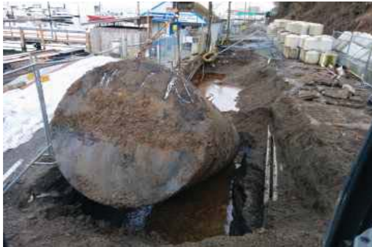
Photograph 11: Removal of 8000 gallon UST five - View South east
