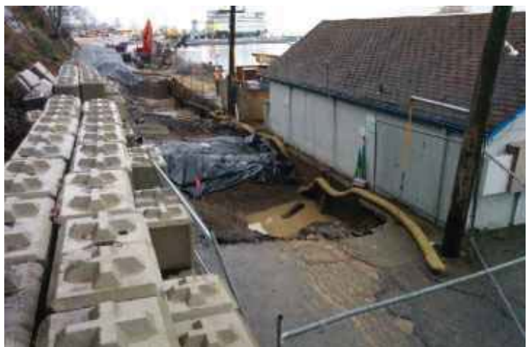
Photograph 18: Excavation area post UST removal - View North
