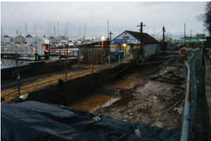
Photograph 17: Excavation area post UST removal - View south
