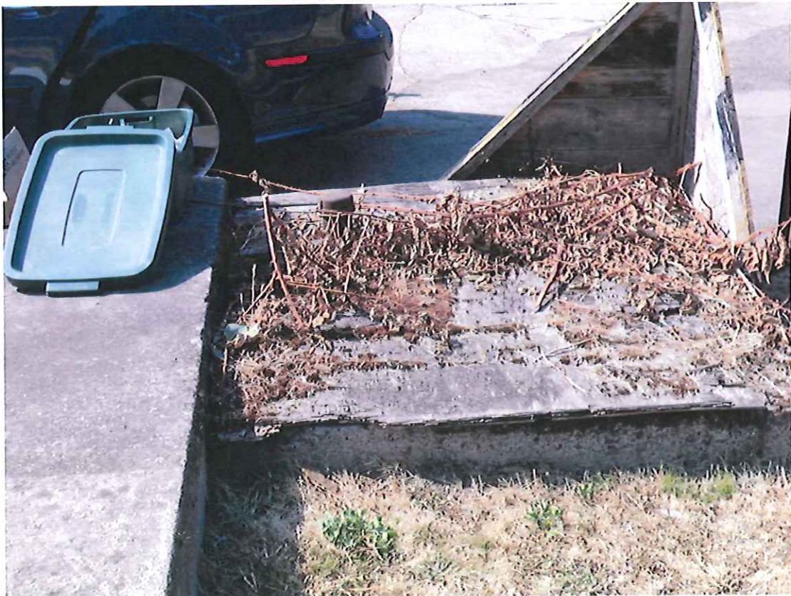
Photograph 2: View of the Federal Center South heating oil UST fill port on the north side of the Federal Center South UST 1. This may indicate the presence of a fourth tank at the Federal Center South facility.
