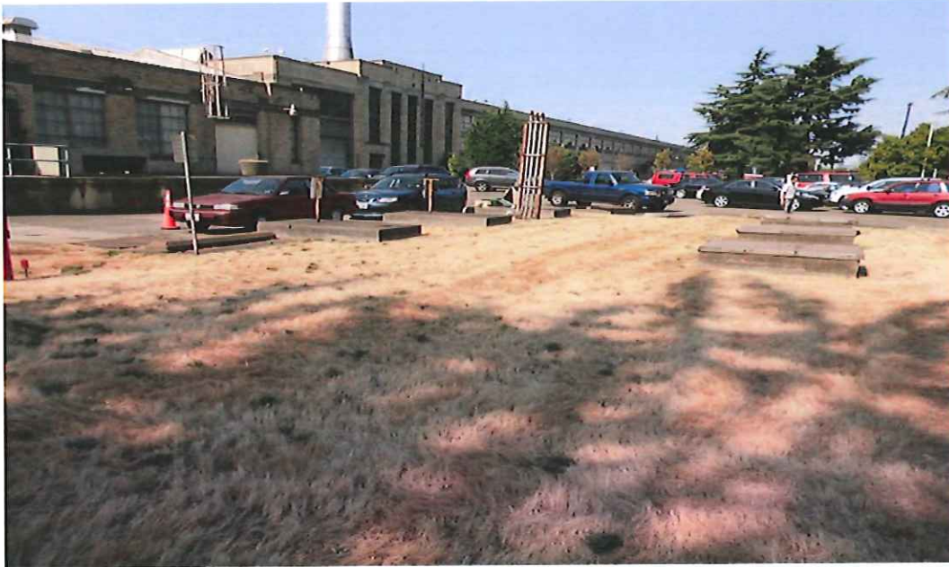
Photograph 1: View of UST vent and fill vaults and the three tanks vents. Building 1206 is seen to the left of the UST structures and Building 1201 is in the background right.
