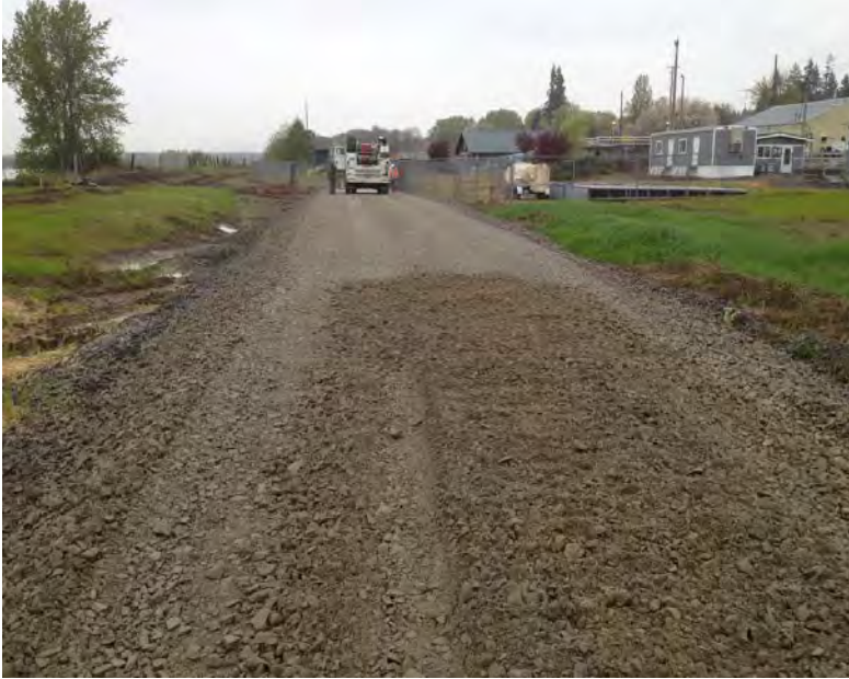
Photo 1: Crushed rock placed on roadway
