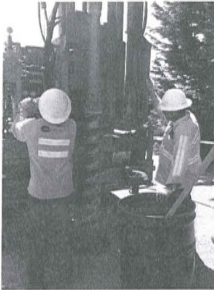
Drilling a new extraction well
