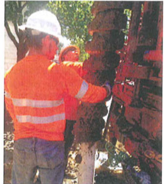
Installing MW-9R for petroleum contamination removal.
