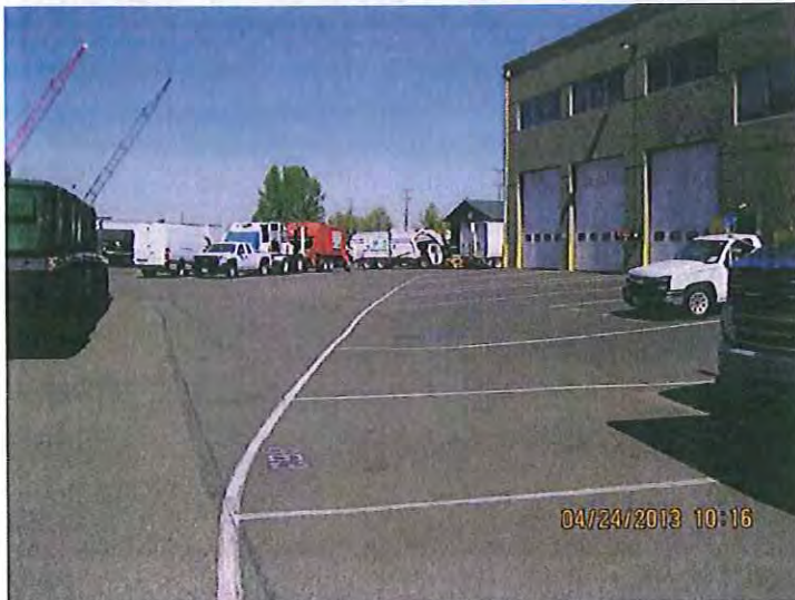
#1. DESCRIPTION: Wastes are transferred between trucks and the warehouse. Truck maintenance takes place in the north 3 bays of the main building. There are no known connections between the interior floor drains and the storm drain system.
