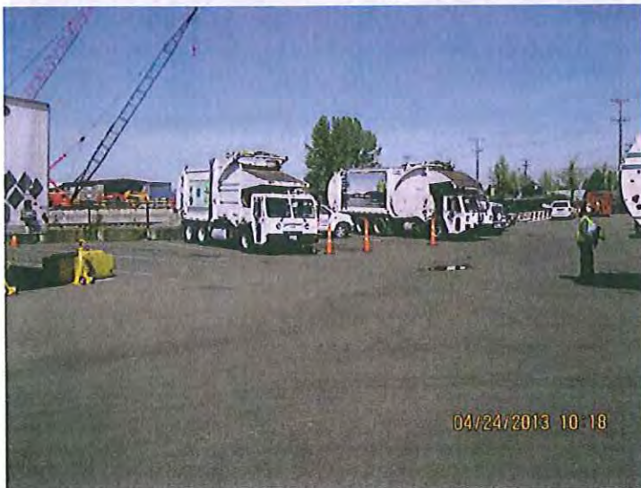
#3. DESCRIPTION: The storm filter treatment vault is located in the ground near orange cones. All stormwater from the site flows to the storm filter treatment system except what comes off the roof. The facility should sample and analyze roof run-off to confirm that pollutants are not going to the river without treatment.
