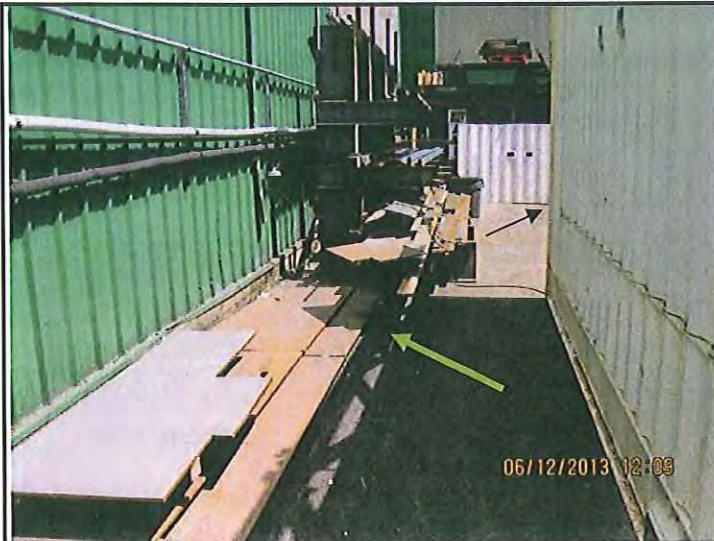
#13. DESCRIPTION: The storm drain catch basin indicated by the black arrow is mapped to be connected to the sanitary sewer. The manhole under the steel plates (green arrow), does not have a mapped connection in the site map. The drains and structures in this area should be verified and accurately reflected on the site map.
