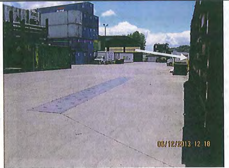
#14. DESCRIPTION: The slotted metal plate is the wash pad. Vehicles and equipment are washed and fueled here. A tanker truck is situated on a shipping flat, white arrow, just out of view (see also Photo # 16). It is used for fueling forklifts. An off-site mobile fueler comes on site to refuel large equipment at this location. This pad was later determined by Seattle Public Utilities to have a connection to the storm drain system
