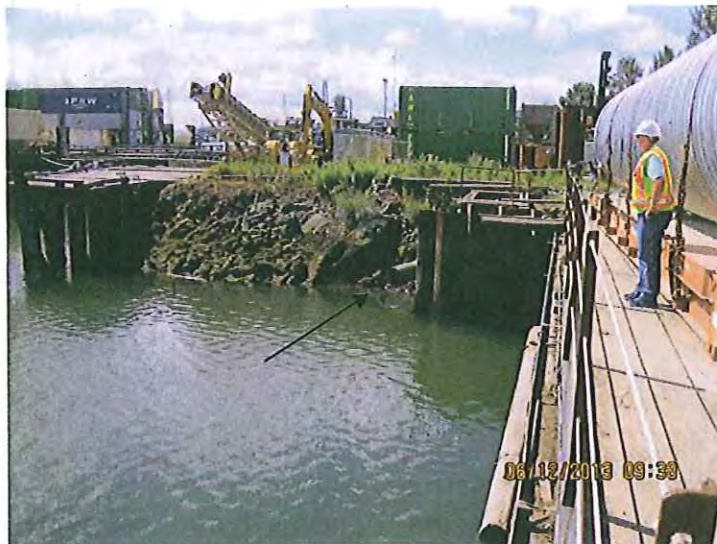
#3. DESCRIPTION: The treatment system and tanks seen in Photos # 4 -6 are located just beyond the silver pipe. Outfall # DP-2 (arrow) discharges here.
