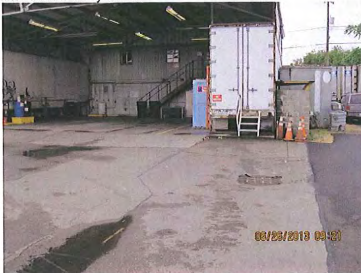
#3. DESCRIPTION: Maintenance of packer cranes and other equipment generally occurs under a roof, but some activities take place outdoors for cranes that cannot fit completely under the roof.
