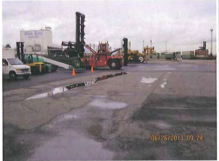
#2. DESCRIPTION: At the south end of the facility is the packer maintenance shop. All catch basins have filter inserts in them.
