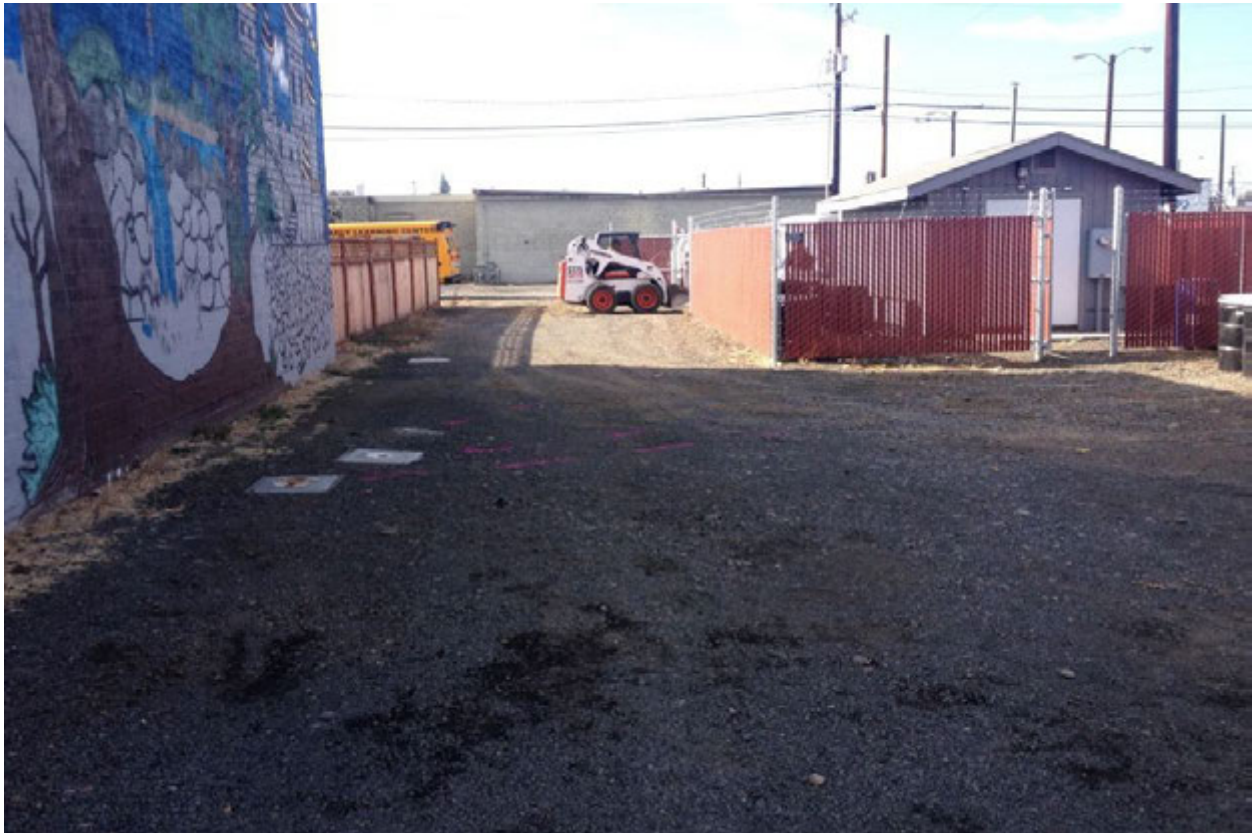
Photograph 1 – Former Frank Wear Cleaners site conditions prior to beginning construction. Children’s daycare building on the left, SVE system on the right. Photograph taken facing west.
