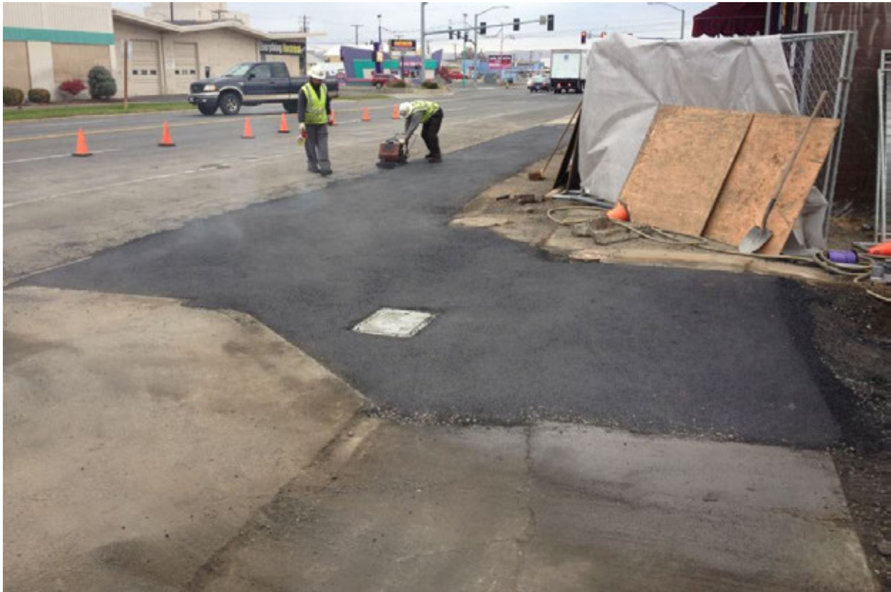
Photograph 23 – Extraction well trench surface completed using hot asphalt. S 3rd Ave is on the left, the Site and children’s daycare are on the right. Photograph taken facing south.
