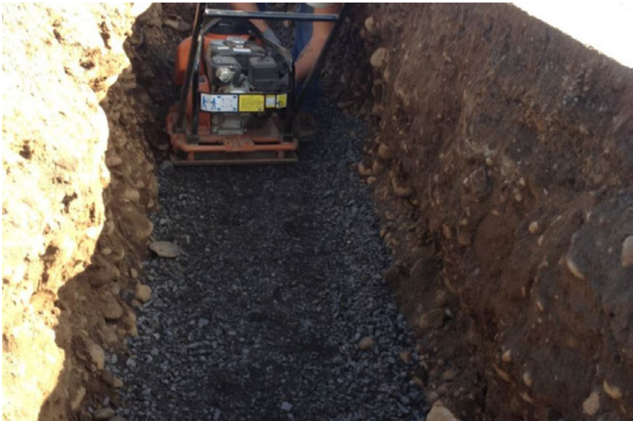
Photograph 16 – Typical trench with pipe bedding material placed and beginning compaction.
