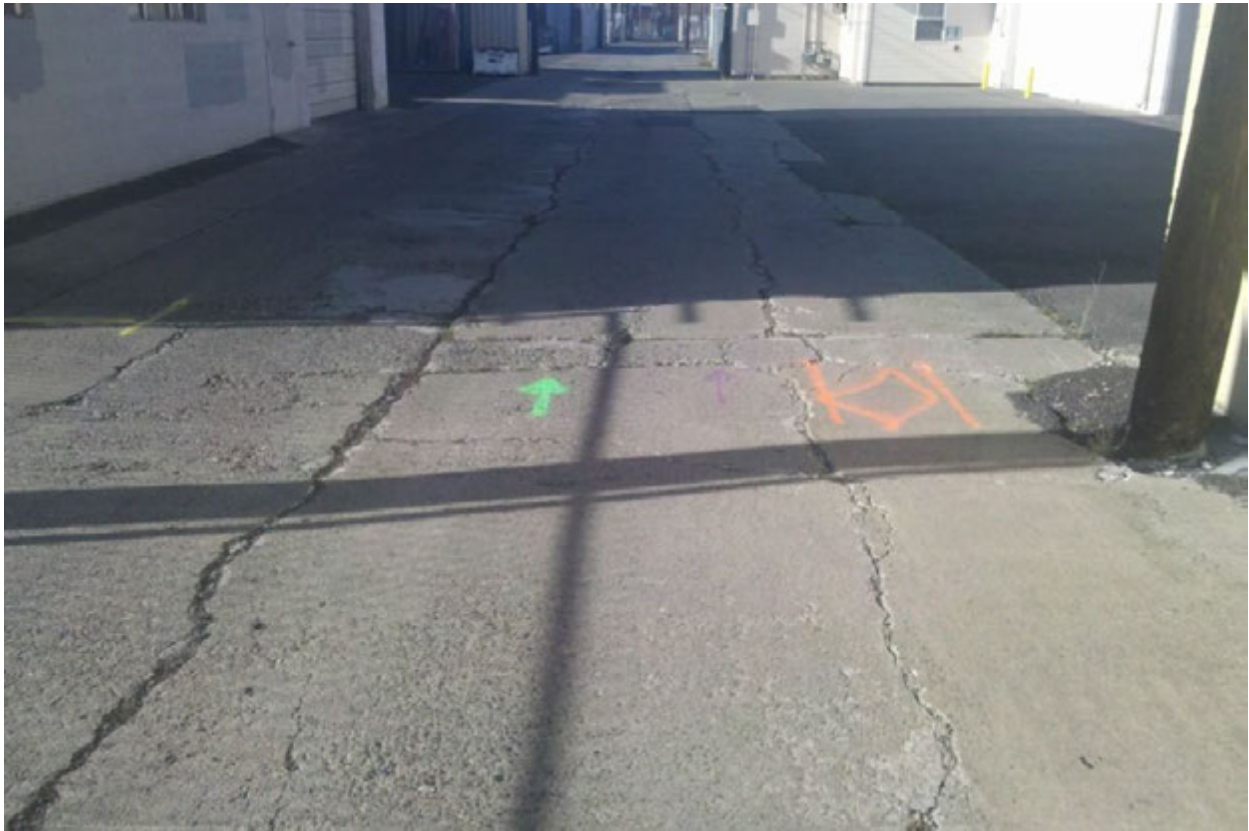
Photograph 5 – Alleyway along the west side of the Site showing multiple underground utilities including from left to right; natural gas, sewer, irrigation, and communication lines. Photograph taken facing south.
