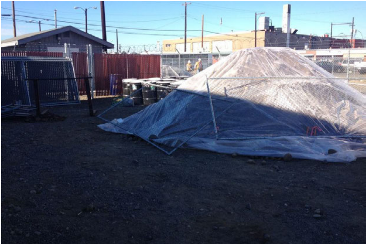
Photograph 31 – Excavated soil pile on the Site pending analysis for disposal. Photograph taken facing northwest.
