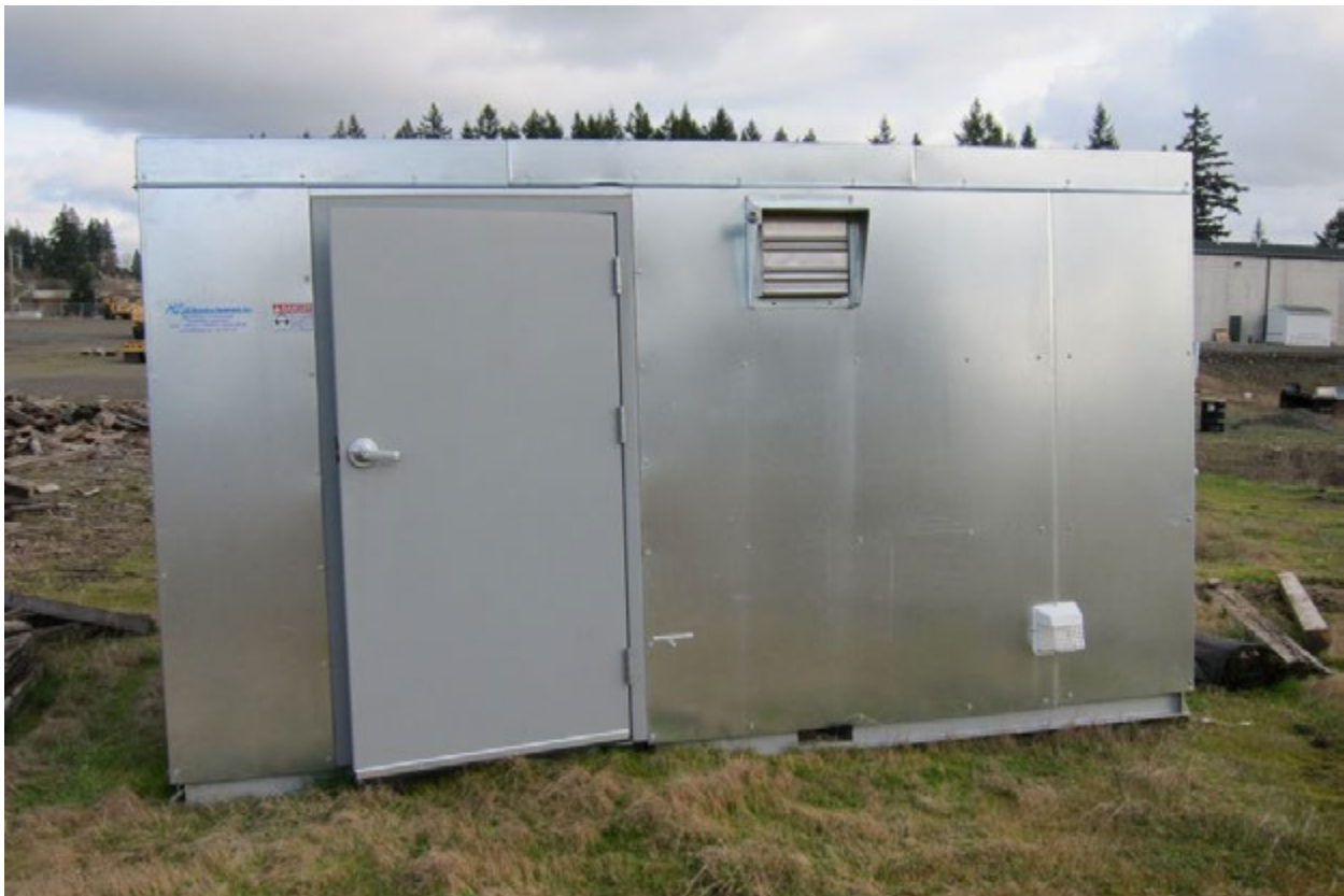
Photograph 6 – GTS prior to delivery. Photograph shows the external construction of the building including I-beam skid foundation.
