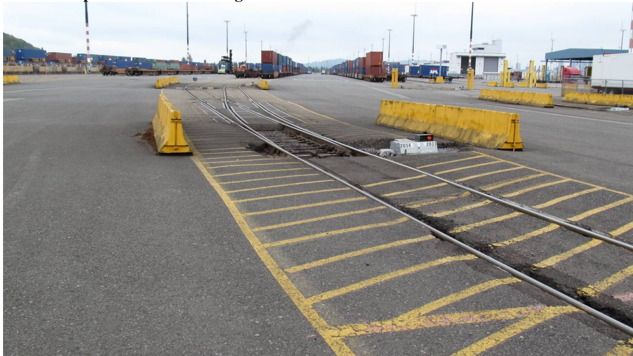
Photo 1: Asphalt Surface with Degradation Near Tracks – from the south
