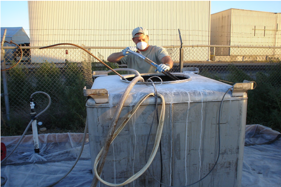
Mixing of injection solution.
