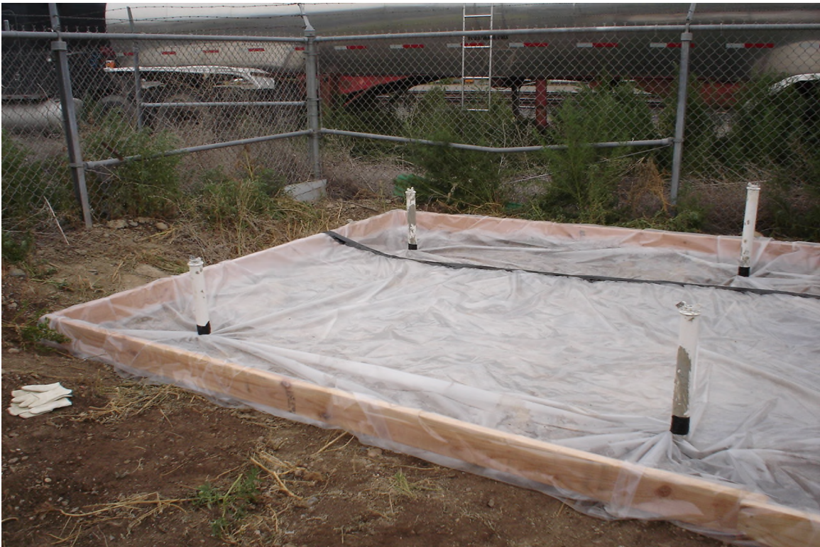
Berm constructed around injection wells.
