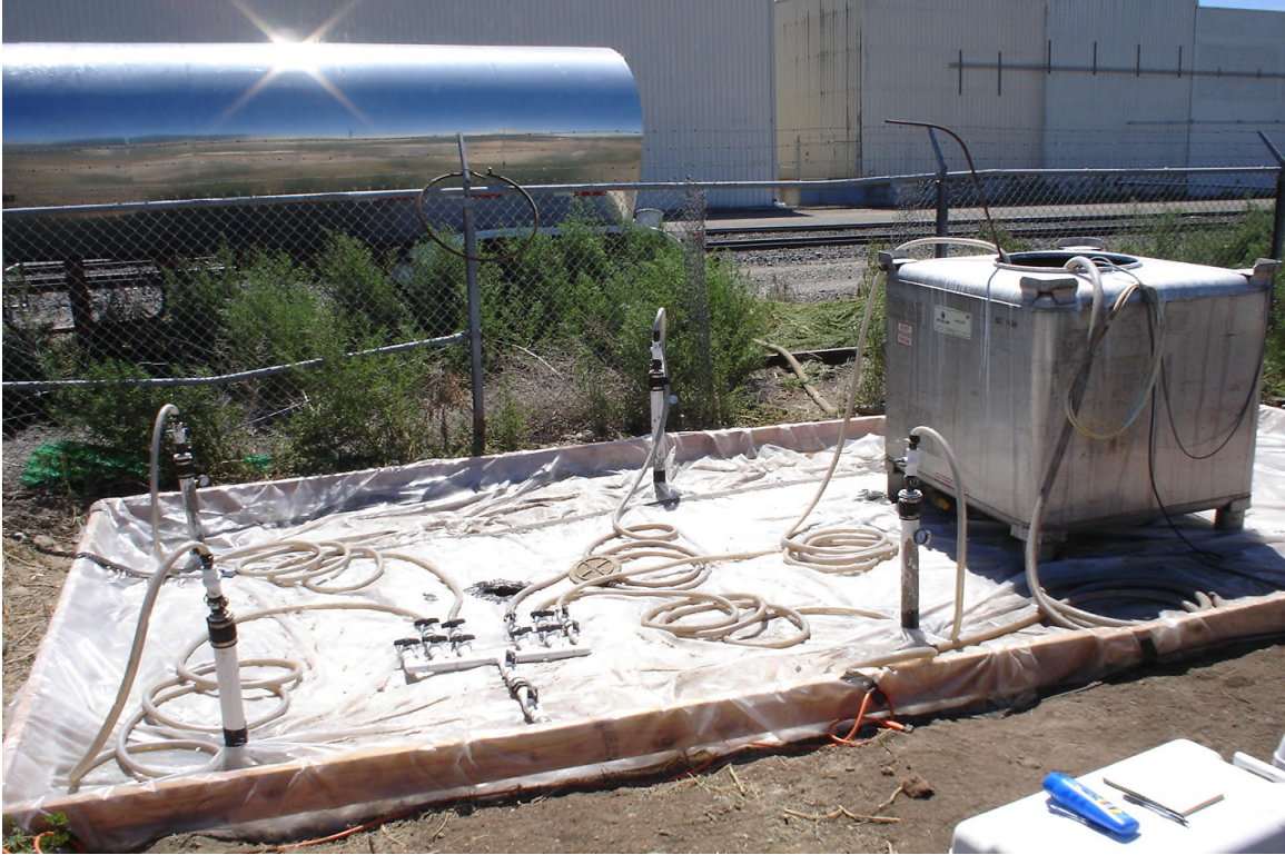
Pilot study mixing and injection system.
