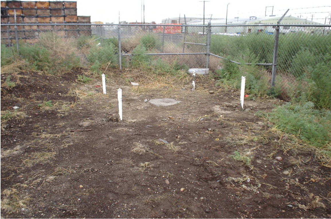
Injection wells IW-1 through IW-4 installed around MW-4.
