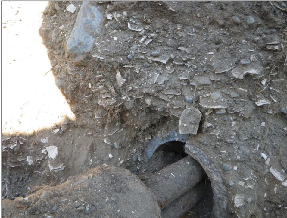
Figure 5-3. Shell layer within sand fill surrounding a concrete utility pipe found within the trench.
