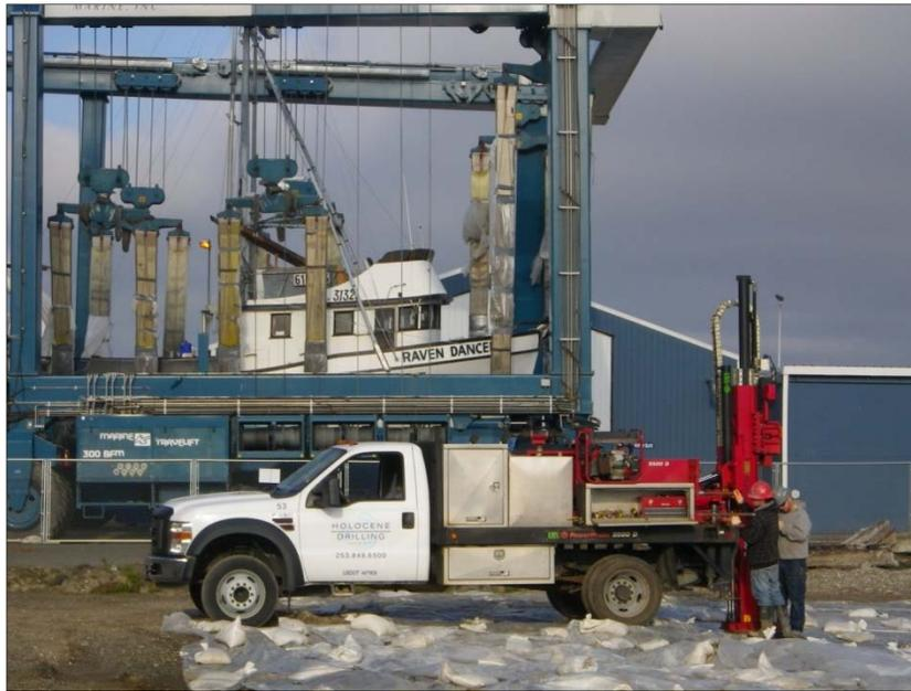
Figure 5-1. Holocene Drilling geoprobing the K Ply mill yard with the Power Probe 9500D. View west.
