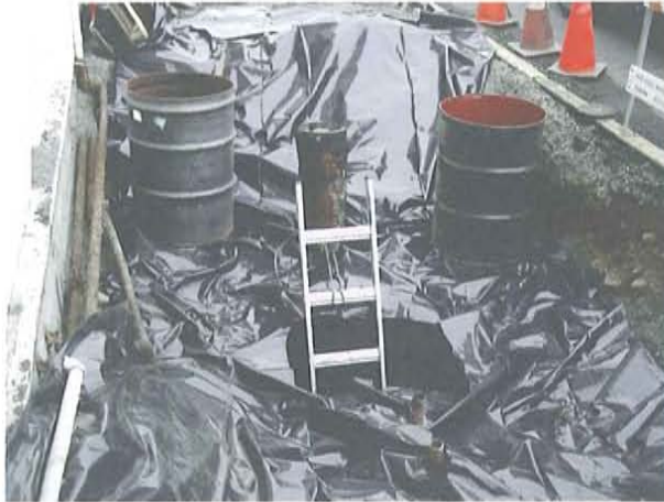
This picture shows the setup for cleaning the east tank.
