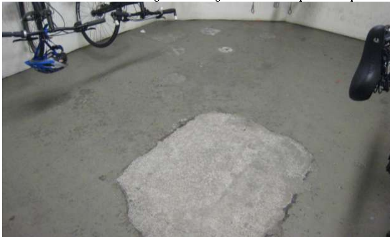
Photo 3: Another tank access cutting in bike storage room – well at top middle of picture
