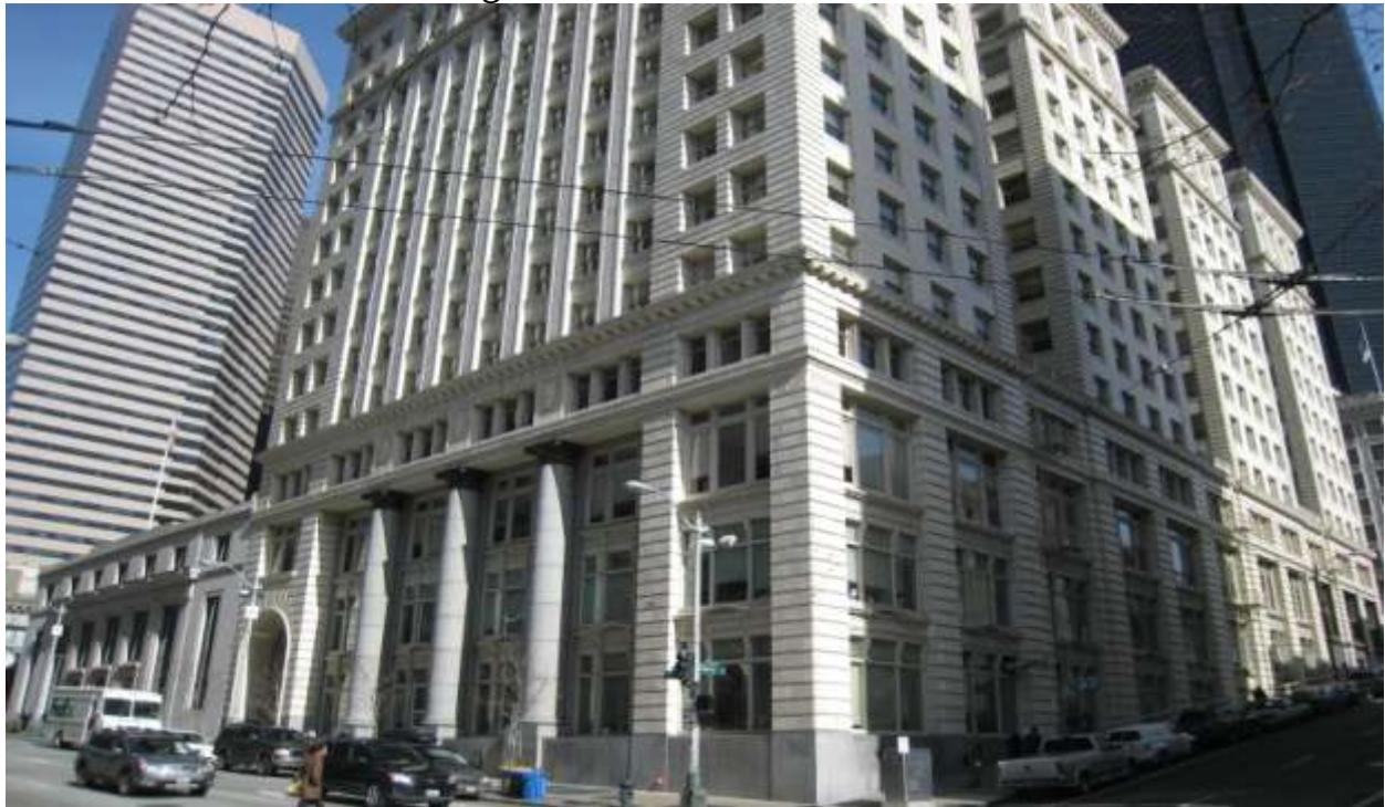
Photo 1: Dexter Horton Building - from the southwest
