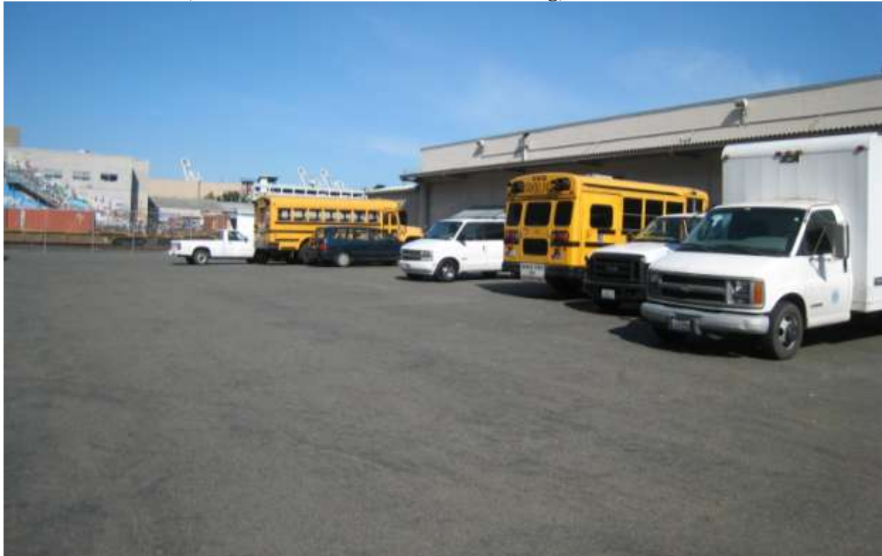
Photo 4: South side, east end of the former VMF Building, where excavations occurred
