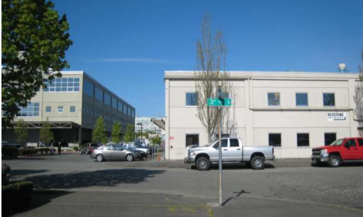
Photo 3: Former GMF Building on the left, VMF on the right - from the east across 3rd
