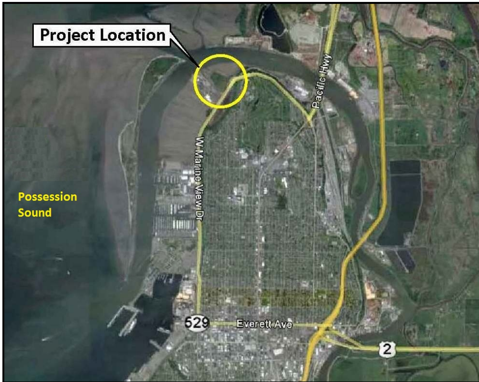
Figure 1. The Bay Wood Products Site is located at 200 West Marine View Drive on Port Gardner Bay in Everett, WA. (Figure 1-1 from the RI/FS)
