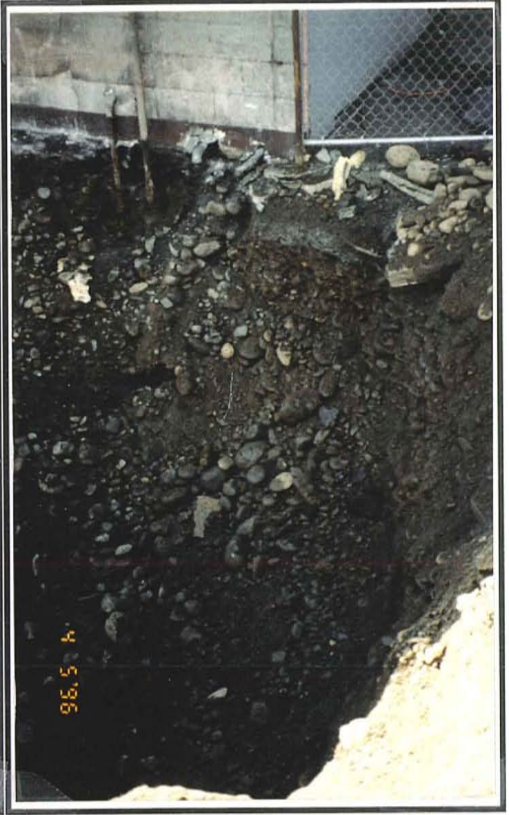
Photo 12. UST #3 excavation sidewall.
