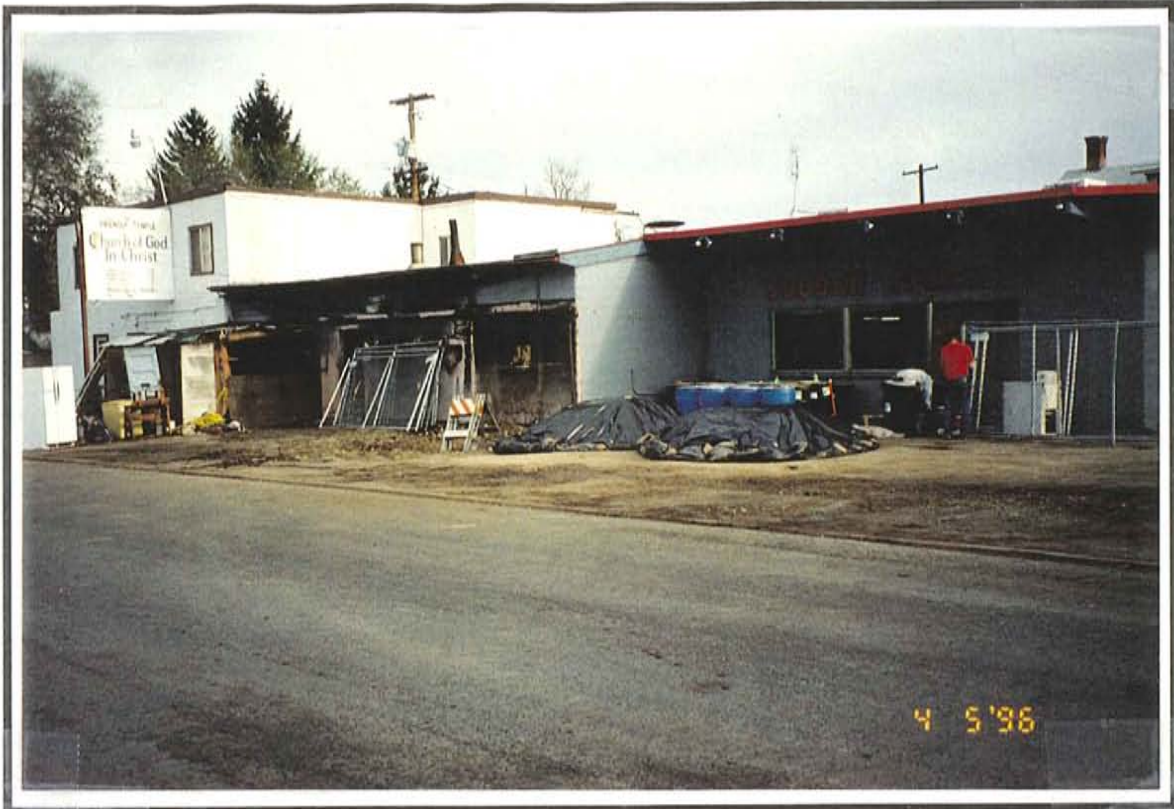
Photo 1. View southeast of site at completion excavation and backfill activities.
