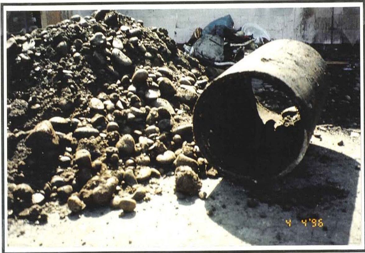
Photo 9. Sump #1 (at right) after removal.
