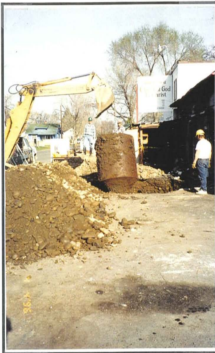
Photo 7. UST #2 being removed from excavation.
