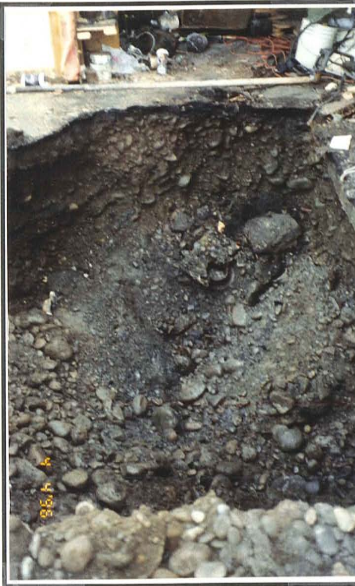
Photo 5. View east of UST #1 excavation prior to excavation of petroleum-contaminated soil.
