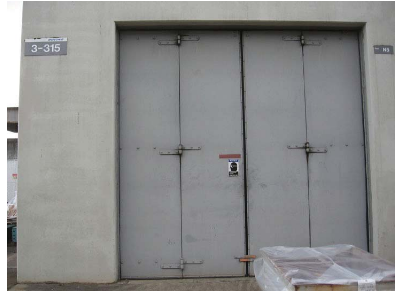
Photo 66. Rubber Gaskets on Doors at Building 3-315
