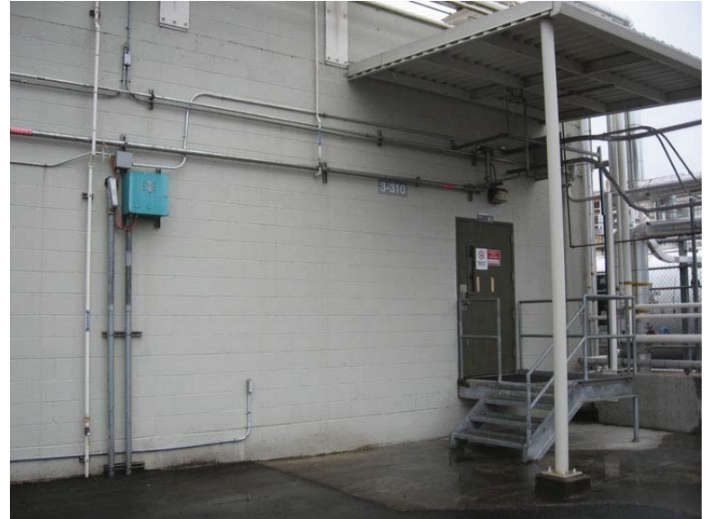
Photo 18. Example of Outdoor Utilities Lines Attached to Building Exteriors at NBF - Building 3-310 (View 1)
