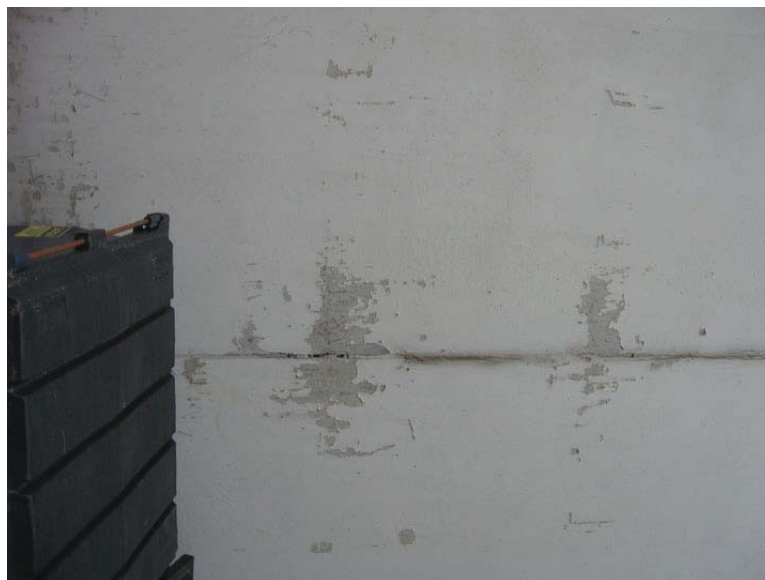
Photo 36. Degraded Paint on Building 3-315 (View 1)
