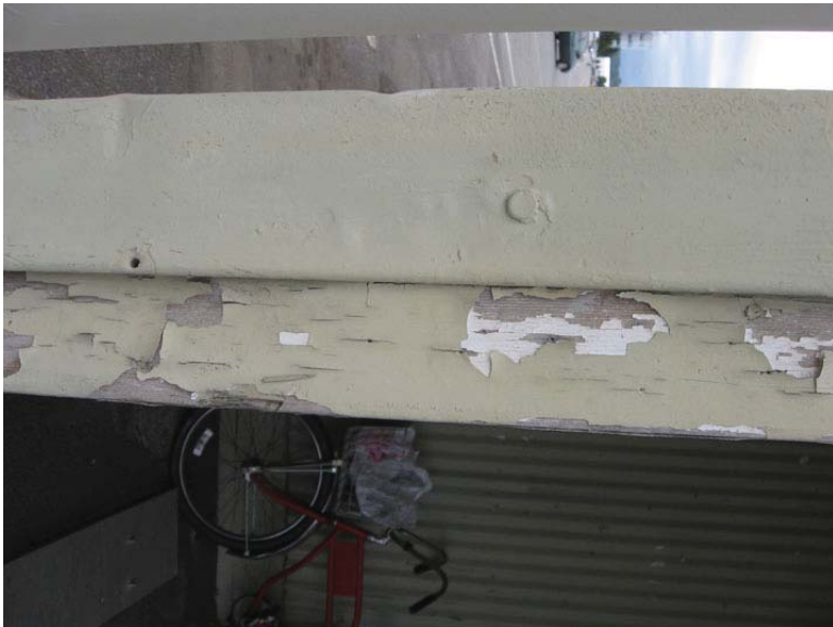
Photo 39. Degraded Paint on Building 7-027-1 - Detail of View 1
