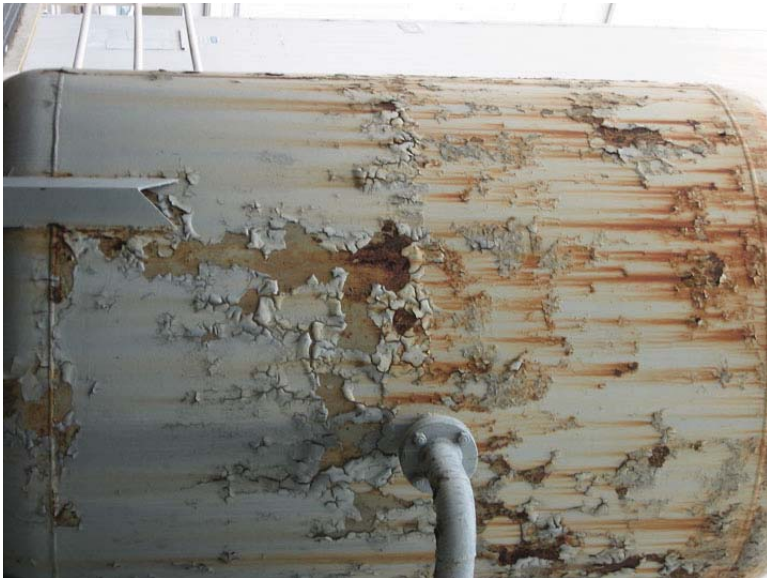
Photo 43. Degraded Paint on Tank or Boiler adjacent to Building 3-374
