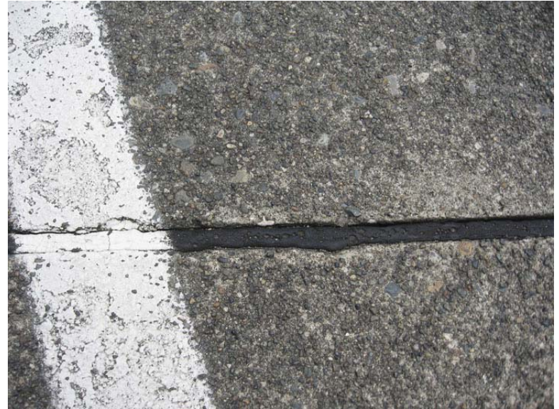
Photo 2. New Caulk with Residual Caulk on Concrete on the Flight Line
