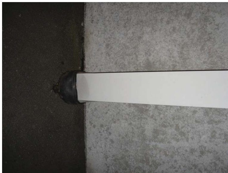
Photo 60. Roof Drain on Building 3-370 - Detail (note drain is connected to SD system)
