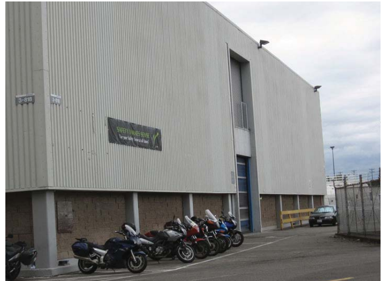
Photo 72. Concrete Block Construction and Metal Siding on Building 3-818
