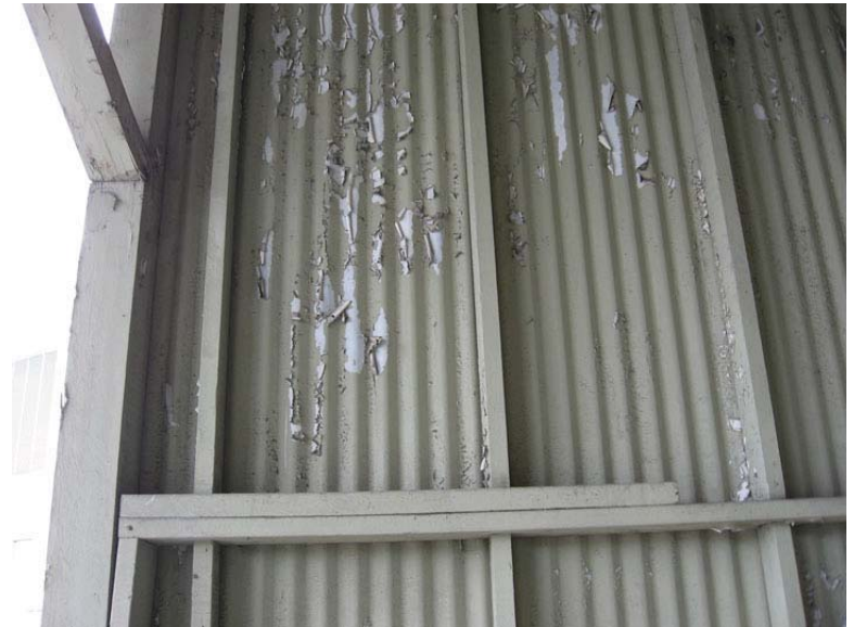
Photo 40. Degraded Paint on Building 7-027-1 (View 2)
