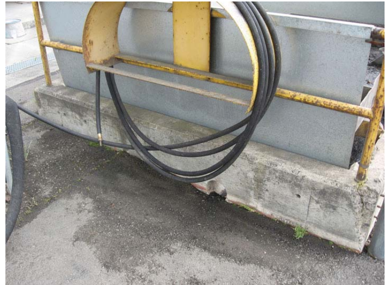
Photo 12. Detail of Drain from the Sweeper Decant Station (note apparent water staining on ground surface)
