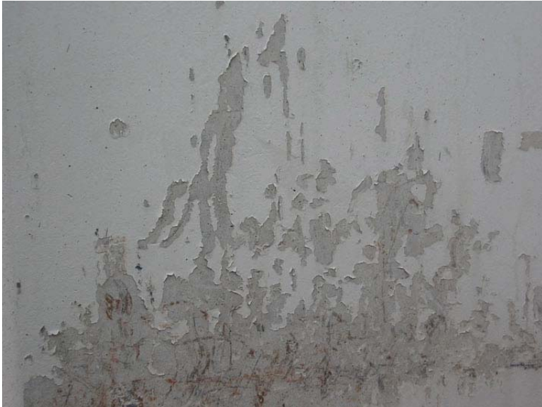
Photo 37. Degraded Paint on Building 3-315 (View 2)
