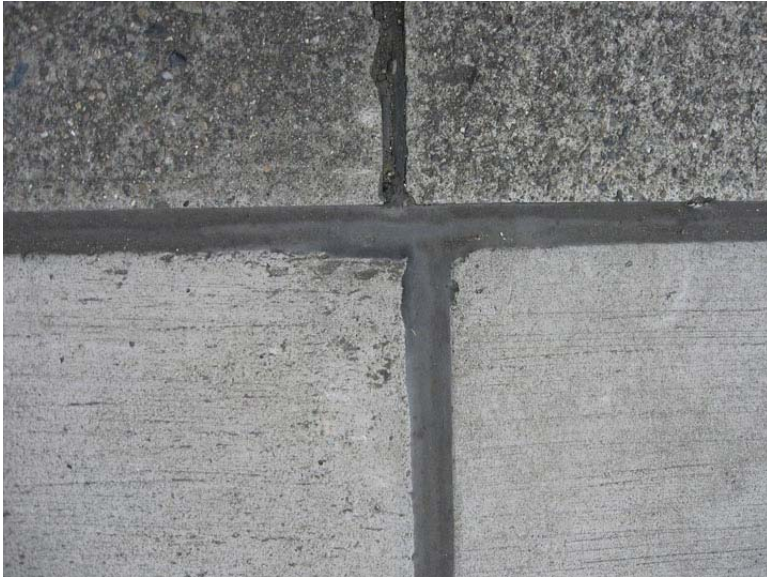
Photo 1. Comparison of New Caulk and Old Caulk between Buildings 3-369 and 3-380
