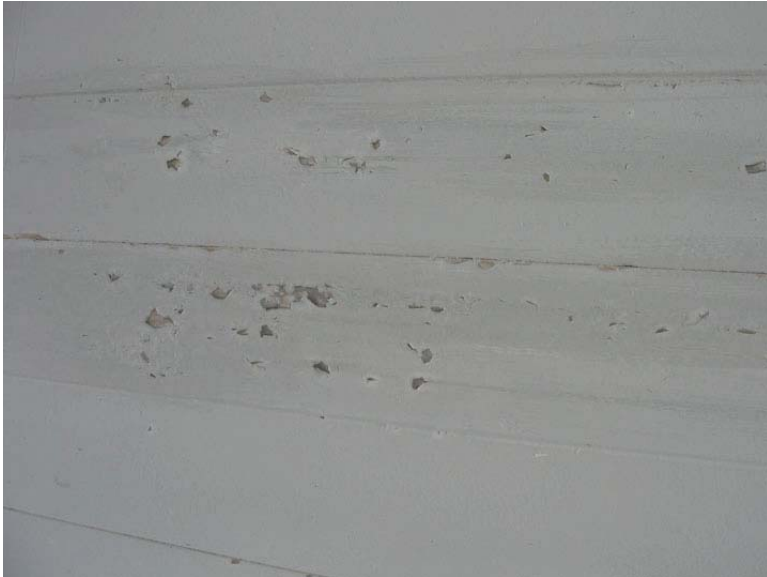
Photo 45. Degraded Paint on Building 3-374 - Detail
