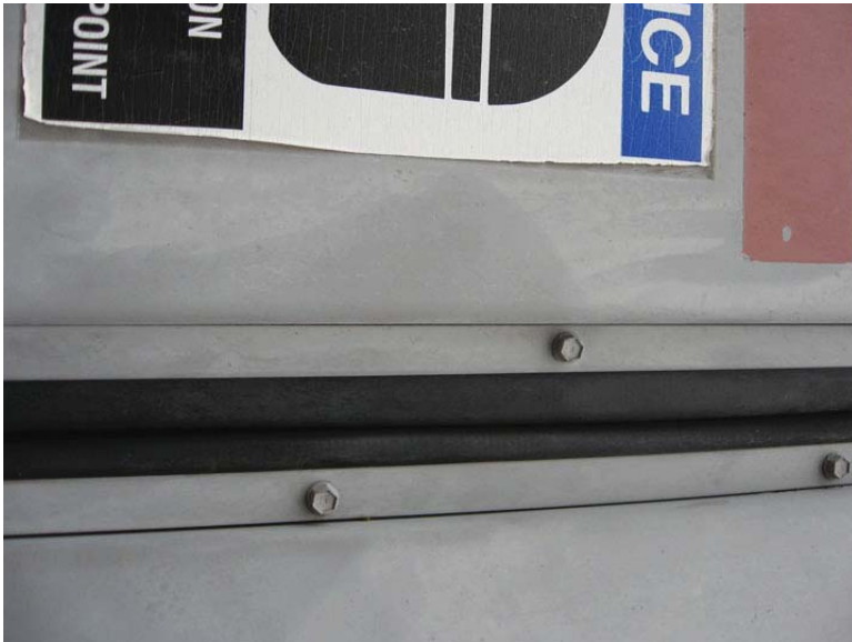
Photo 67. Rubber Gaskets on Doors at Building 3-315 - Detail
