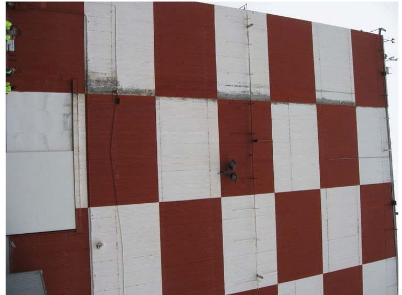
Photo 32. Degraded Paint on Building 3-390
