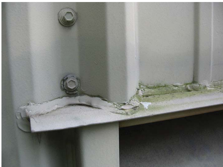
Photo 23. Vent Caulk at Building 3-323
