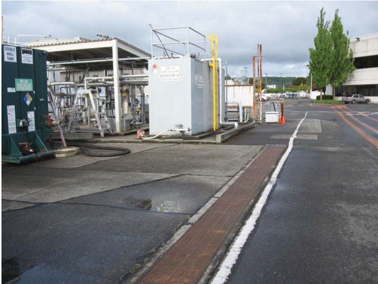
Photo 13. Sweeper Decant Station - Settling Tank
