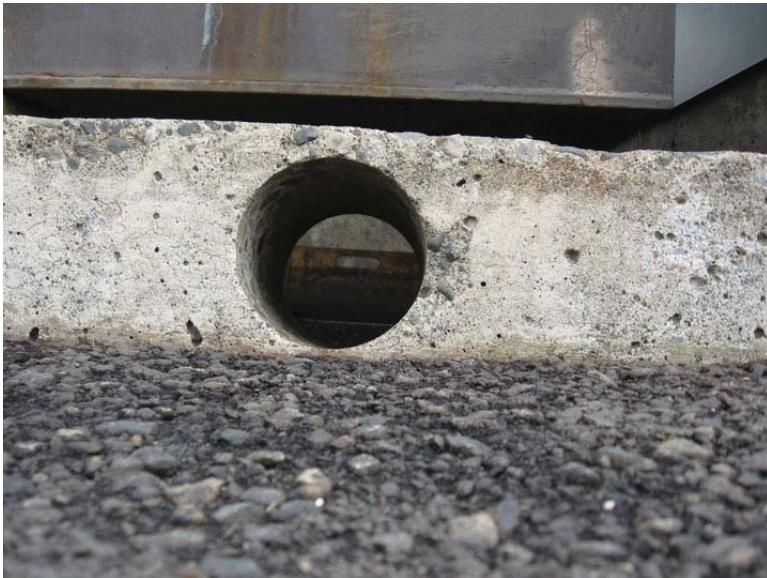
Photo 11. Detail of Drain from the Sweeper Decant Station
