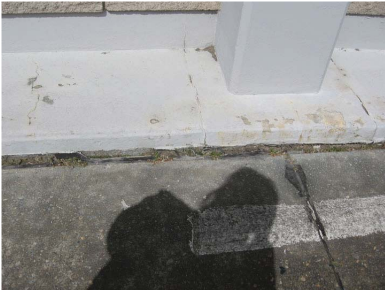
Photo 7. Degraded Caulk between Parking Lot and Sidewalk at Building 3-818
