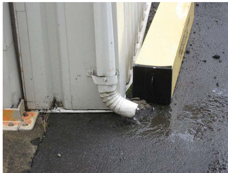
Photo 52. Roof Drain on Building 3-302 - Detail
