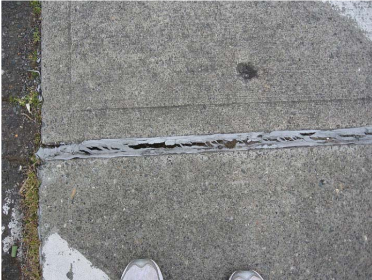
Photo 5. Degraded Caulk on the Sidewalk between Buildings 3-365 & 3-380
