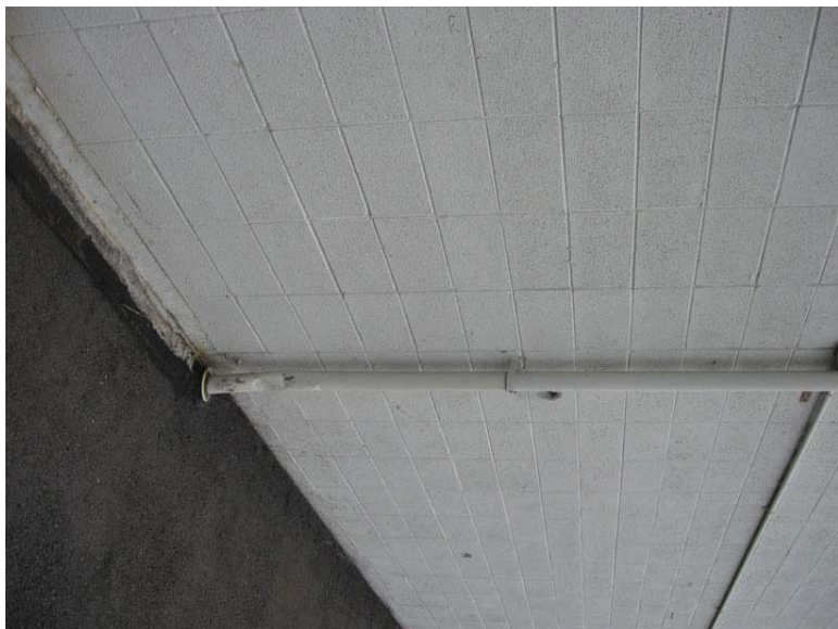
Photo 57. Roof Drain on Building 3-326 (note drain is connected to SD system)
