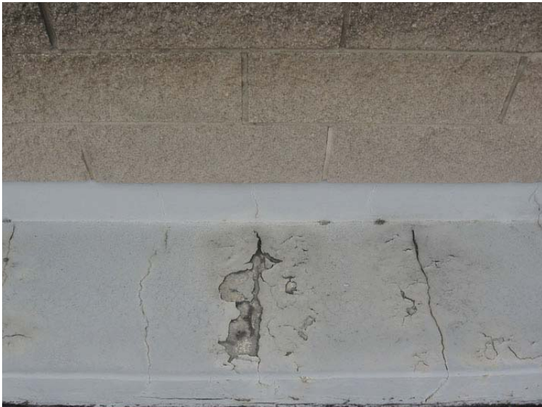
Photo 47. Degraded Paint on Building 3-818 - Detail (note that caulk or mortar between concrete blocks is also degraded)
