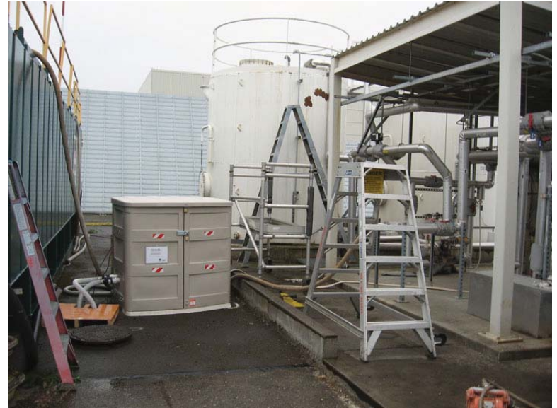
Photo 14. Sweeper Decant Station & Treatment System (note concrete berm around treatment system is not continuous)
