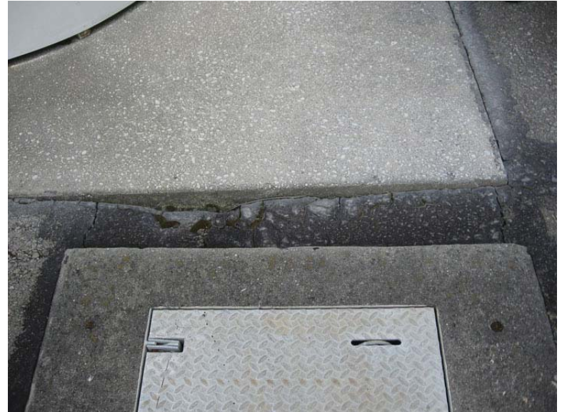
Photo 6. "Hot Patch" Asphalt used as CJM at Building 3-368
