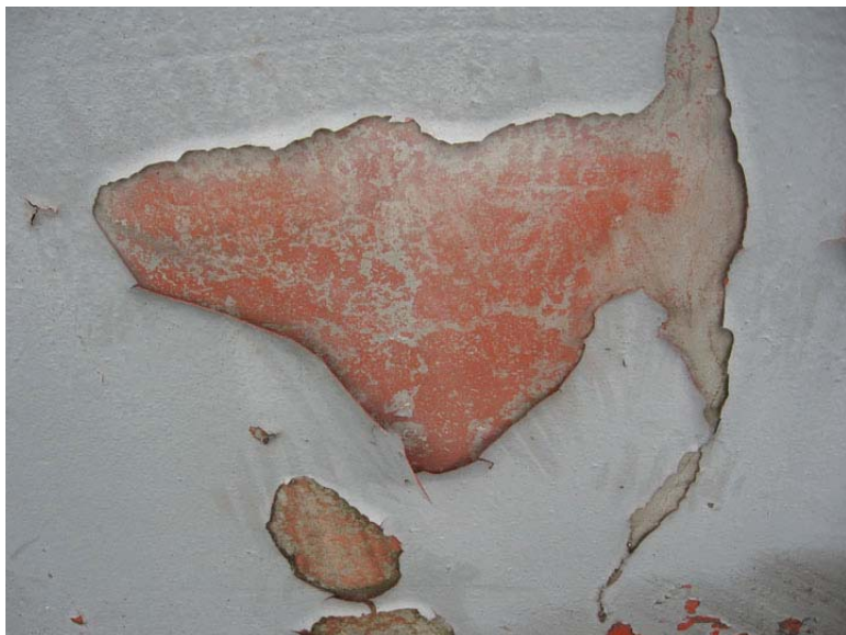
Photo 33. Degraded Paint on Building 3-390 - Detail 1
