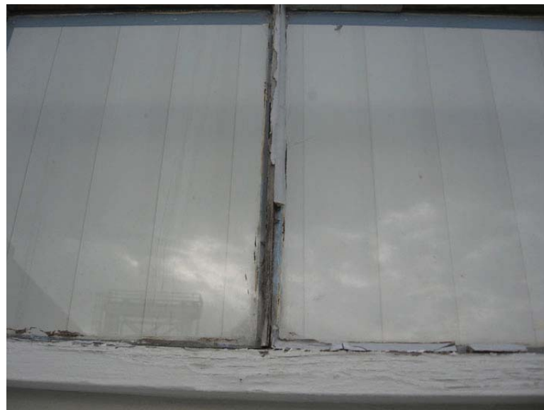
Photo 22. Degraded Window Caulk and Glazing at Building 3-365
