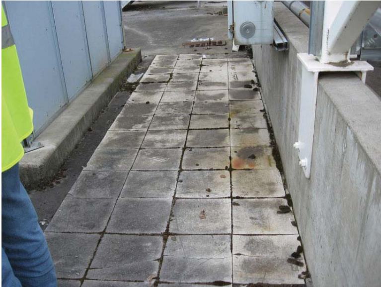
Photo 65. Interior Floor Tiles Used Outdoors near Building 3-310
