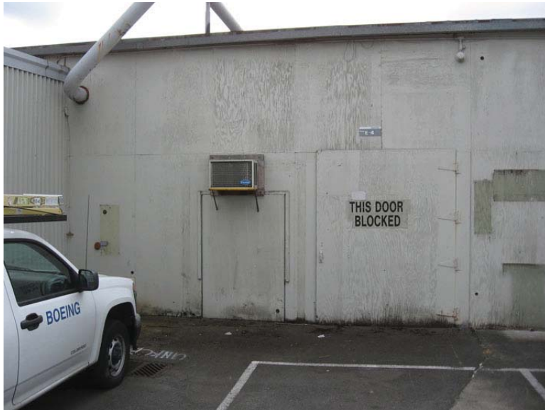
Photo 69. Plywood Siding on Building 3-326
