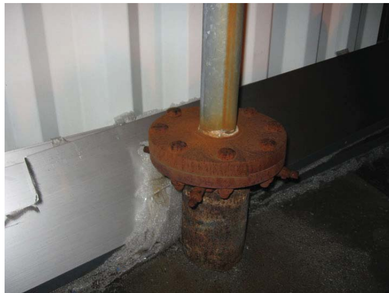
Photo 82. Flange at Building 3-356 (note caulk around connection between the pipe and flange)
