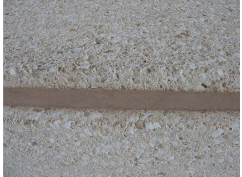
Photo 30. Concrete Joint Material (Caulk) on Building 3-800
