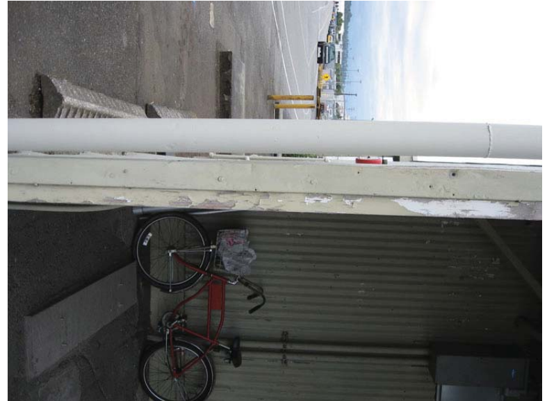
Photo 38. Degraded Paint on Building 7-027-1 (View 1)
