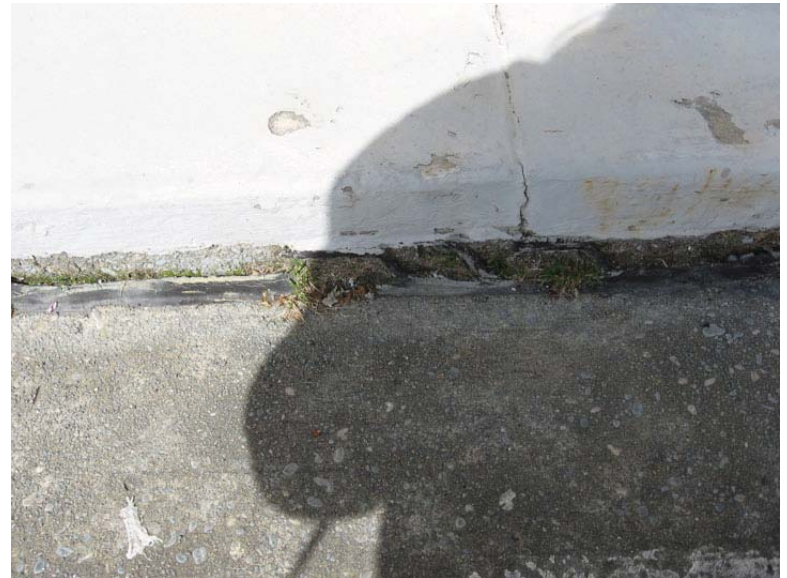
Photo 8. Degraded Caulk between Parking Lot and Sidewalk at Building 3-818 - Detail
