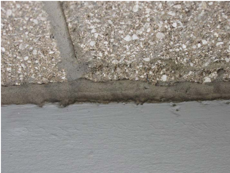
Photo 31. Concrete Joint Material (Caulk) on Building 3-818
