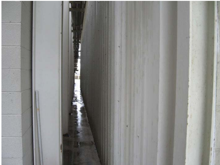
Photo 71. Concrete Block Construction and Metal Siding on Buildings 3-323 and 3-334
