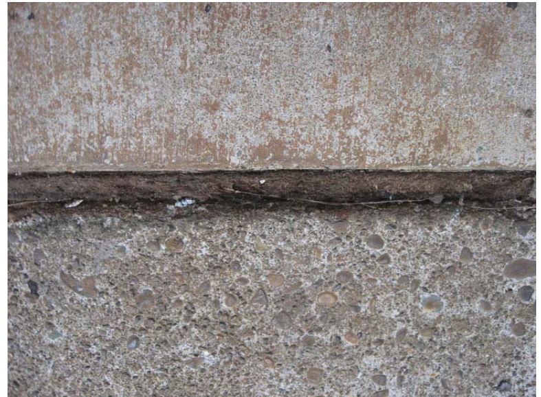
Photo 4. Fibrous CJM between Buildings 3-334 and 3-332
