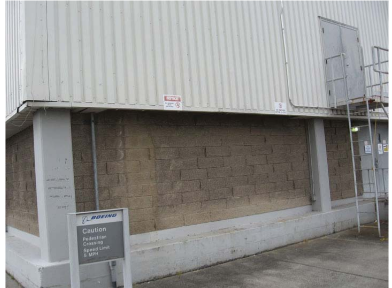
Photo 46. Degraded Paint on Building 3-818
