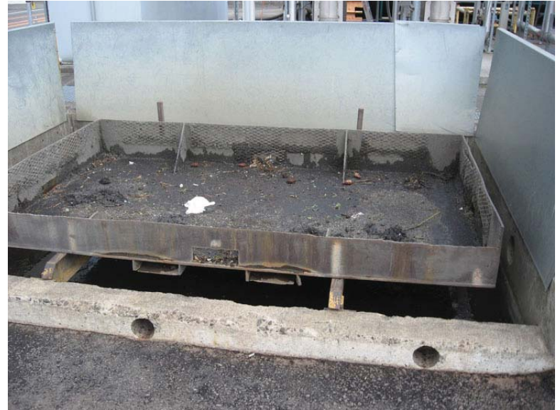
Photo 10. Sweeper Decant Station (June 17, 2010)
