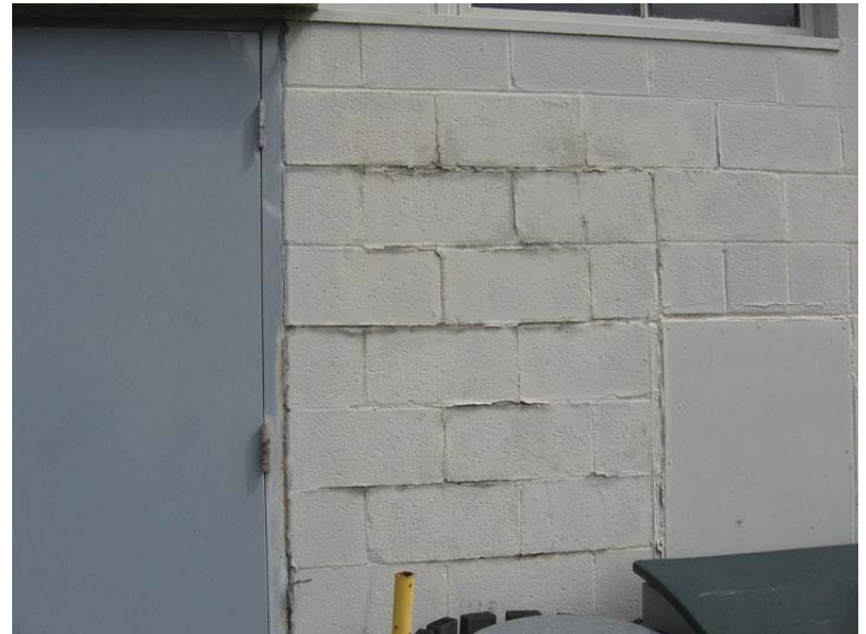
Photo 48. Degraded Paint on Building 3-822 (note that door caulk is peeling away from the door jamb)
