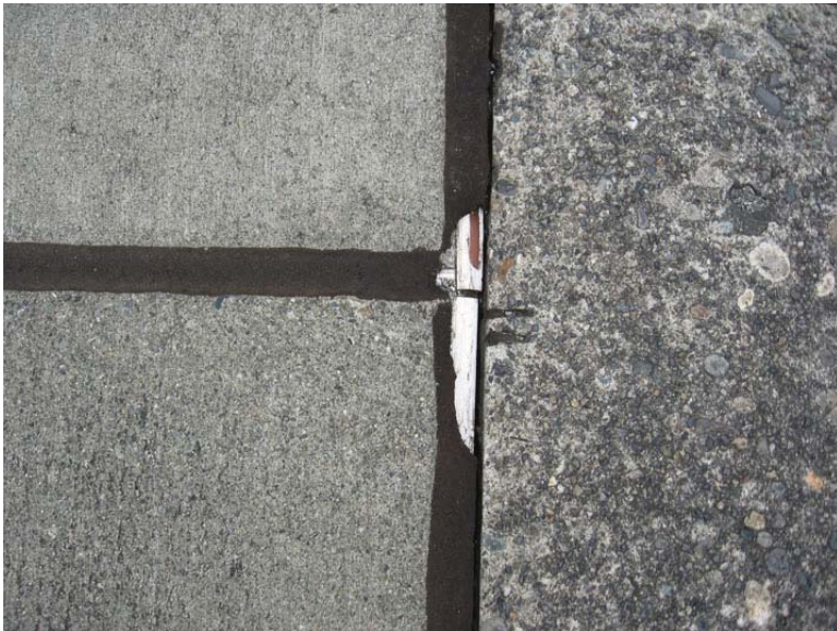
Photo 3. Degraded Caulk with Plastic Backing on the Flight Line
