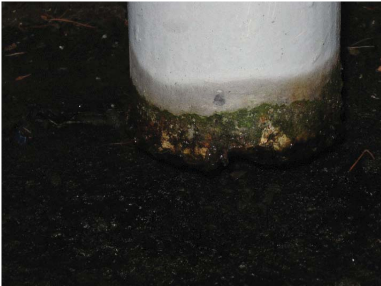
Photo 63. Roof Drain on Building 3-397 - Detail (note connection to SD system is broken)
