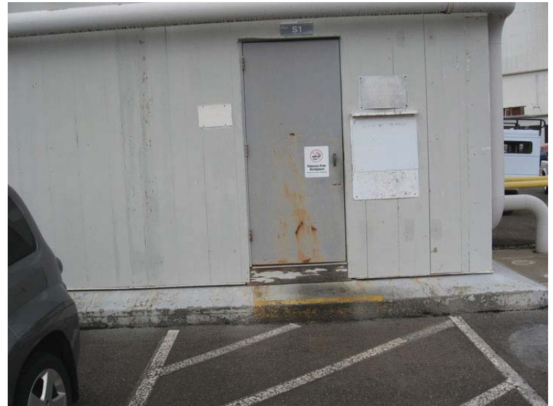
Photo 44. Degraded Paint on Building 3-374
