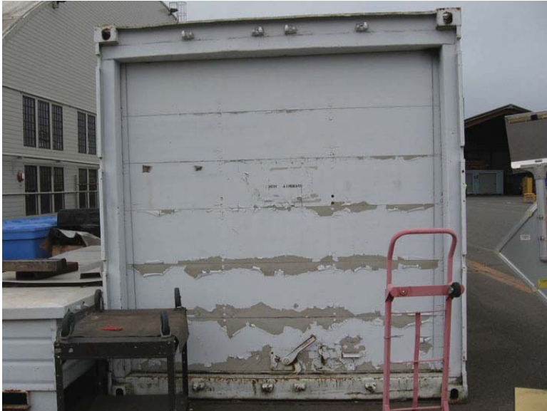
Photo 41. Degraded Paint on Container near Building 3-350
