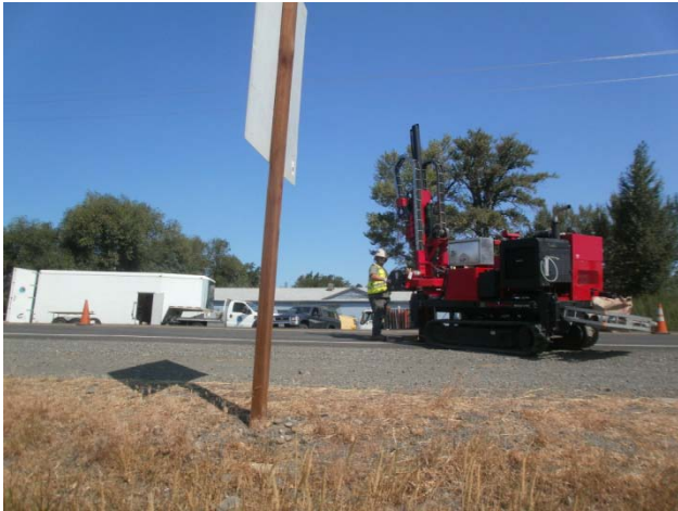
Advancing boring BH-17.
