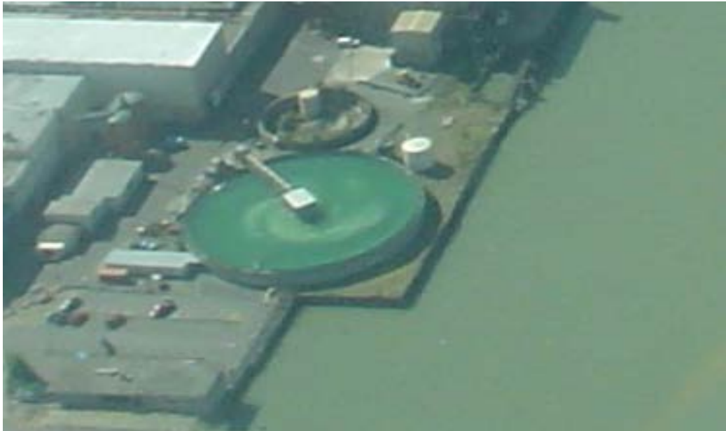
Plate 3 Aerial Photograph of Clarifier Tank and Creosote-timber Clarifier Bulkhead to be Removed, South Shoreline of Inner Waterway Area (facing south)
