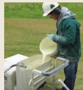
FIGURE 1: FILLING A PUMP WITH ORC ADVANCED SLURRY
