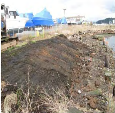
Photograph 3 Final grade before geotextile is laid down.
