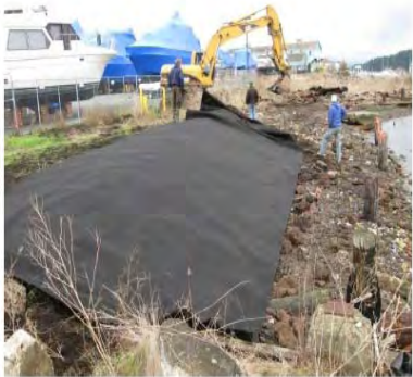
Photograph 4 Rolling out geotextile.
