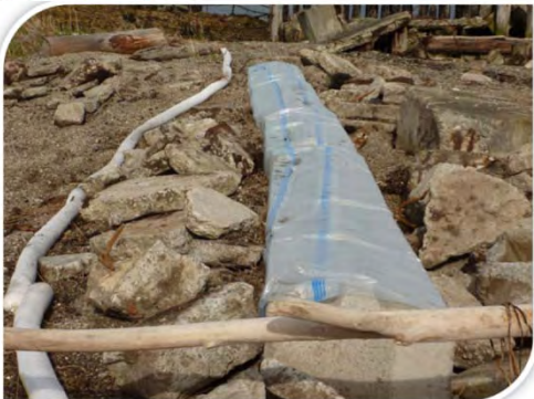
Photograph 4 Rolling out geotextile.
