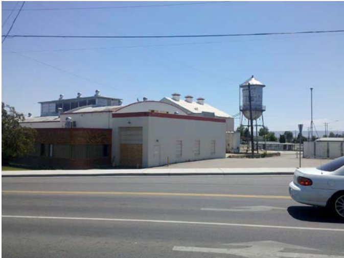
View of the Site from the North
