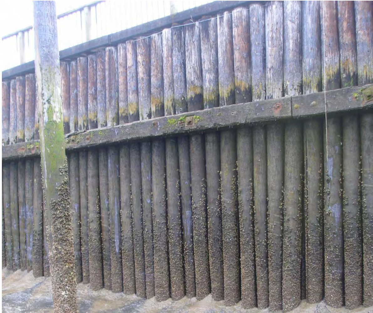
Photograph 2: Segment B Bulkhead Wall
