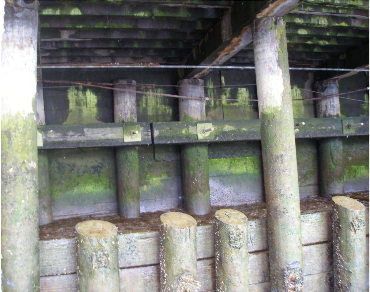
Photograph 1: Segment A Bulkhead Wall
