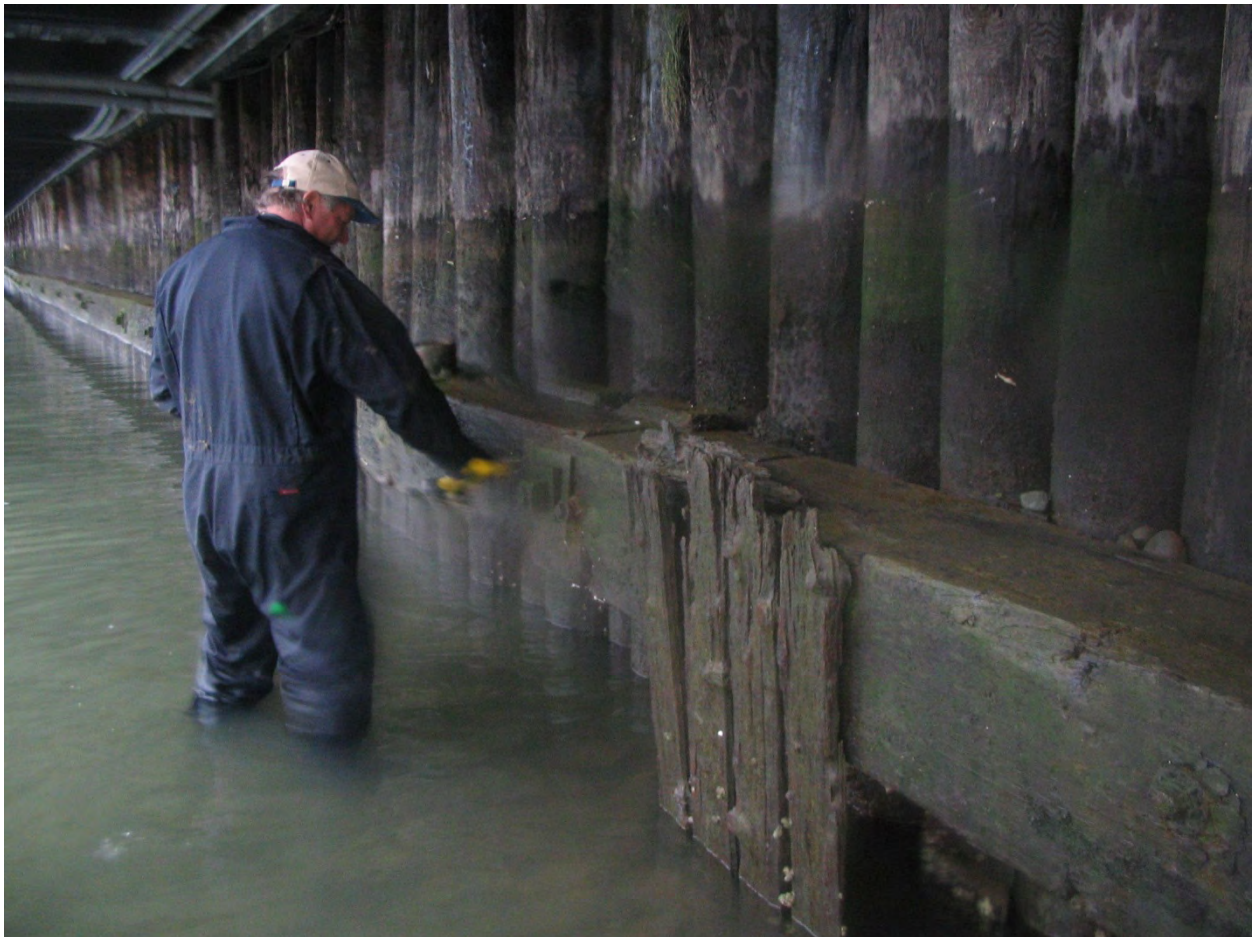
Photograph 3: Segment C Bulkhead Wall
