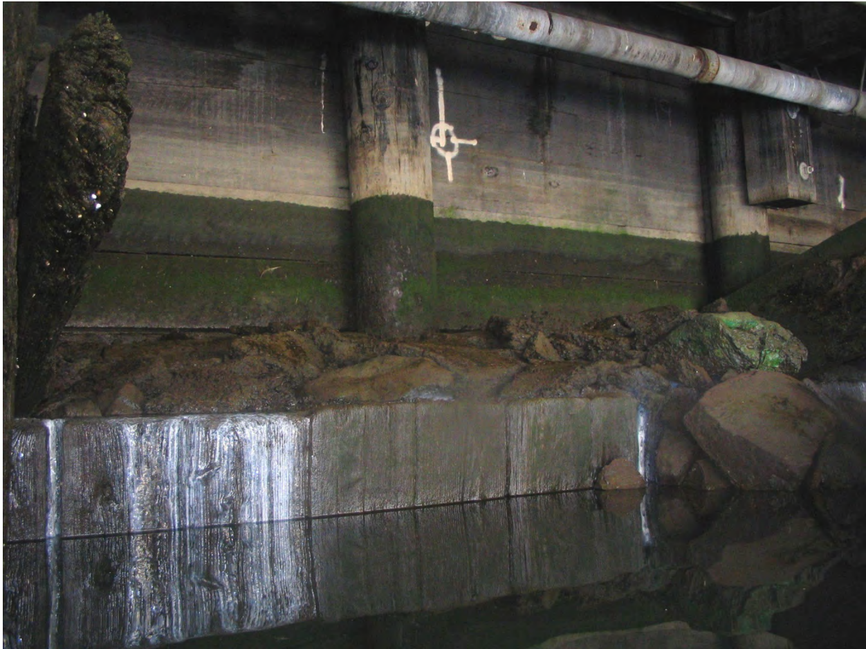
Photograph 4: Segment D Bulkhead Wall
