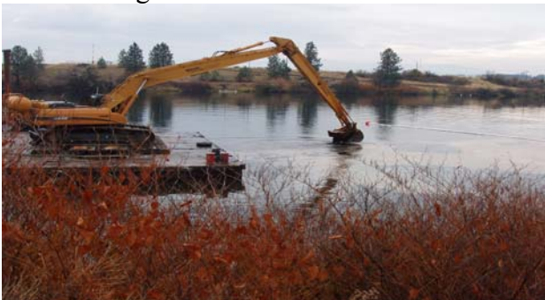
Placing the Cap at Upriver Dam
