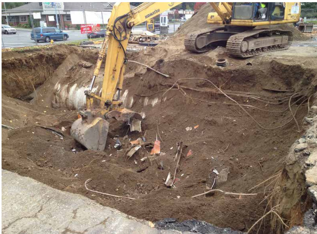
Removal of pieces of second 12,000-gallon single-wall fiberglass UST for disposal.
