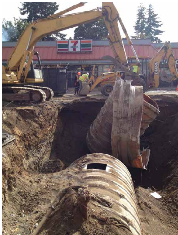
Removal of third 12,000-gallon single-wall fiberglass UST for disposal.
