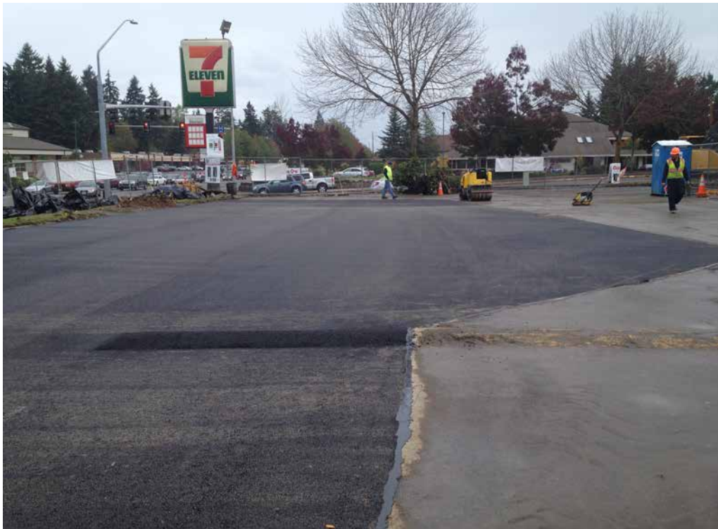
View of site at end of asphalt paving.
