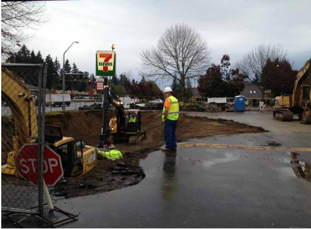
View of backfilling operation.
