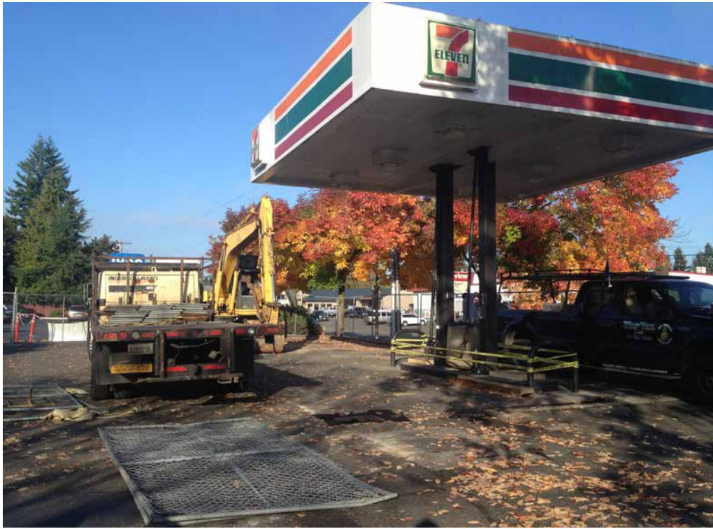
View of gasoline canopy prior to commencement of work.
