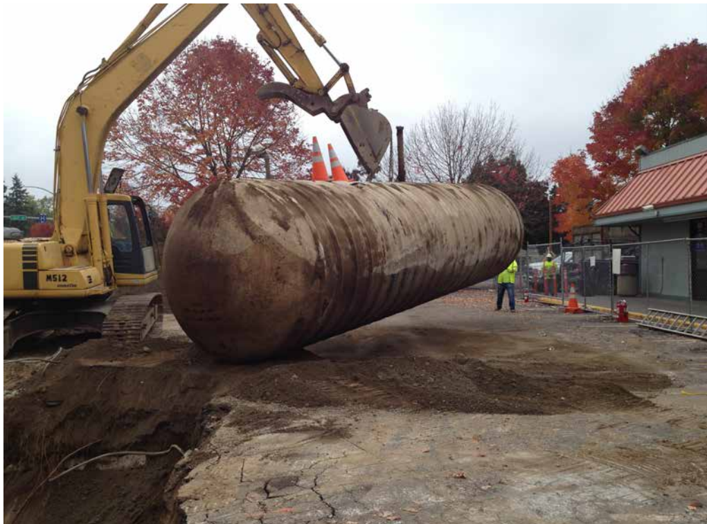
Removal of first 12,000-gallon single-wall fiberglass UST.
