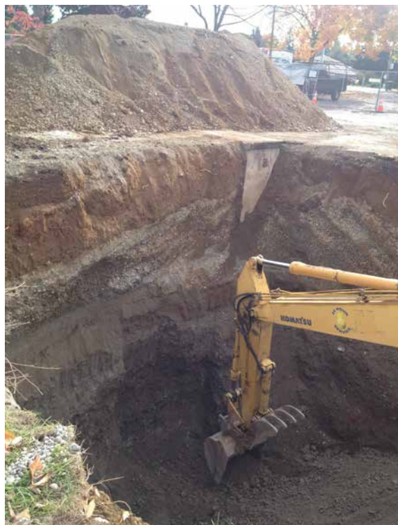
View of over excavation of dispenser area.
