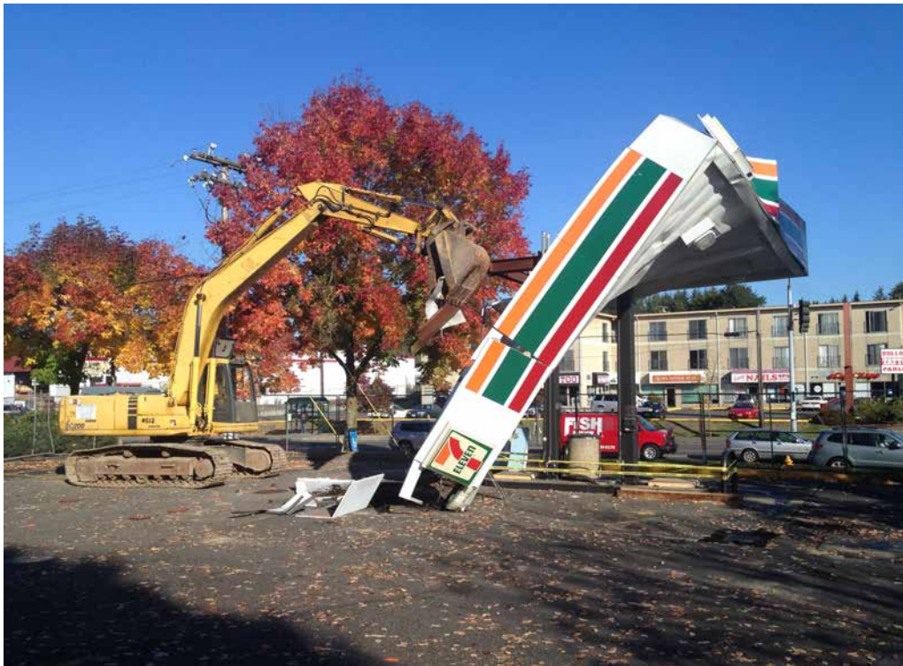
Removal of gasoline canopy.
