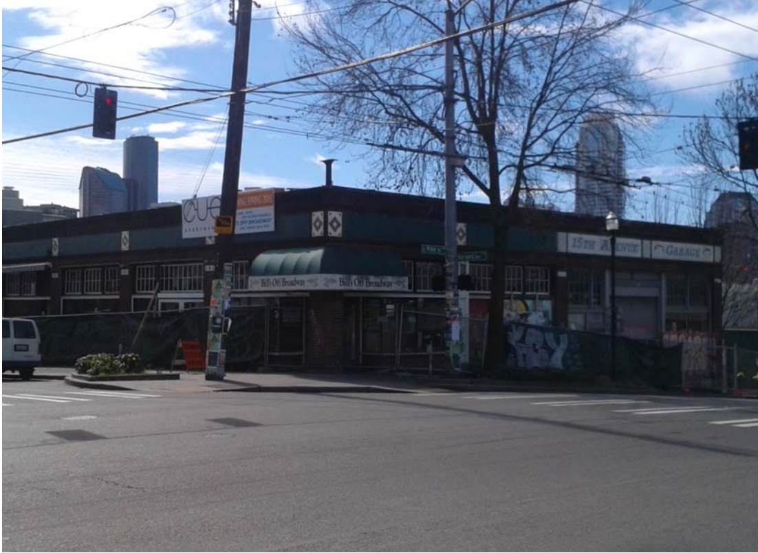
Photograph 1 – View of northeast corner of building, looking southwest. The entrances for the 15th Avenue Garage and Bill's Off Broadway can be observed behind the construction fencing.
