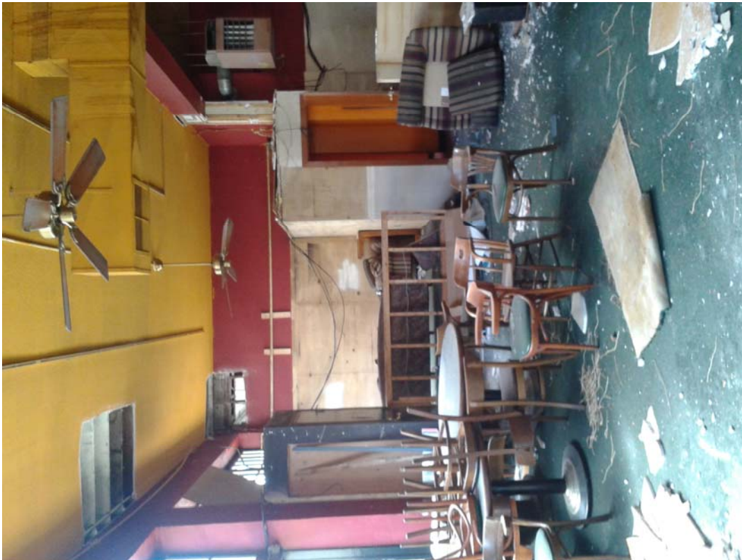
Photograph 2 – Interior of Bill's Off Broadway restaurant. Note hole cut in ceiling for HBM testing and natural gas heater hanging from ceiling to the right of the photograph. (← up)
