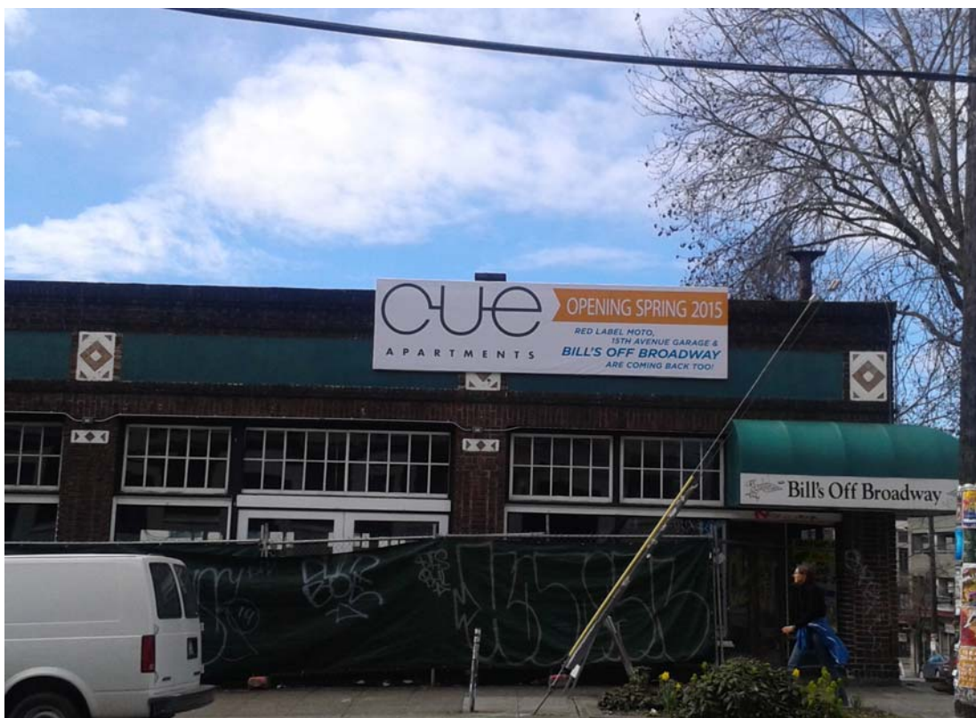
Photograph 10 – View of east wall of building, looking west.
