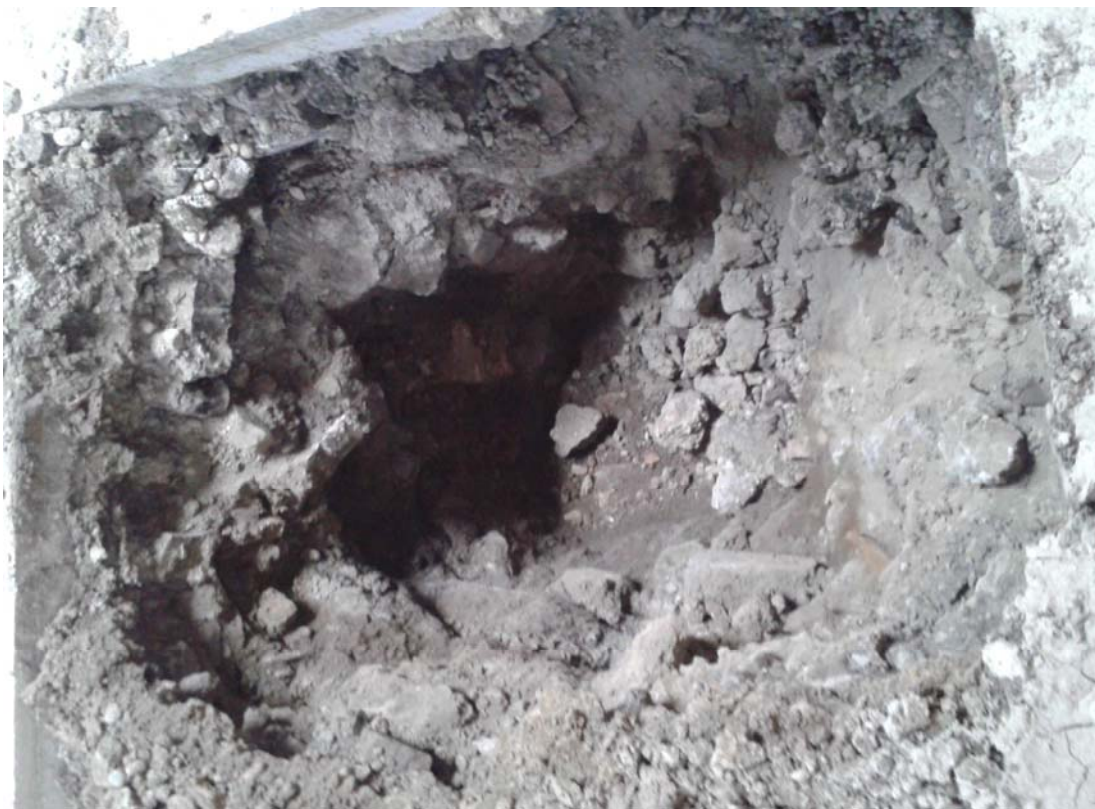
Photograph 5 – Test pit at south end of 15th Avenue Garage, showing rubble below concrete floor to a depth of approximately 8 feet. (← up)
