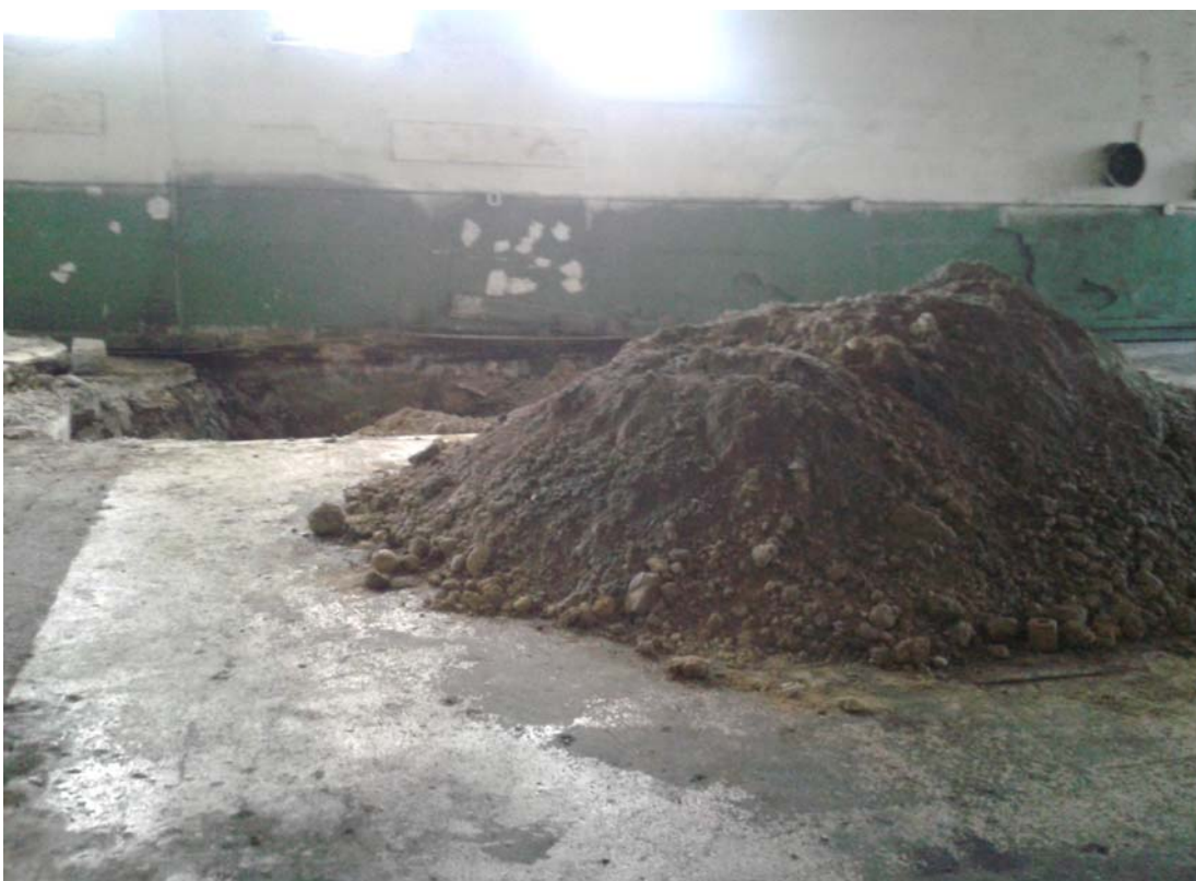
Photograph 6 – Interior of 15th Avenue Garage, showing second test pit along west wall. Excavated material is predominantly soil.
