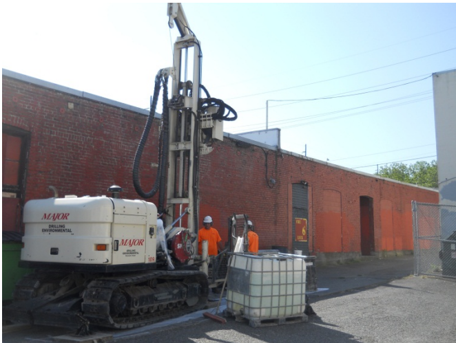
Photograph 17. Installing a monitoring well in the alley between the 800 Roy Street and 701 9 th Avenue North parcels.
