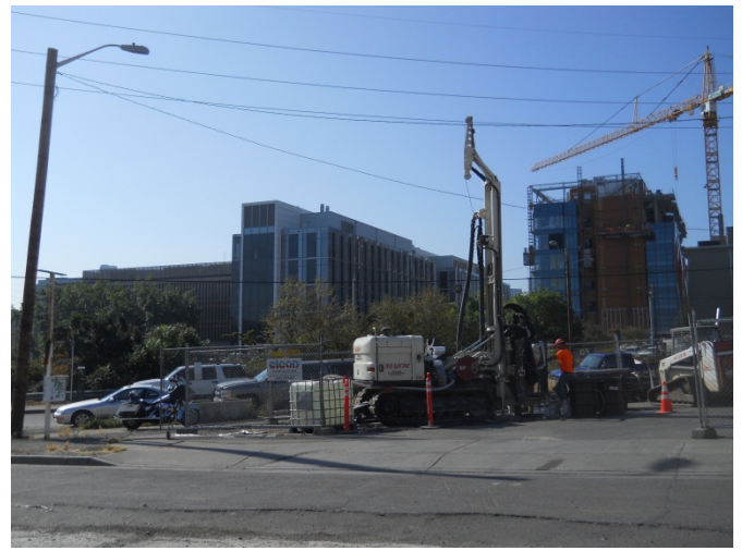
Photograph 14. Installation of monitoring well MW106 on the south-adjoining property.
