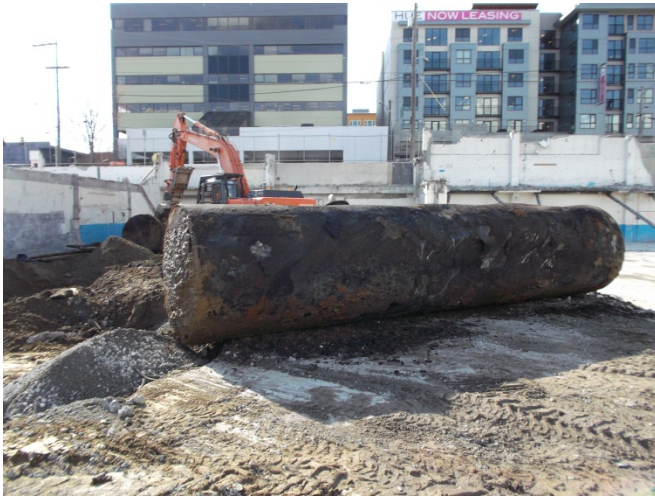
Photograph 15. View facing west of underground storage Tank 2 during March 2013 decommissioning activities.
