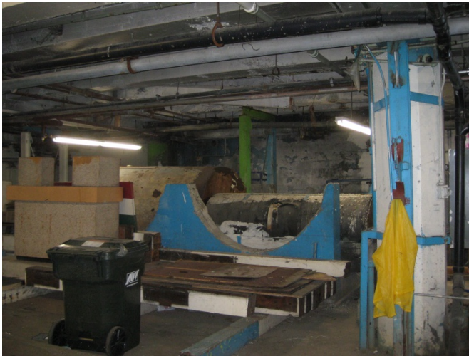
Photograph 9. Aboveground storage tanks and saddles in the eastern portion of Building A basement.
