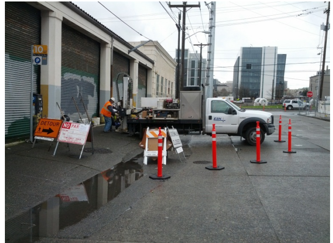
Photograph 16. Installation of soil-gas sampling point to the east-adjoining property, 800 Roy Street parcel.
