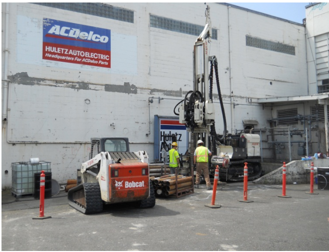
Photograph 13. Installation of monitoring well MW101 on the Property, facing southwest.
