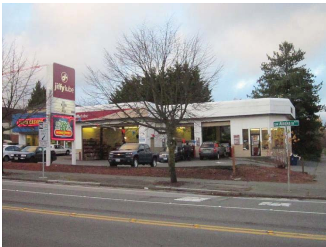
Photograph 5. Northwest-adjacent Jiffy Lube.
