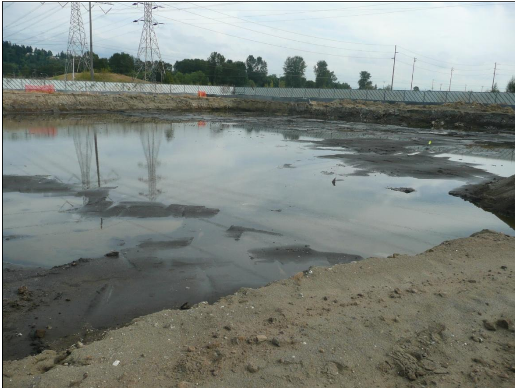
5. Looking southeast across the completed Closed Landfill excavation.
