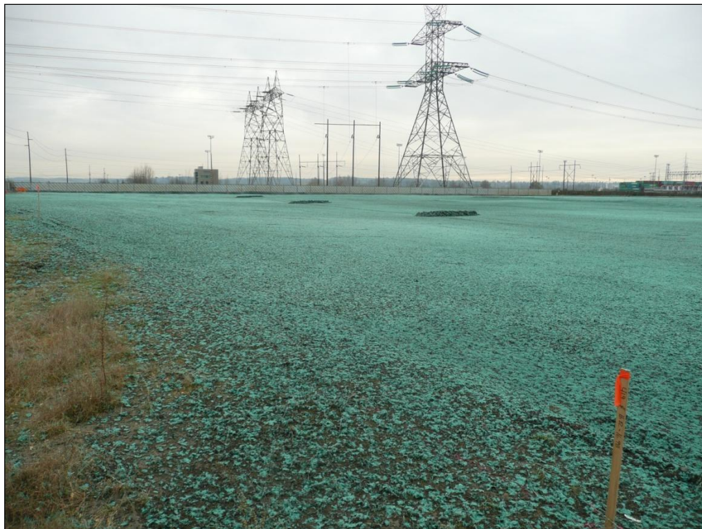
10. Looking southwest across the Closed Landfill area after completion of excavation backfilling and hydroseeding.
