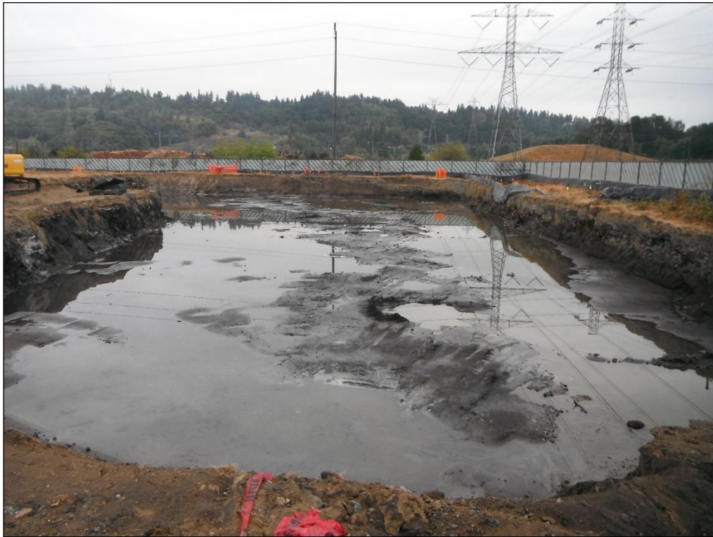
2. Looking east across the Closed Landfill area excavation (in progress).
