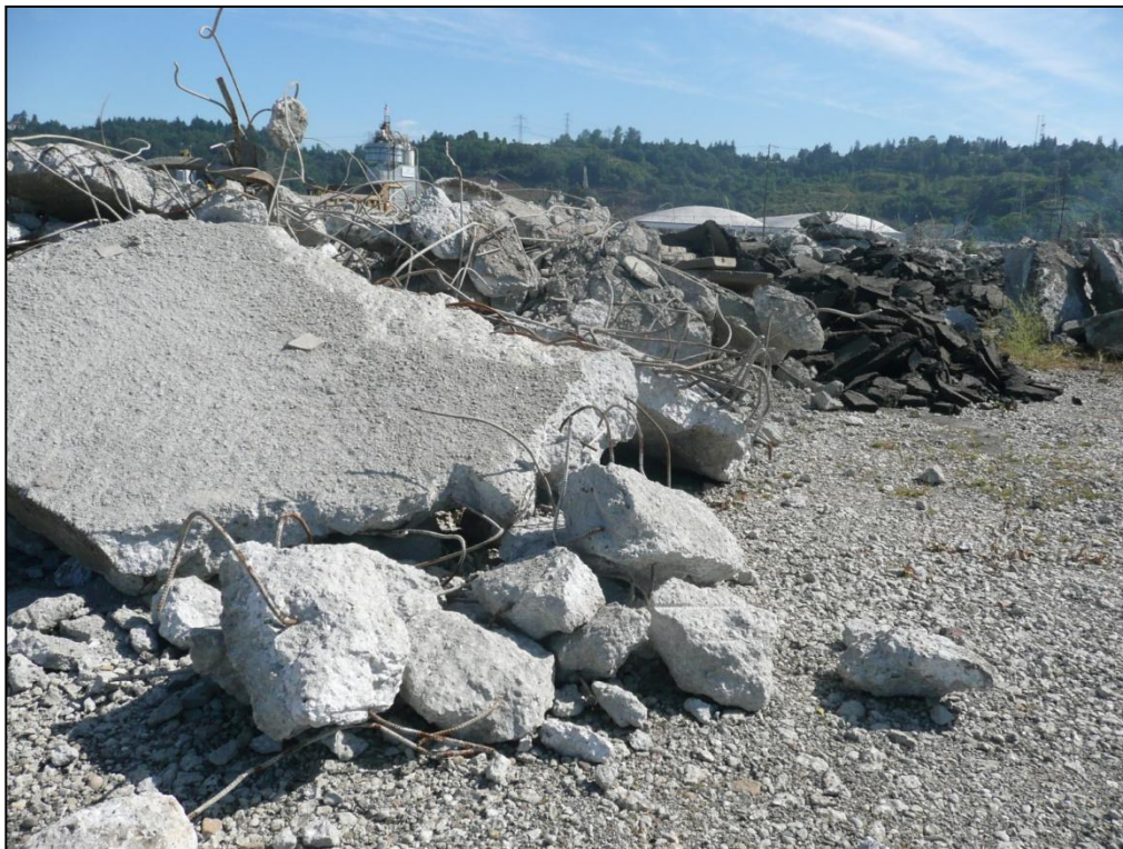
4. Stockpiled concrete and asphalt demolition debris prior to rubblization.
