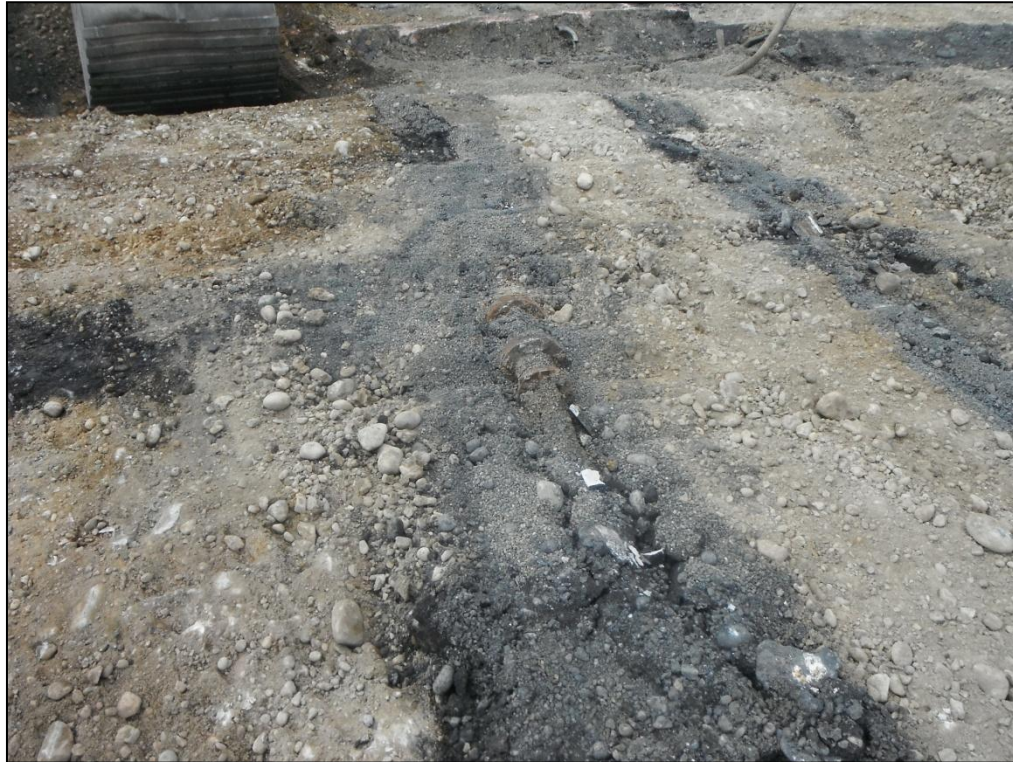
9. Close-up view of SPL material used as utility trench backfill.
