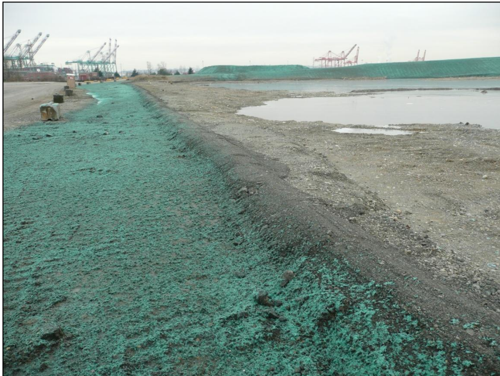
16. Looking southwest at the stormwater diversion berm constructed along the south side of the SPL Area excavation where water is ponded.
