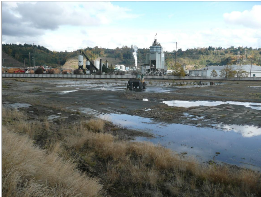
1. Looking northeast across the SPL Area prior to removal of surficial concrete slabs and asphalt pavement.
