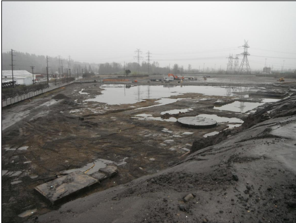
15. Looking southeast across the completed SPL Area excavation from the dredged soil stockpile, with water ponded in a significant portion of the excavation.
