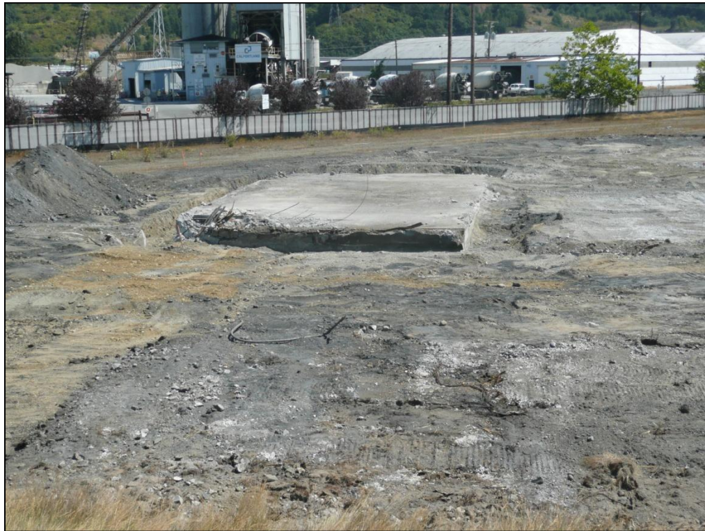
7. Looking east across the pot dumping slab in the former SPL management facility.
