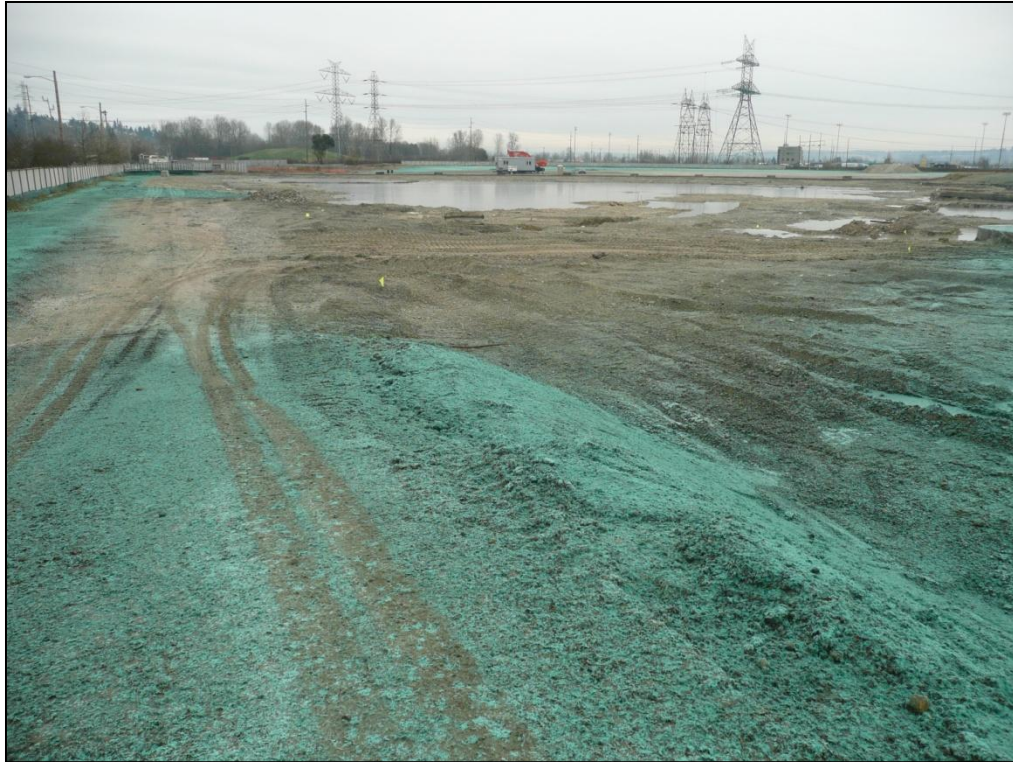
17. Looking southeast across the completed SPL Area excavation from the northern end of the dredged soil stockpile.
