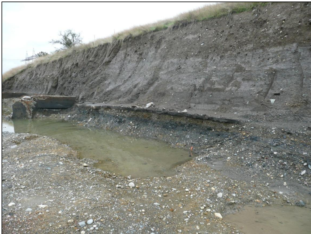
12. Looking southwest at a layer of SPL material extending under the dredged soil stockpile.
