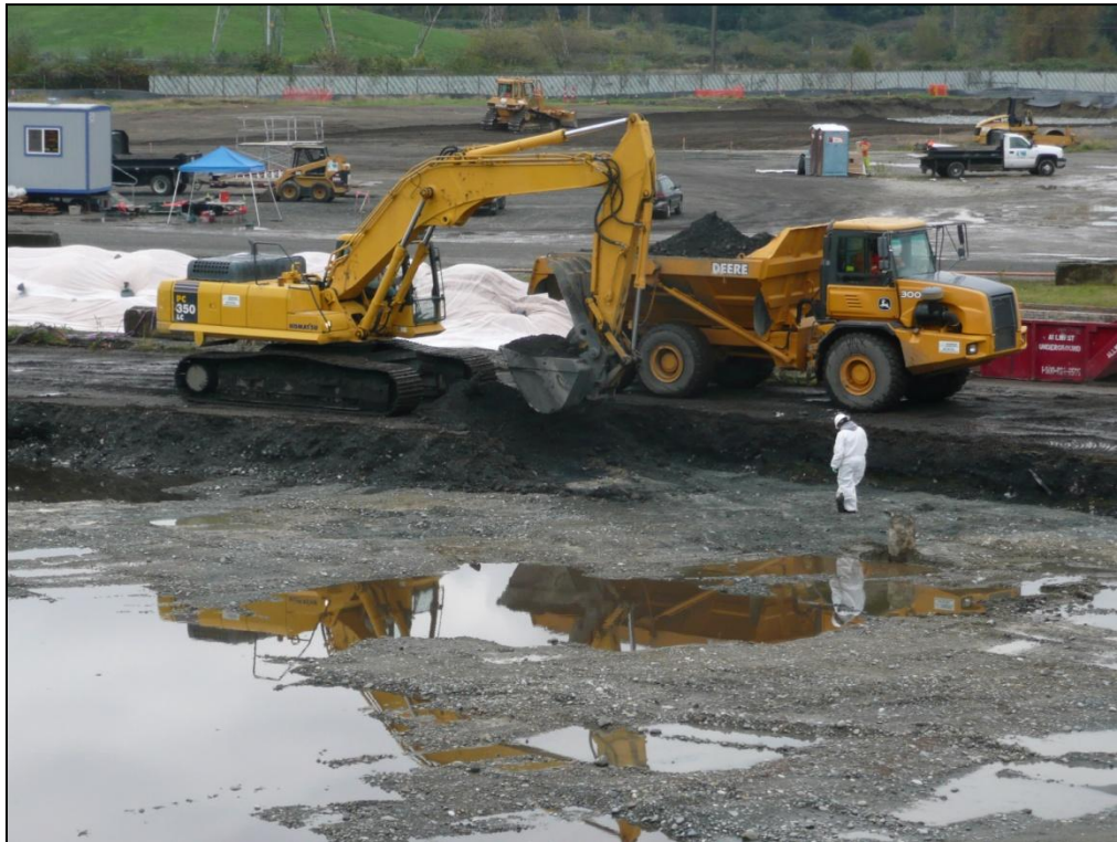
11. Looking southeast across the southern portion of the SPL Area during removal of SPL material.
