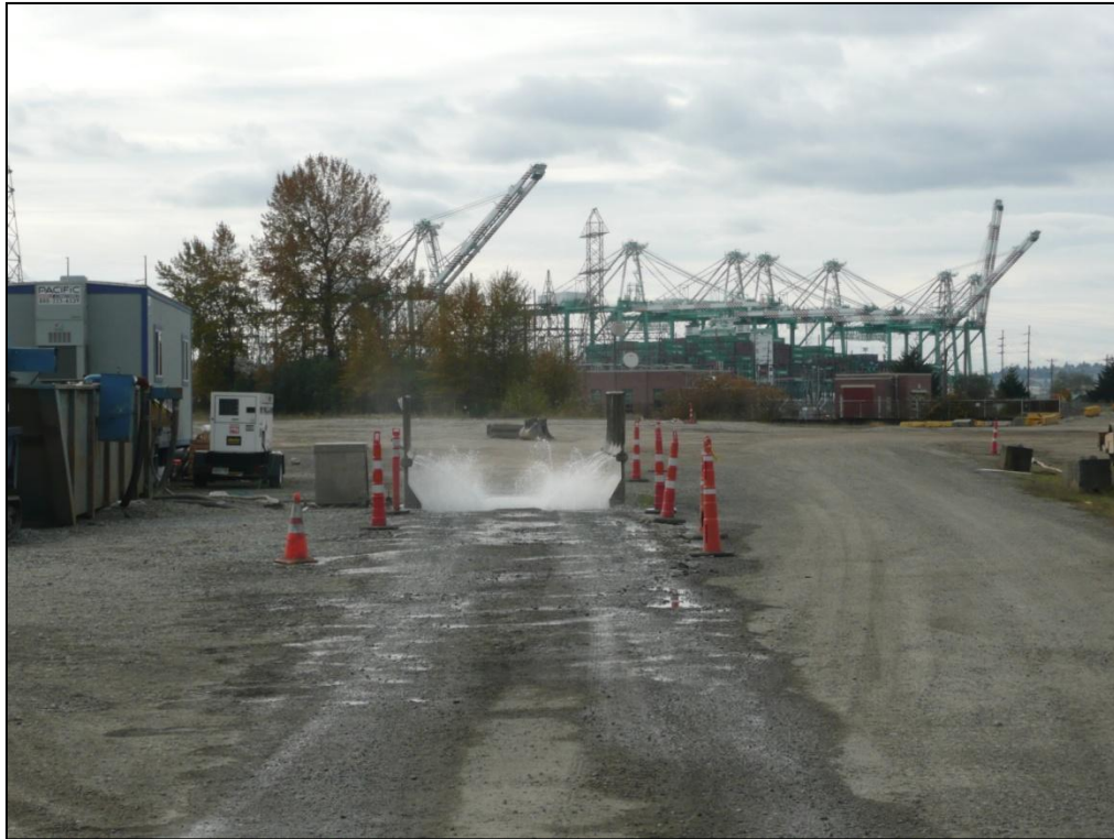
5. Looking southwest toward the automated wheel wash facility located adjacent to the site access road.
