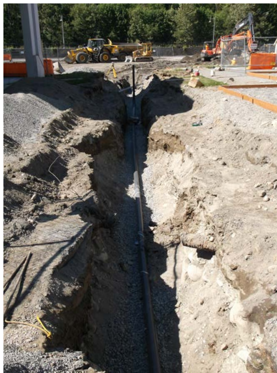
Photograph 14: Side sewer installation, looking north.
