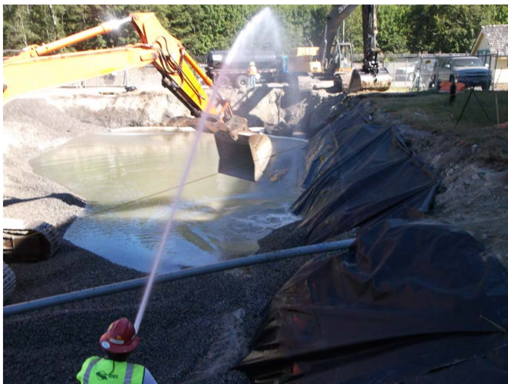
Photograph 10: Liner installation and backfilling, looking north from grid location F14.
