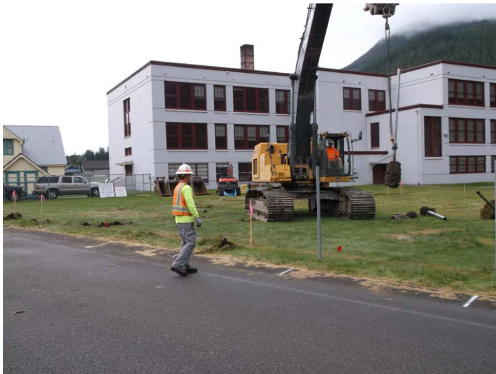
Photograph 1: Site preparation activities, looking southeast from West River Drive.
