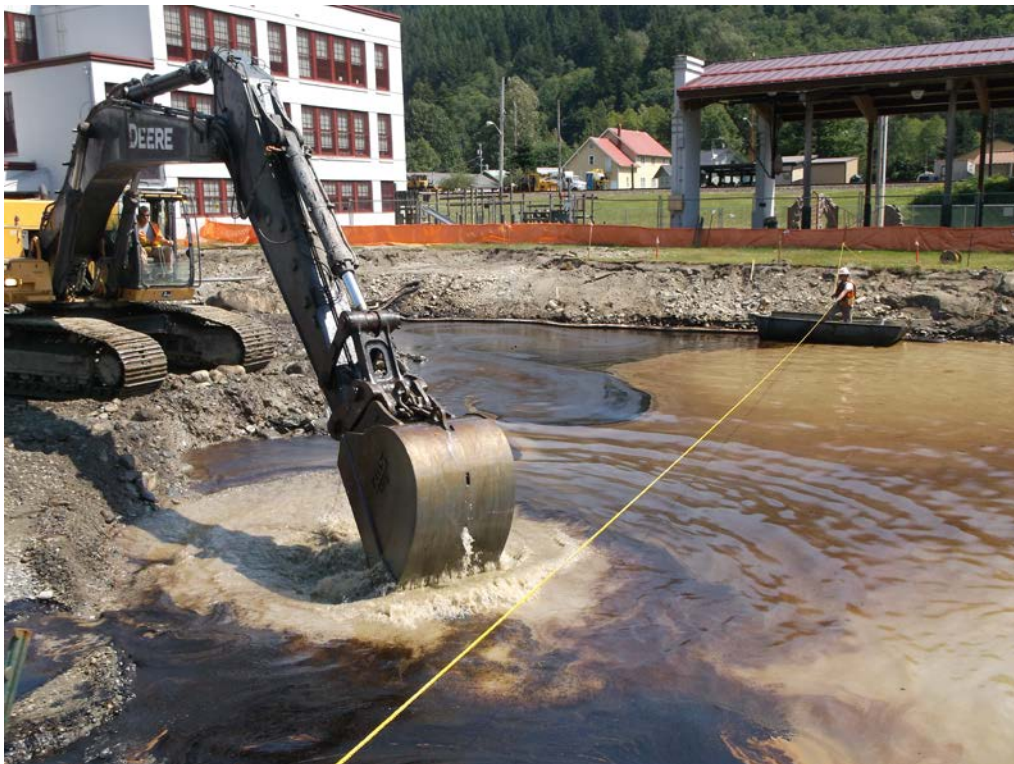
Photograph 3: Excavating below the vertical delineation limit (VDL).
