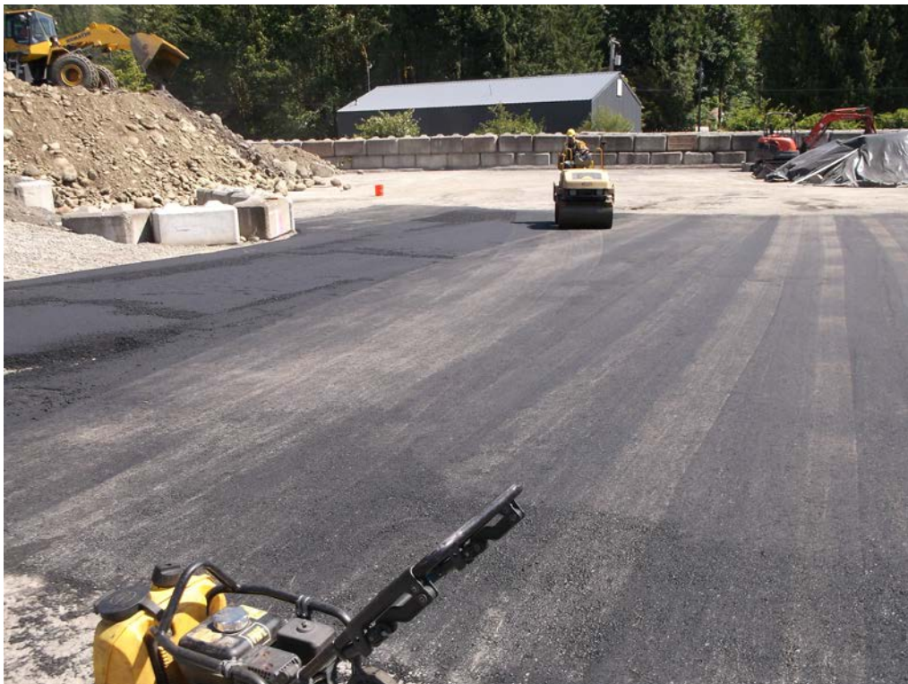
Photograph 11: Paving for soil-handling facility expansion, looking south.
