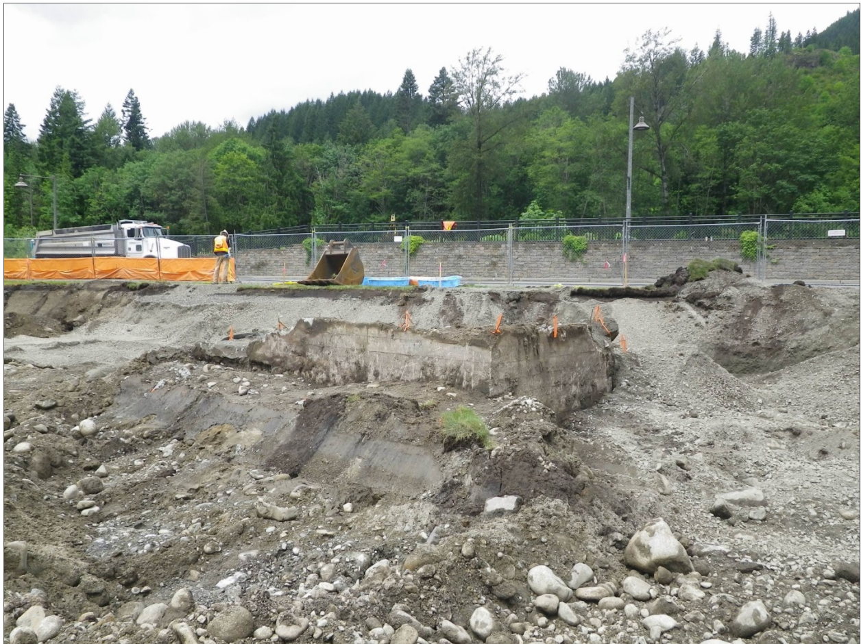
Figure 5-5. Overview photograph of cleared foundation remnants (view to northwest).
