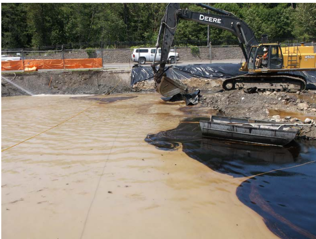
Photograph 4: Excavating below the VDL, removing liner installed in 2006.
