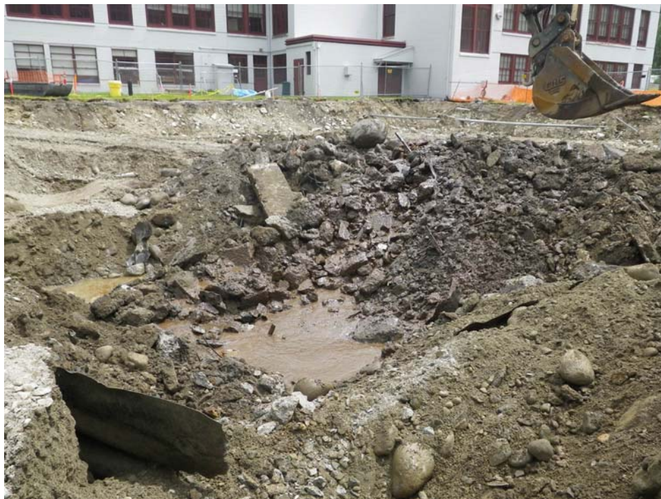
Photograph 8. Overview of water table, containing contaminated materials, beneath foundation (view to southeast).
