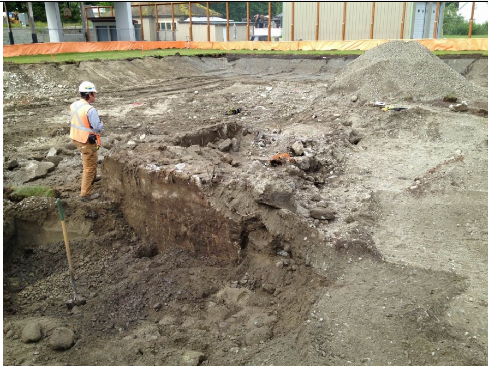
Photograph 7. Overview looking southwest of the east wall of the foundation.
