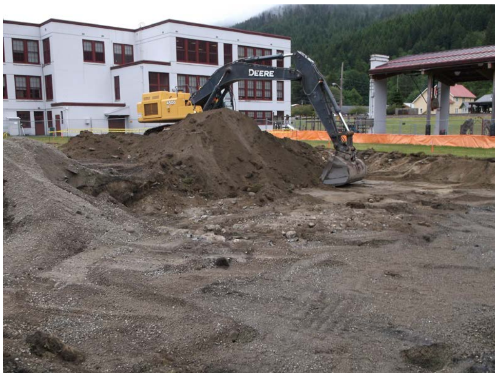
Photograph 2: Overburden removal, looking southeast from grid location C8.
