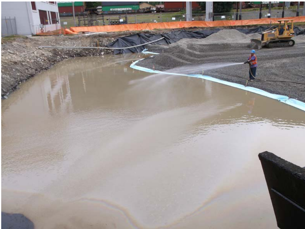
Photograph 5: Oil recovery, looking south from grid location B12.
