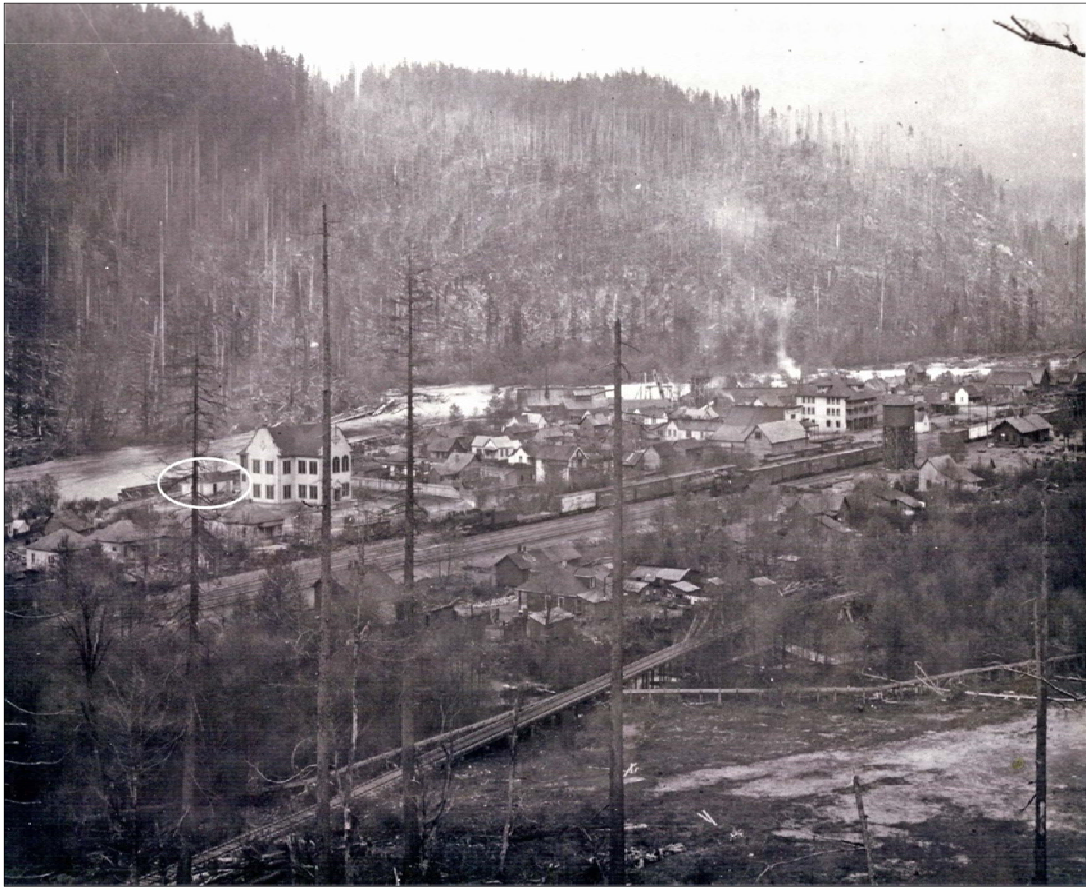
Figure 3-1. Overview photograph of the Town of Skykomish, view to the northeast, dating to ca. 1902 to 1914. A small coal shed to rear of school is circled. Photograph courtesy of the Skykomish Historical Society.
