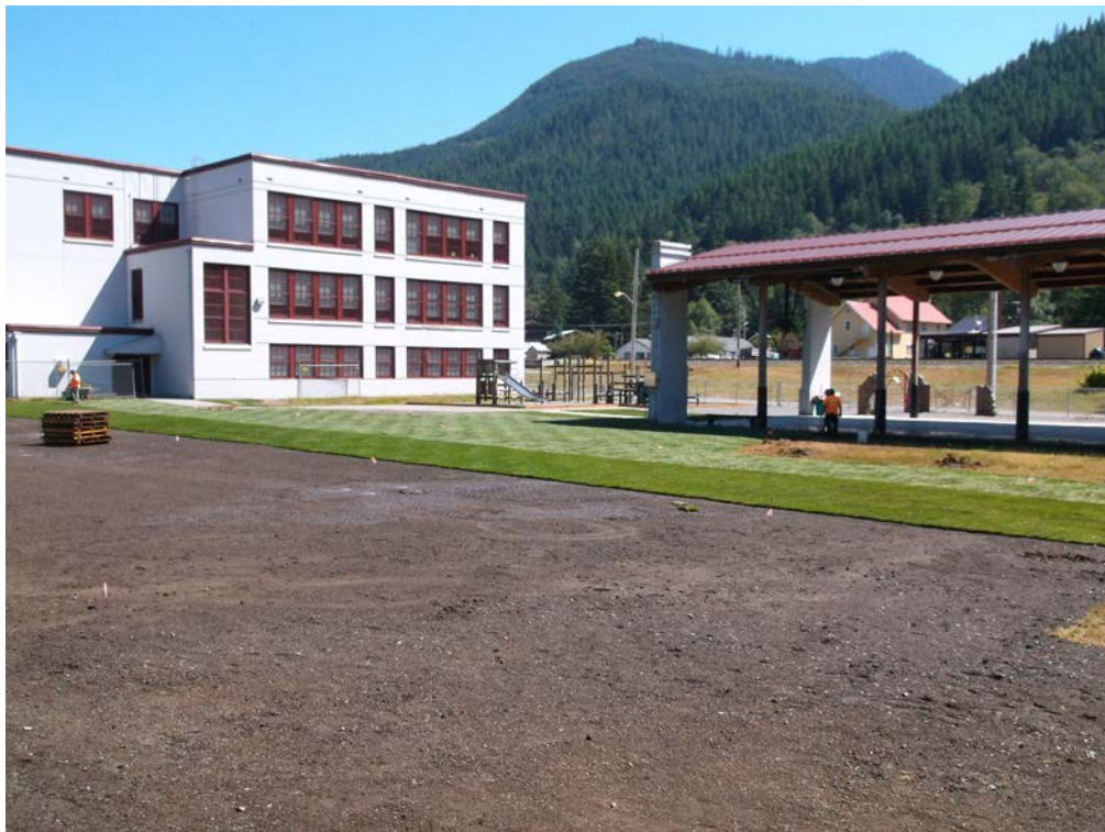
Photograph 17: Restoration activities, looking southeast.
