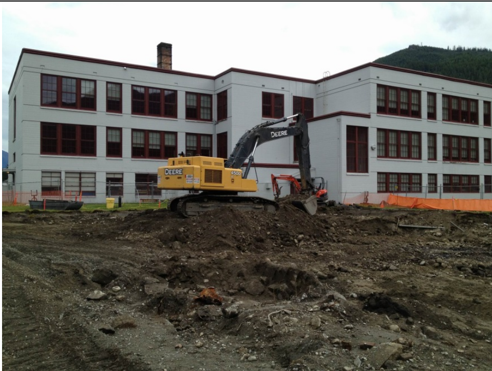
Photograph 1: Overview of foundation (in foreground), looking southeast to existing school.
