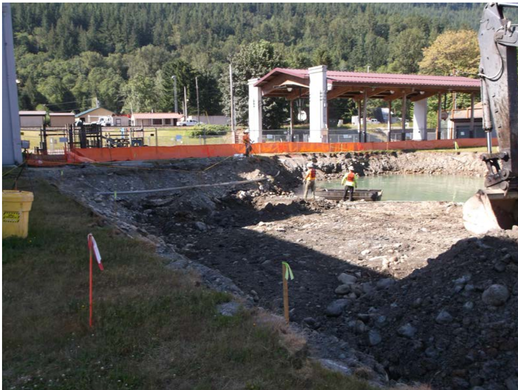
Photograph 7: Schoolyard excavation, looking south from grid location B14.
