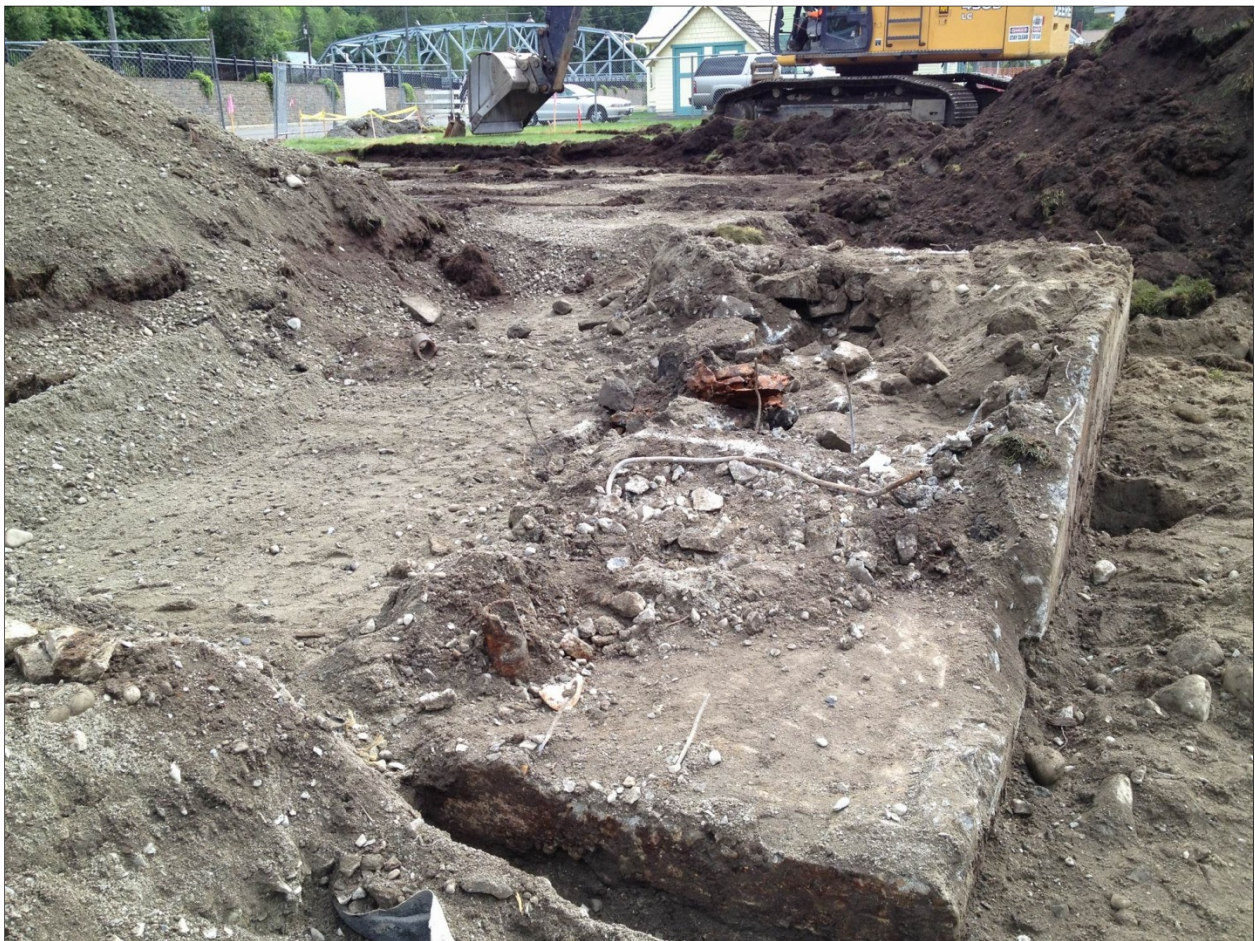
Figure 5-4. Overview photograph of partially cleared foundation remnants (view to northeast).
