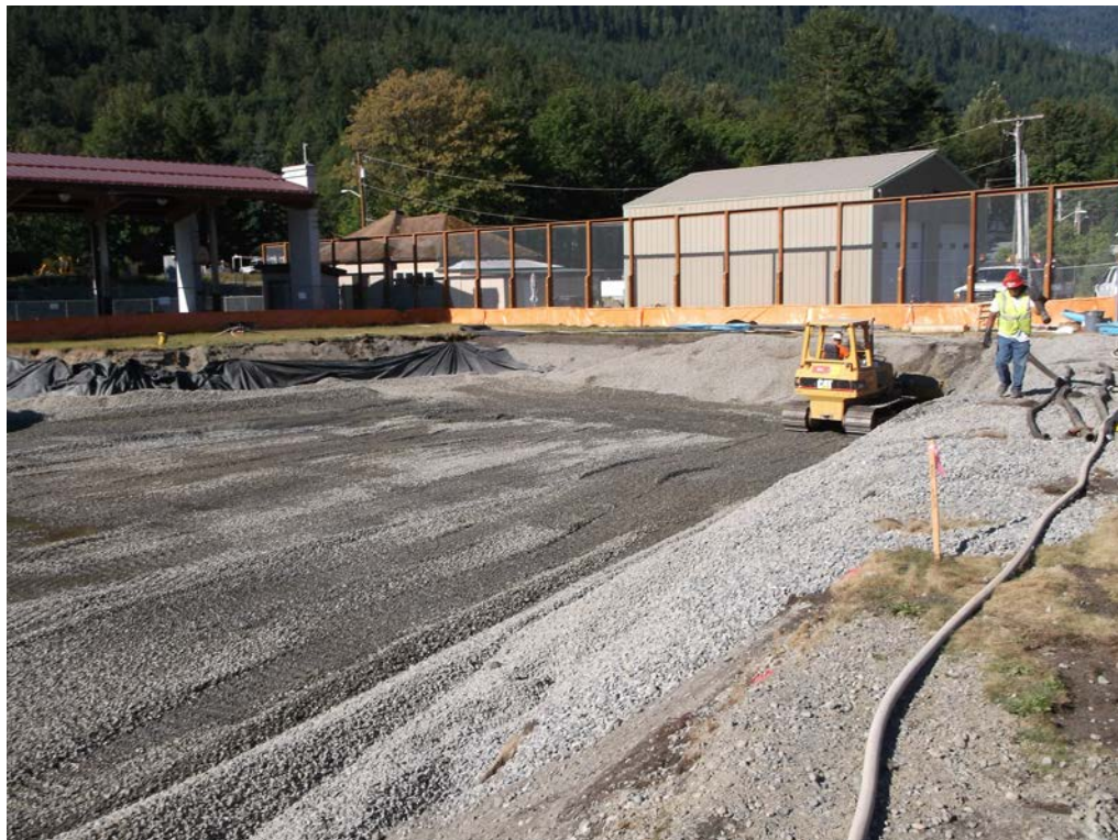
Photograph 13: Stabilization backfill activities, looking southwest from grid location B12.
