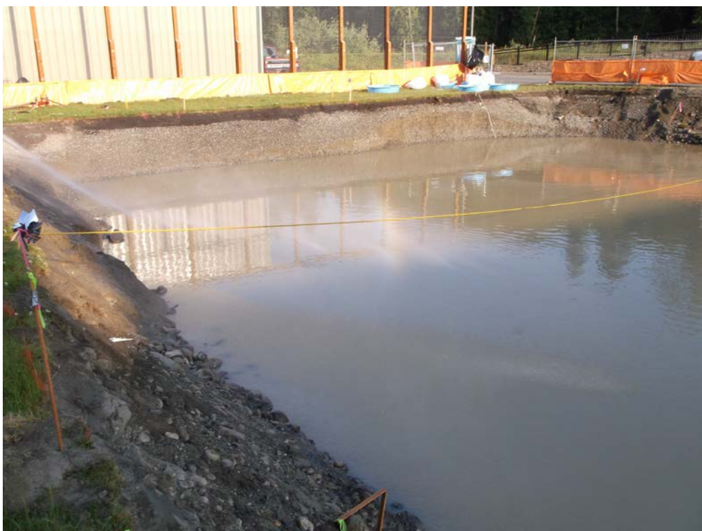
Photograph 6: Excavation looking west from grid location G12.
