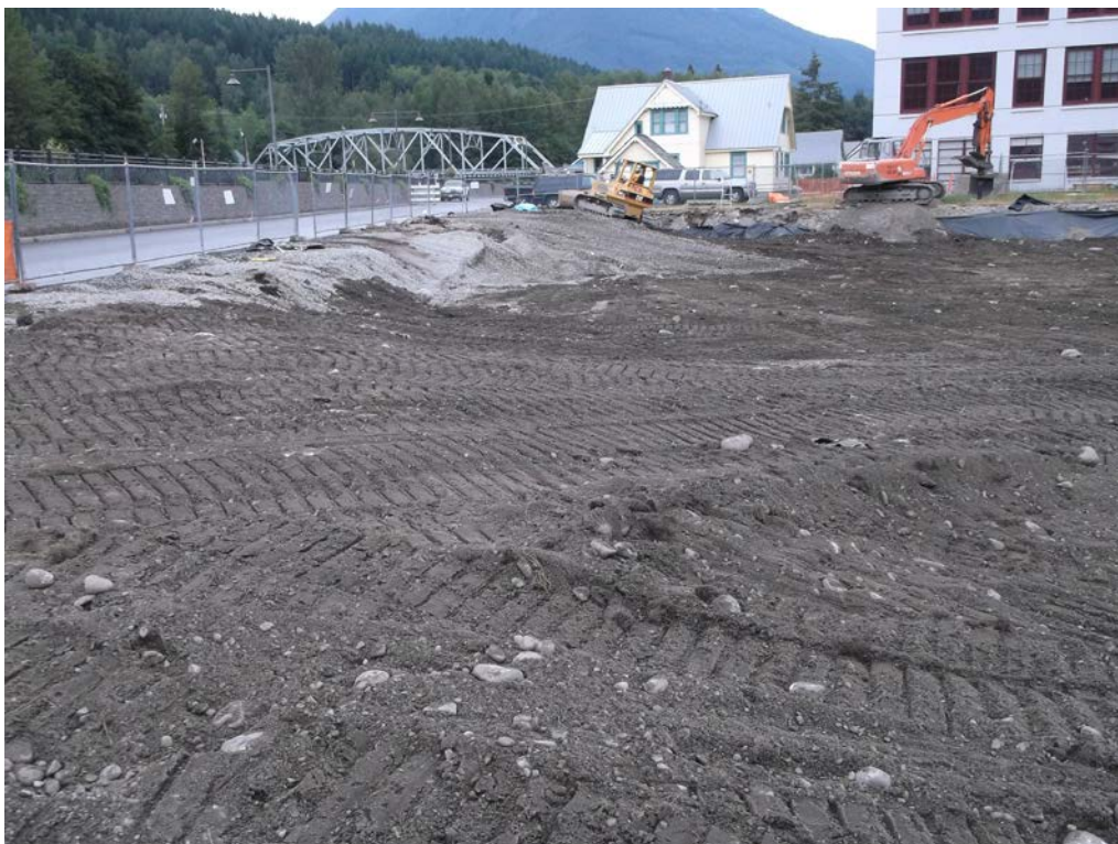
Photograph 15: Overburden backfill activities, looking east from grid location C8.
