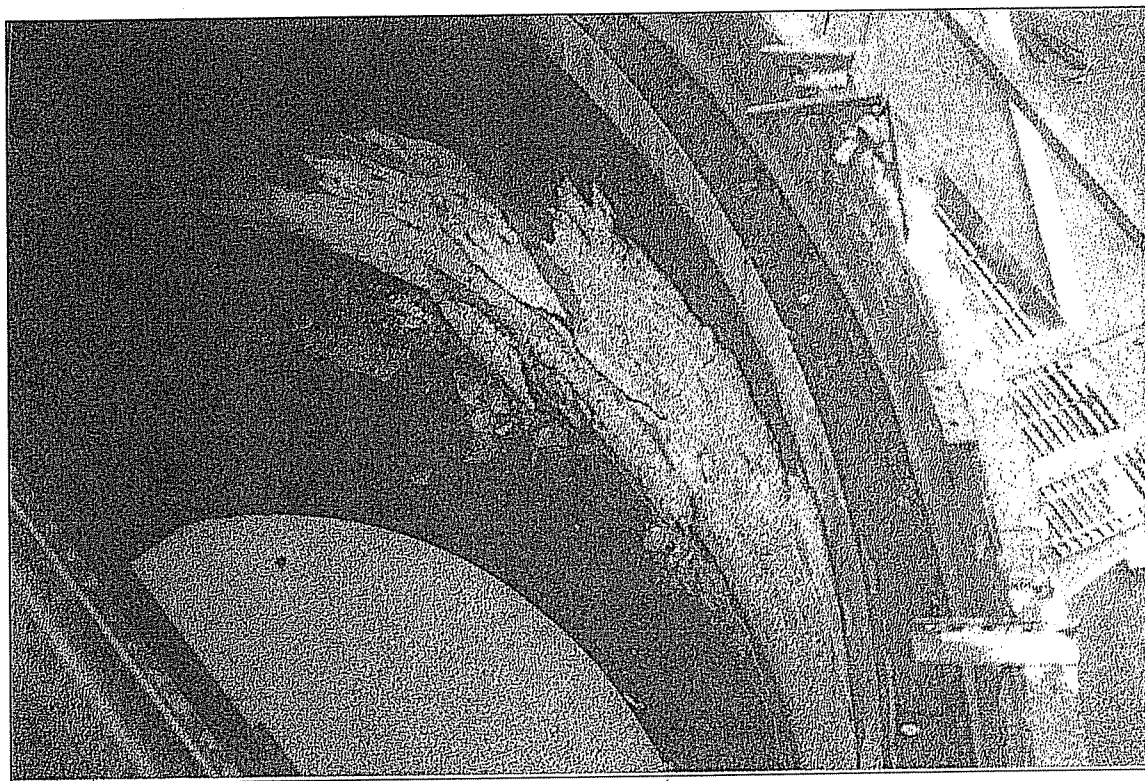
2. Interior condition of the treatment tank prior to closure activities.
