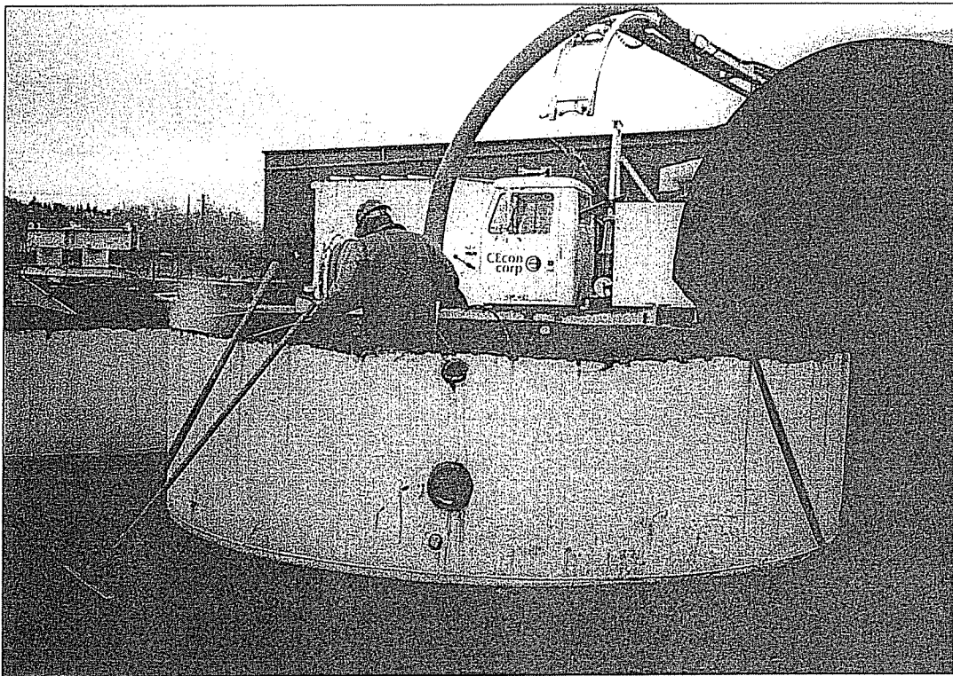
9. Leachate removal in bottom of surge tanks.
