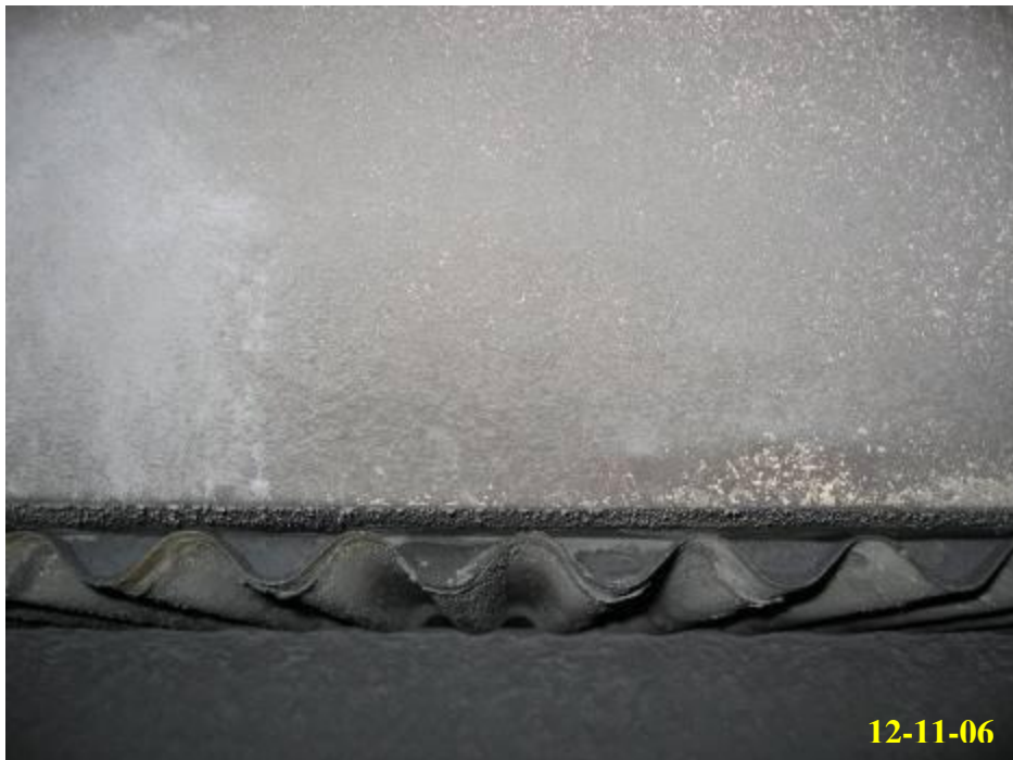
6.6 - Roof vent joint prior to cleaning
