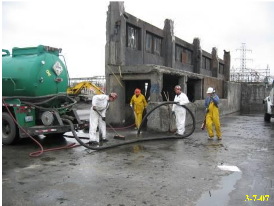
6.30 - Washing/cleanup vacuuming of floor under east mezzanine
