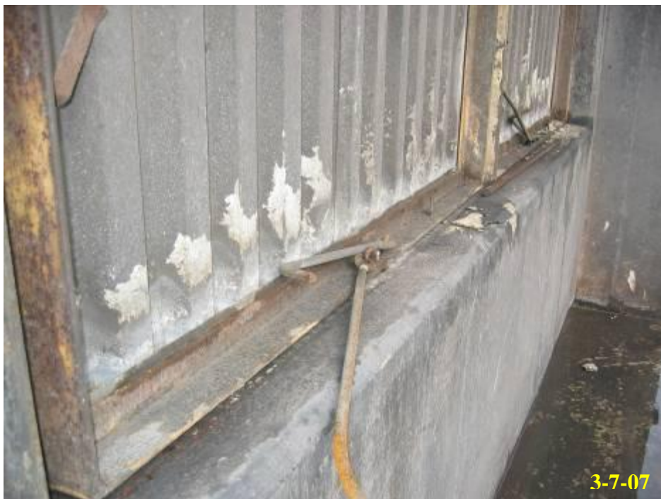
6.36 - Wall louver area after final cleaning
