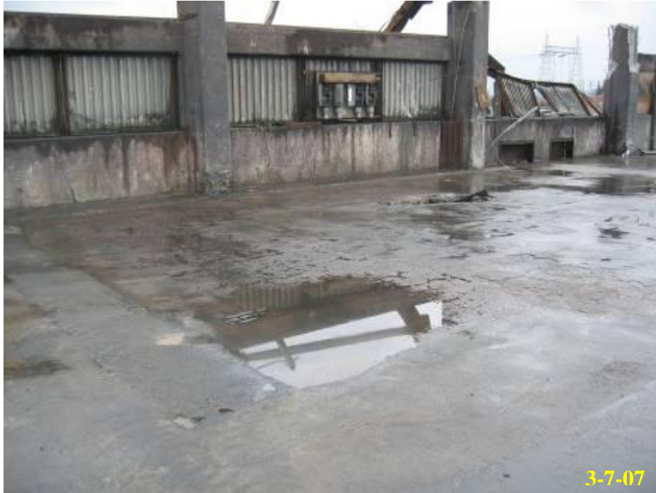
6.35 - North mezzanine floor after final cleanup
