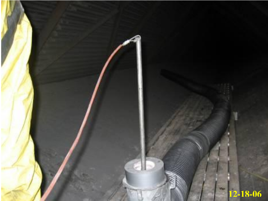
6.7 - Roof vent interior prior to cleaning
