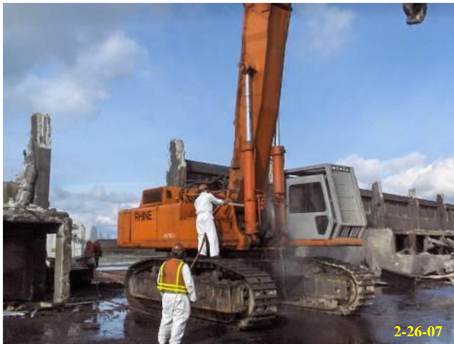
6.44 - Decontamination of equipment (typical)
