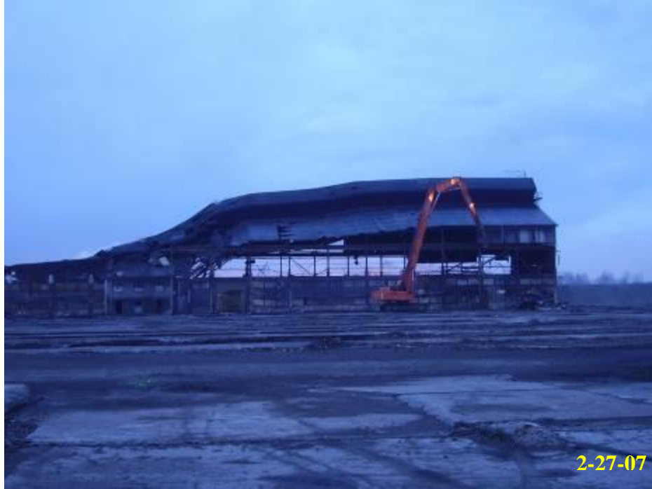
6.41 - Demolition of building siding/columns
