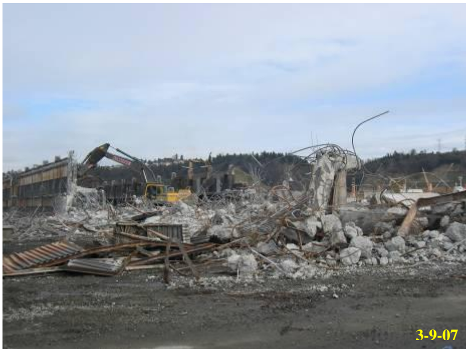
6.46 - Demolition of west concrete walls
