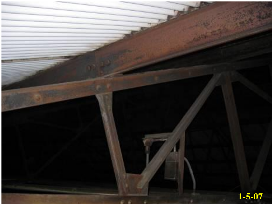
6.32 - Building trusses after final cleaning
