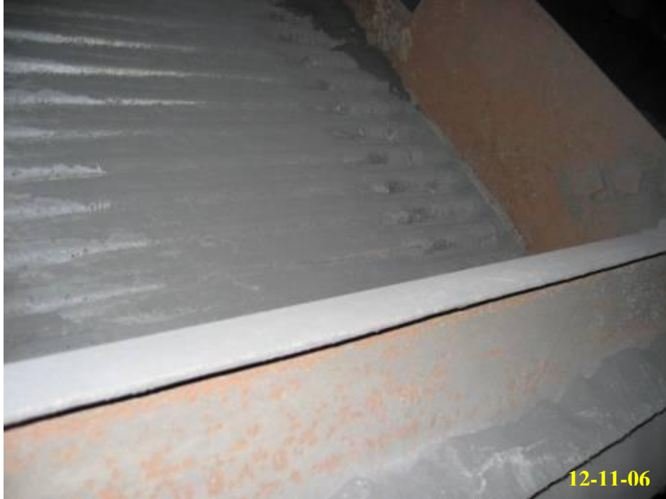
6.5 - Roof to vent structure prior to cleaning
