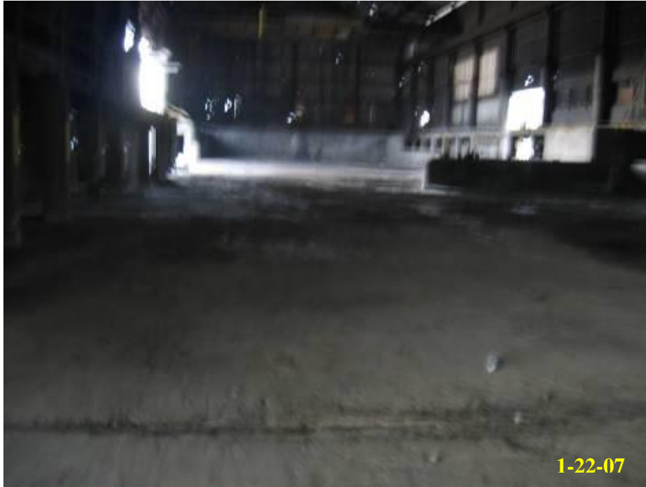
6.15 - Floor during cleaning
