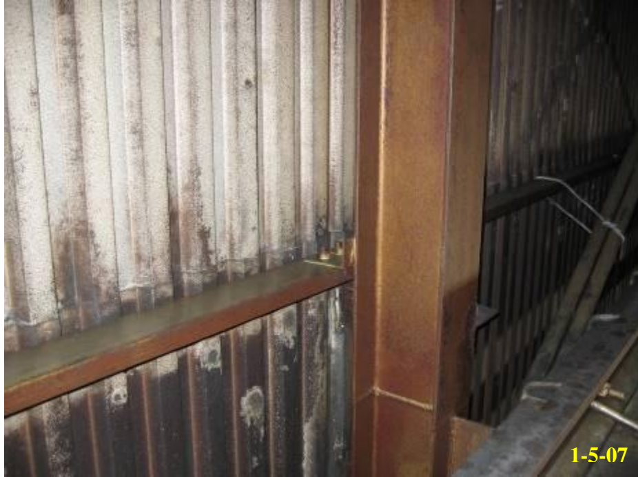
6.33 - Building wall structural after final cleaning
