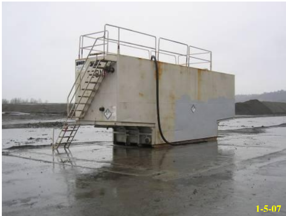
6.48 - First rented tank used for waste wash water storage
