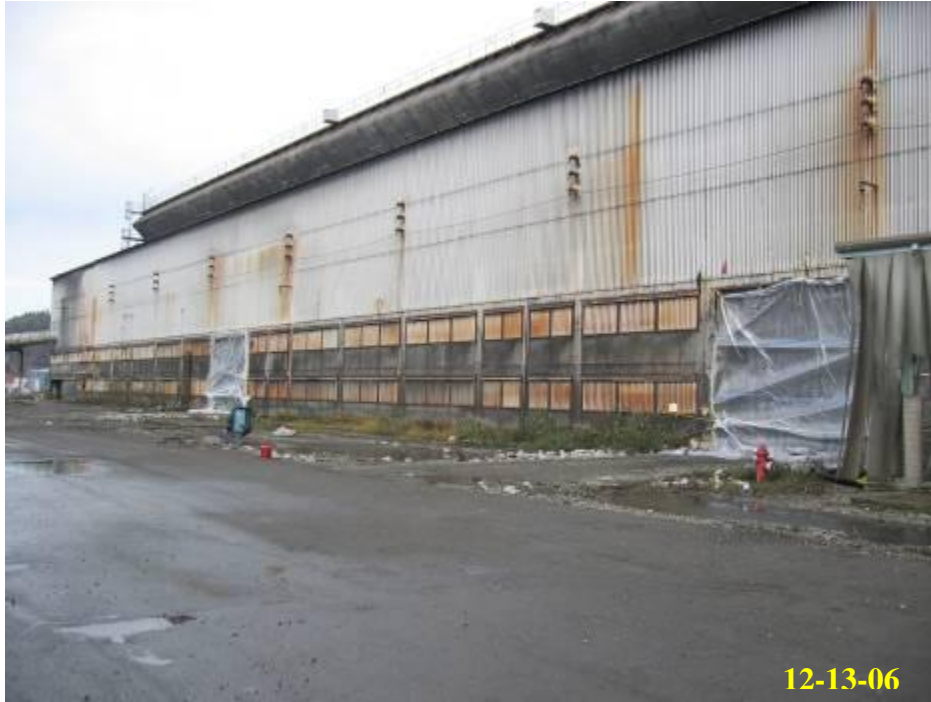
6.11 - Doorway sealing during building cleaning
