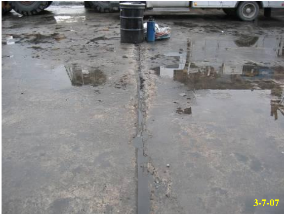
6.39 - Floor of main building after final cleaning
