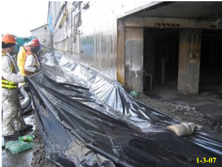
6.23 – Wash water containment management during washing of wall interior
