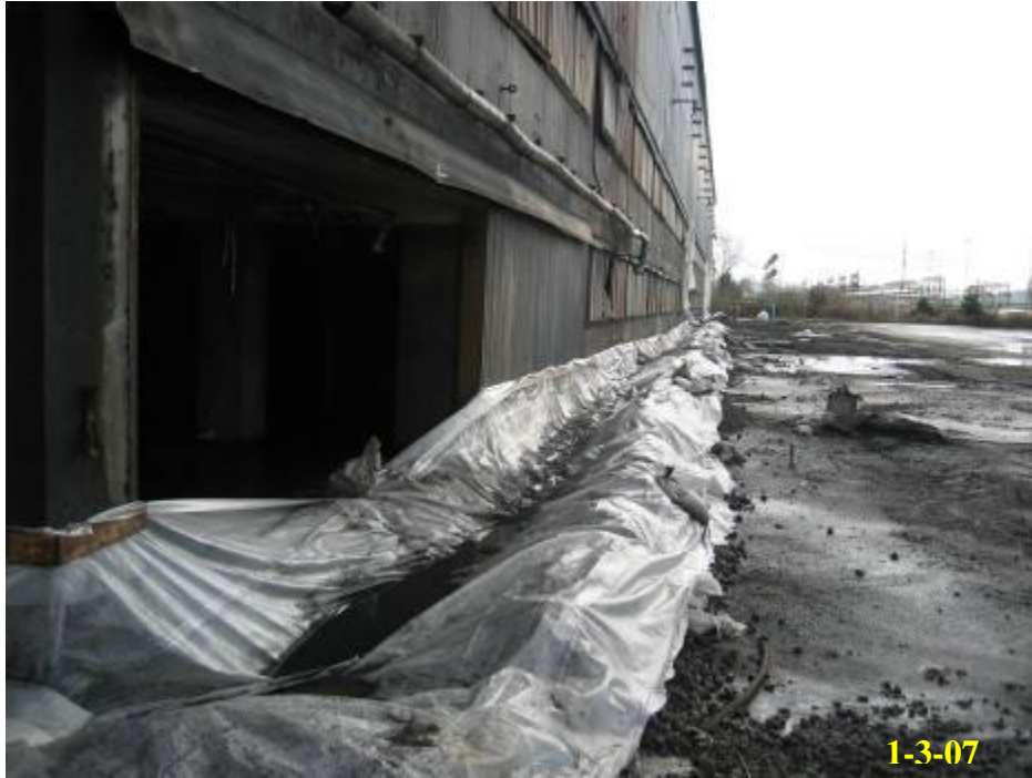
6.17 – Wash water containment berm constructed around building
