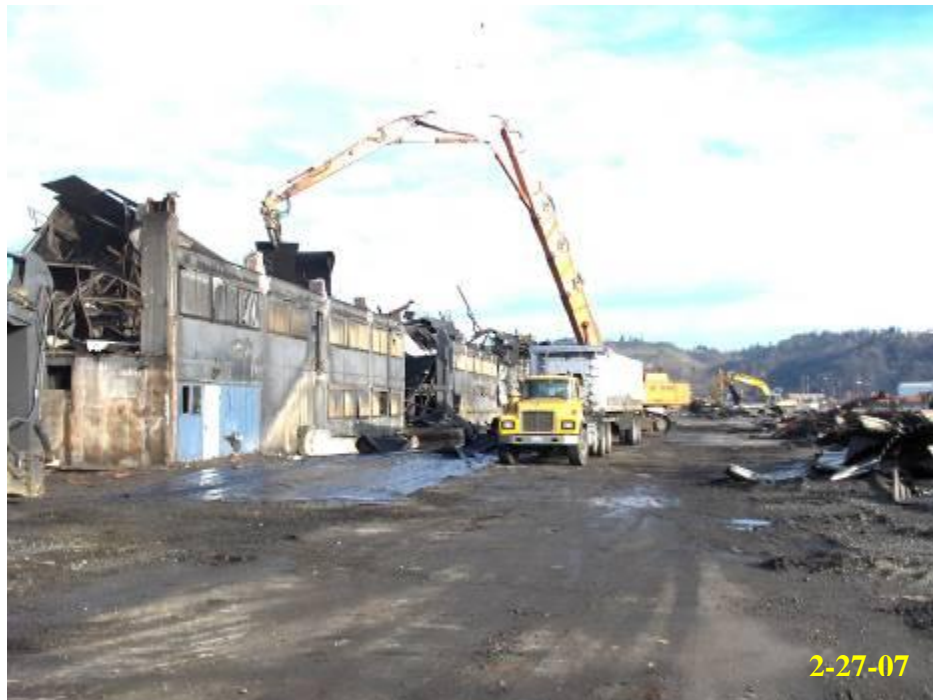
6.42 - Metal processing and loading of roof panels for disposal
