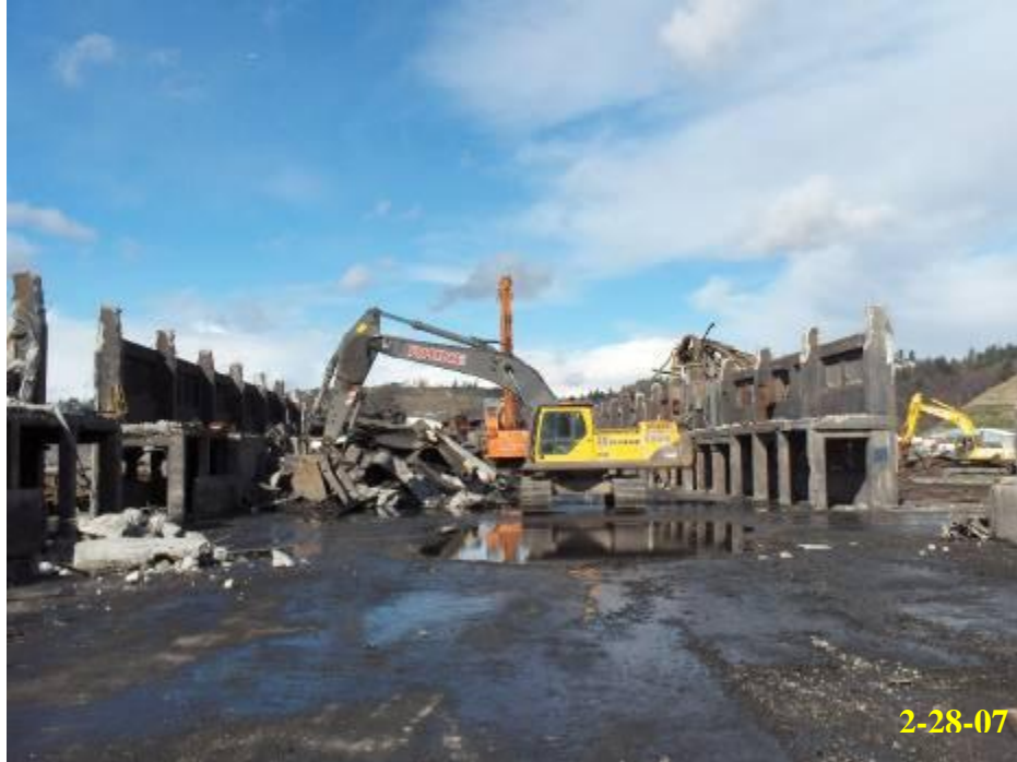
6.43 - Metal processing during building demolition
