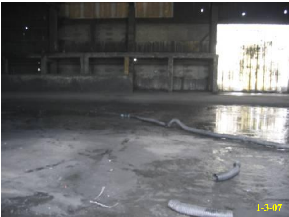
6.26 - Typical wash water vacuuming from floor during building washing
