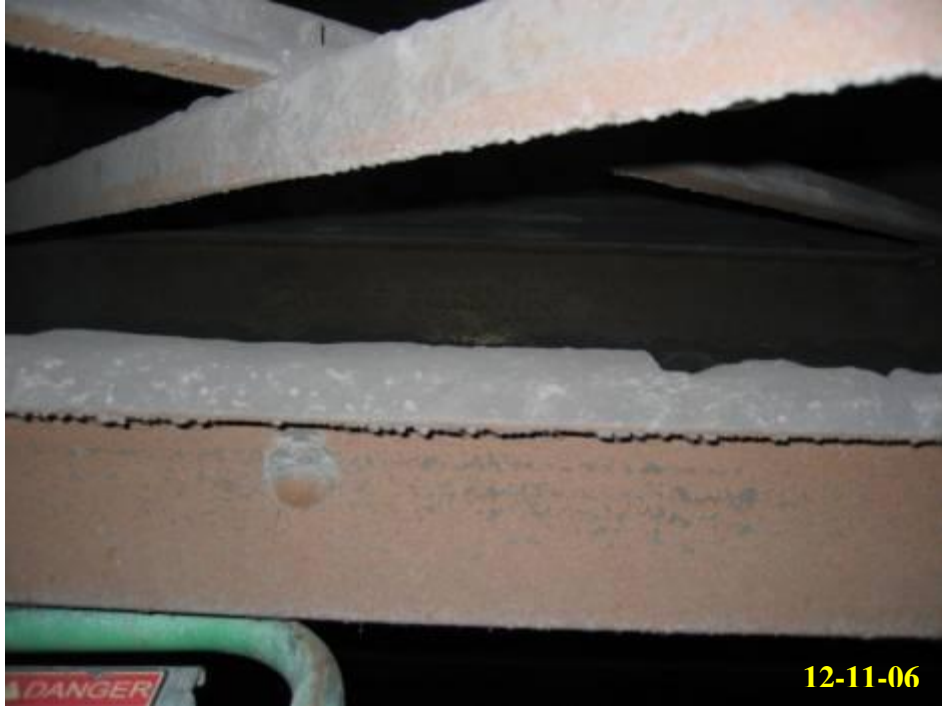
6.3 - Trusses prior to cleaning
