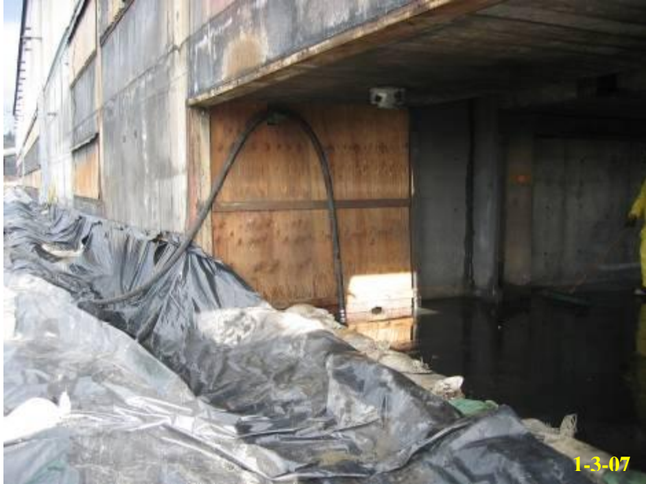
6.27 – Wash water vacuuming/containment (typical)
