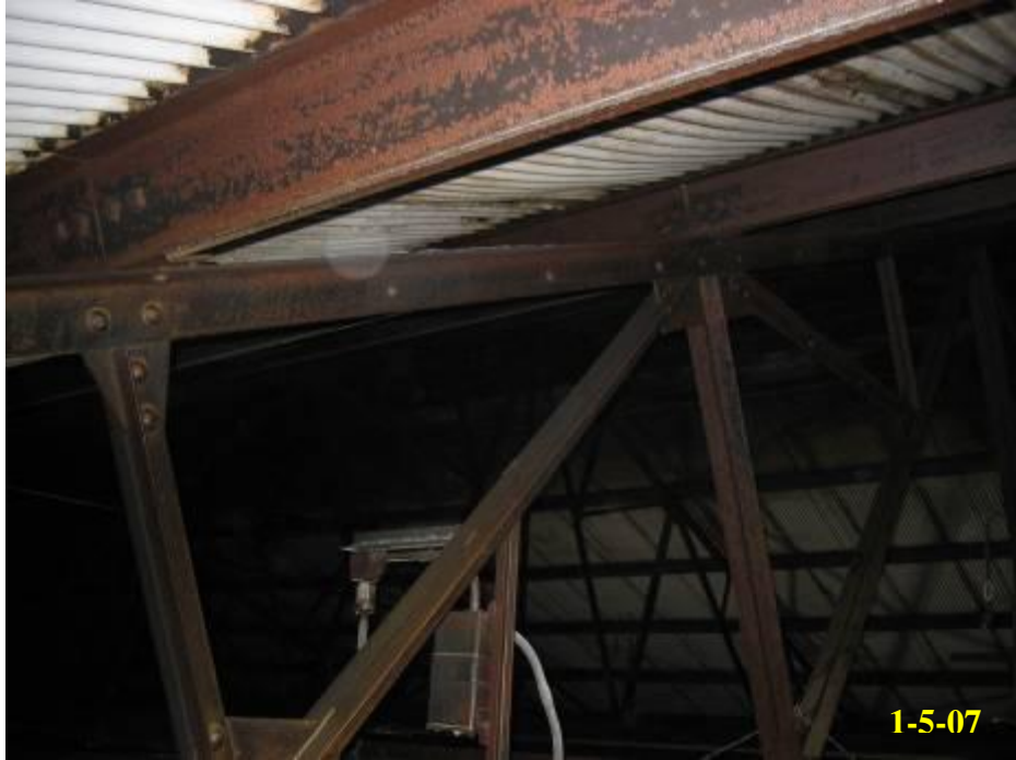
6.21 - Roof trusses during washing
