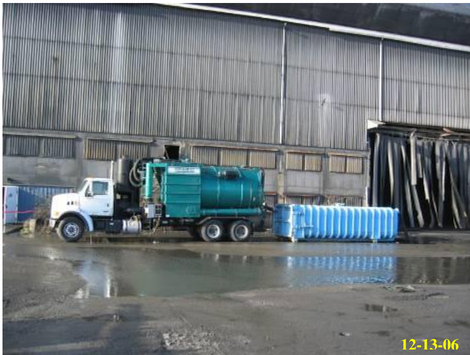
6.16 - Vacuum truck and dust enclosure type roll-off box during vacuuming
