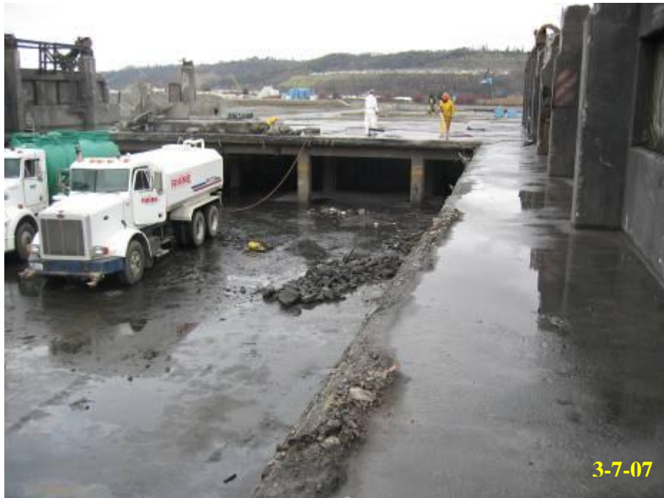
6.28 - Washing of north mezzanine floor
