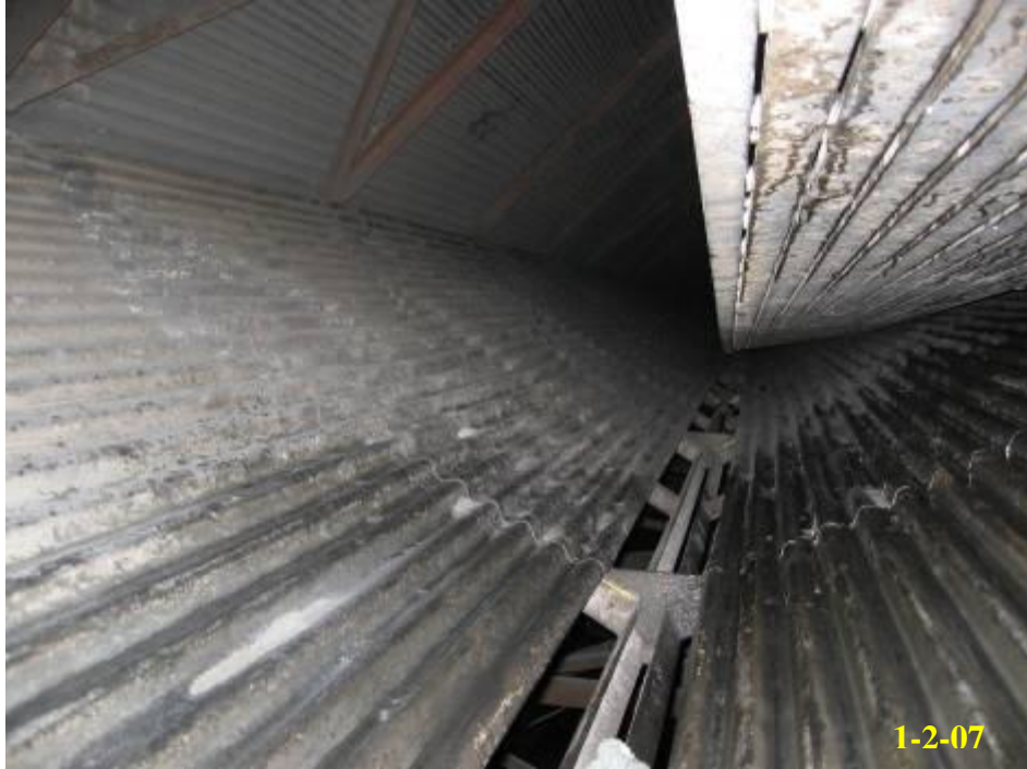
6.31 - Roof vent interior after final cleaning
