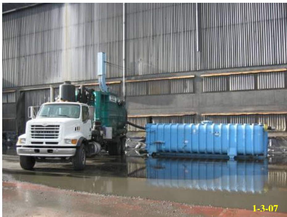
6.24 - Vacuum truck staging during building washing
