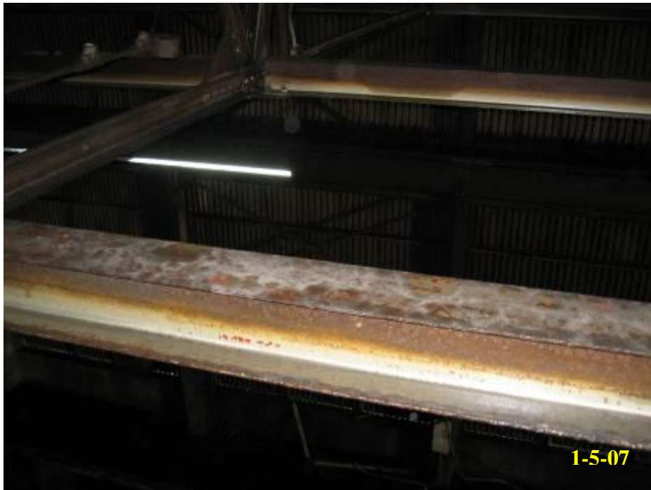
6.34 - Typical roof structural after cleaning
