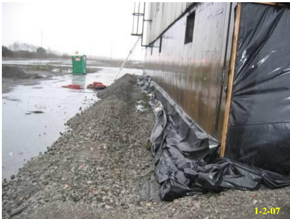
6.18 – Wash water containment berm showing attachment of Visqueen to building wall
