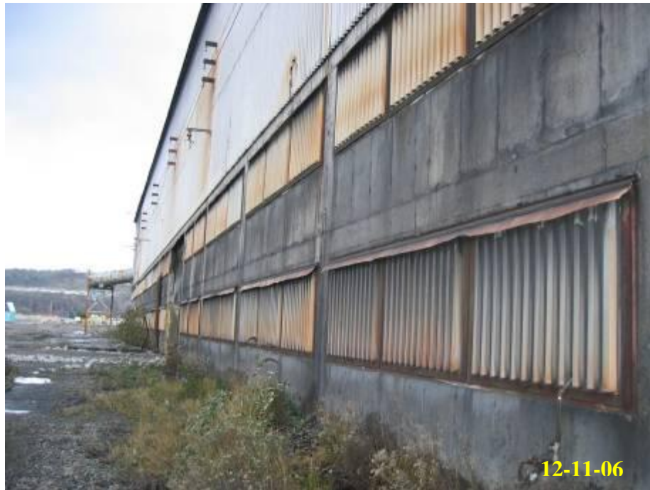
6.1 - West exterior of building prior to construction of wash water containment
