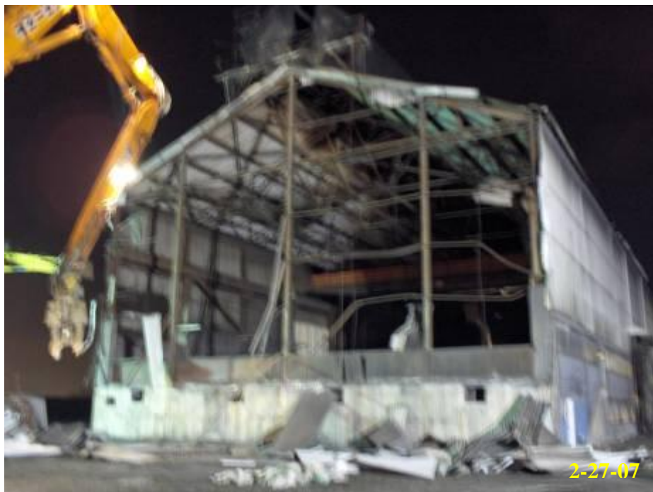
6.40 - Start of building demolition at south end
