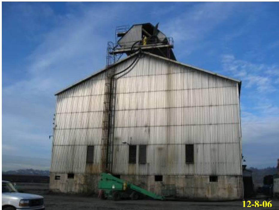
6.12 - Vacuuming of roof vent interior at south end of building
