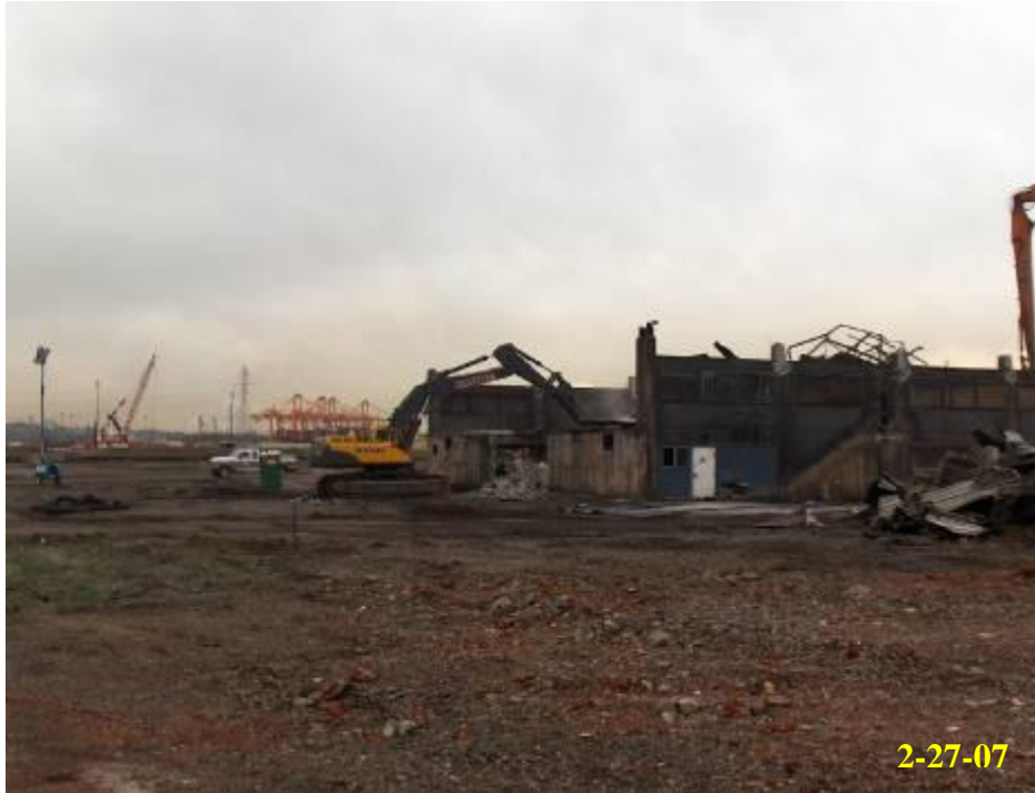
6.45 - Beginning of concrete wall demolition at south end
