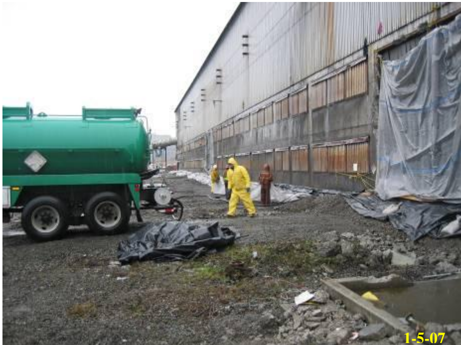
6.22 - Typical vacuuming of wash water from containment during washing
