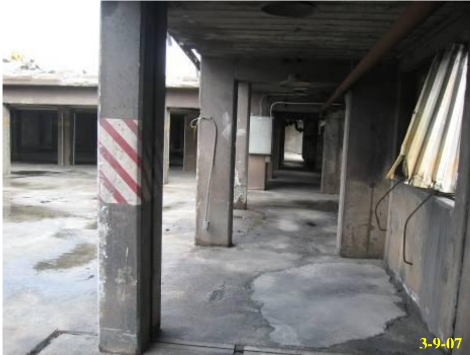
6.37 - Floor under NW mezzanine after final cleanup
