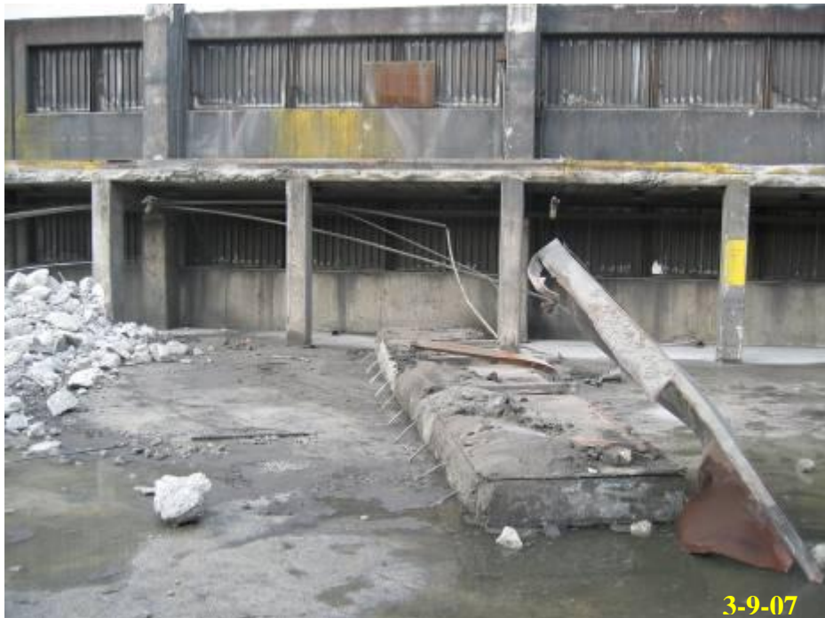
6.10 - Interior building divider prior to cleaning
