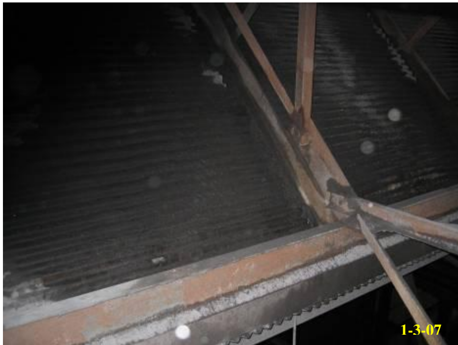
6.4 - Vent to roof joint prior to cleaning
