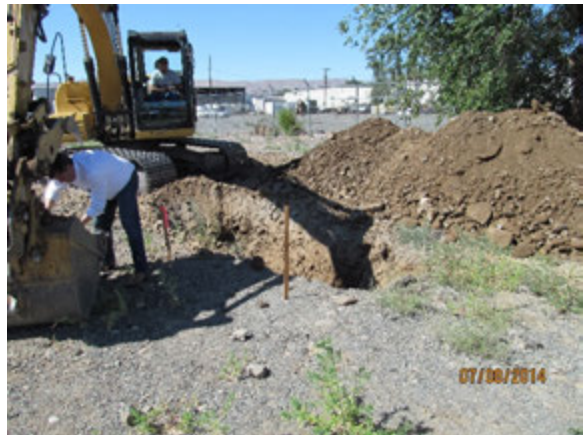
Excavation at North Drywell/PCS area.
