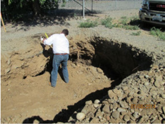
Excavation at Oil Release area.
