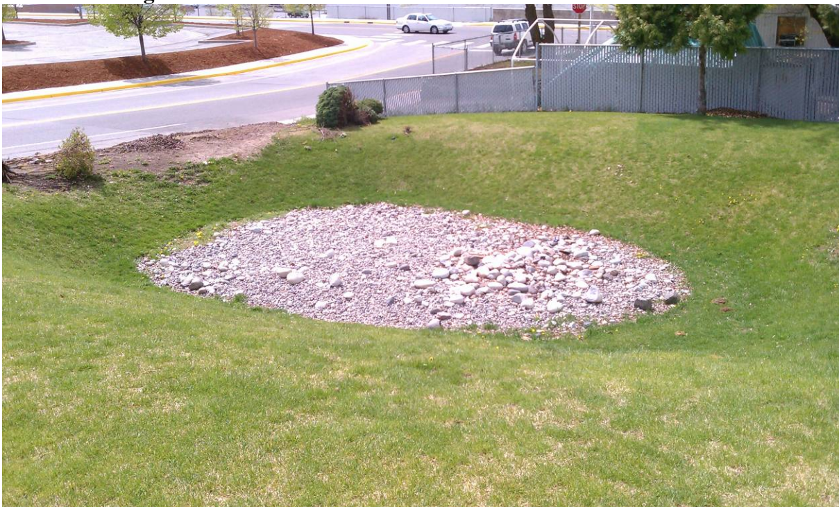
Photo 4: Drainage Swale - from northwest
