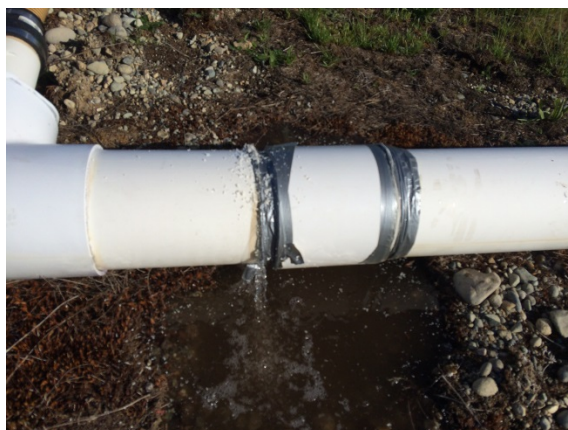
Before header repair at well E-42
