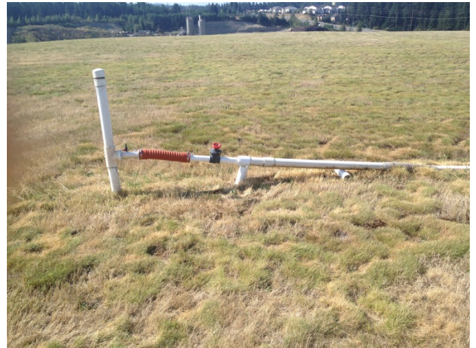
N37 after valve replacement.
