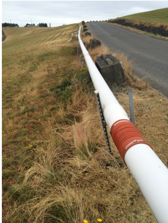
After collapsed header repair between wells N-29 and N-30
