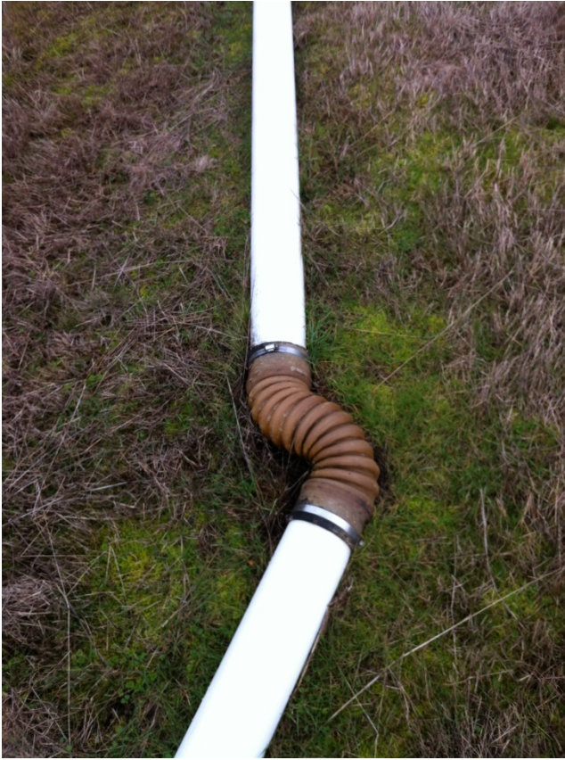
E-39 Lateral Line Repair
