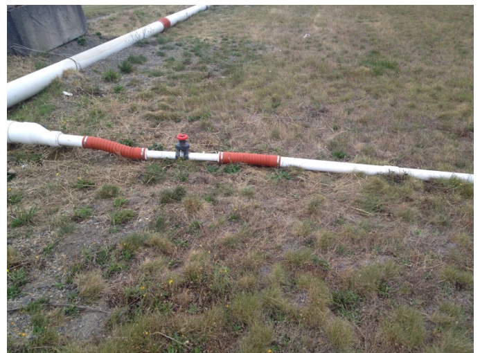
N27 after repair of lateral.
