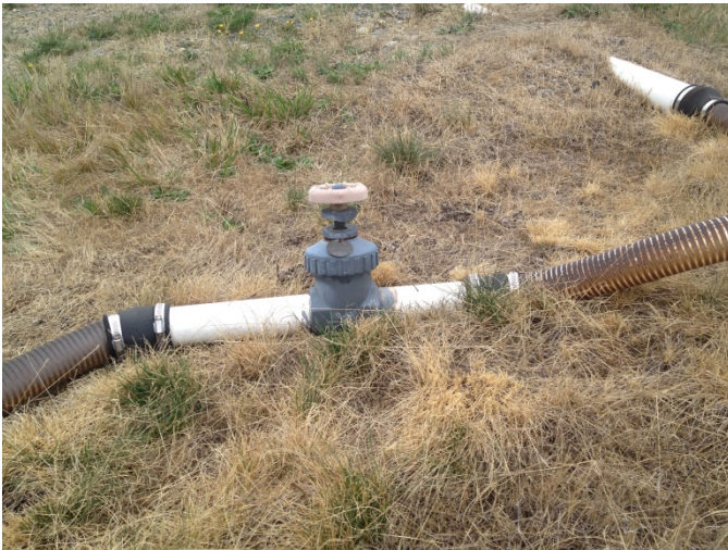
N66 before valve replacement.
