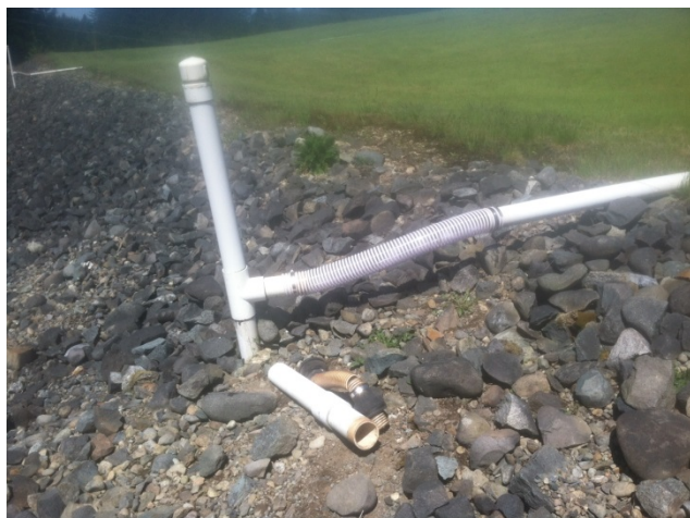
After flexible PVC replacement at wells N-39 & N-56
