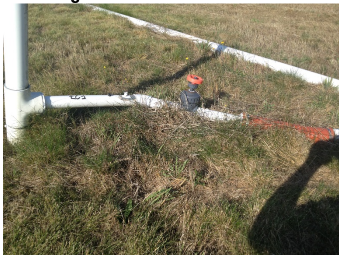
E27 before valve replacement.
