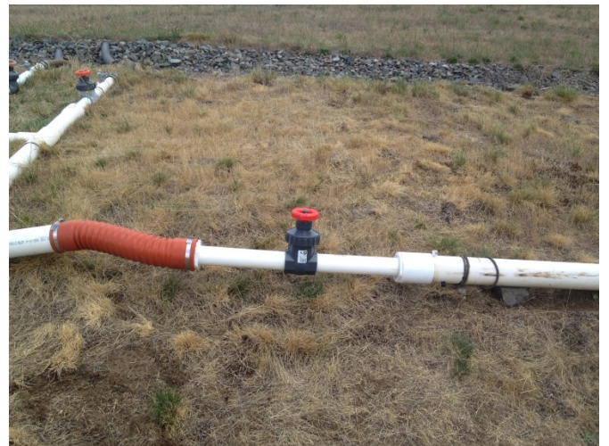
N66 after valve replacement.
