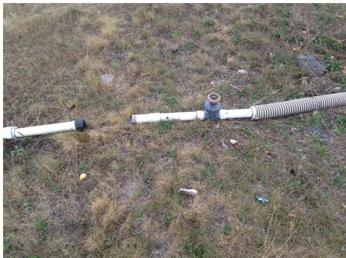
N63 before pipe replacement.
