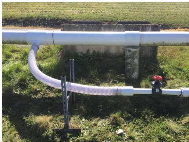
After flexible PVC replacement at wells N-39 & N-56
