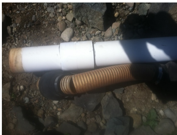
Before flexible PVC replacement at wells N-39 & N-56
