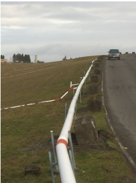
8-Inch Header Pipe repaired
