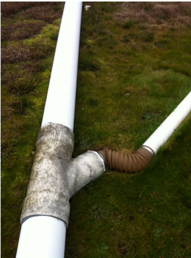
E-41 Flex Hose Repair
