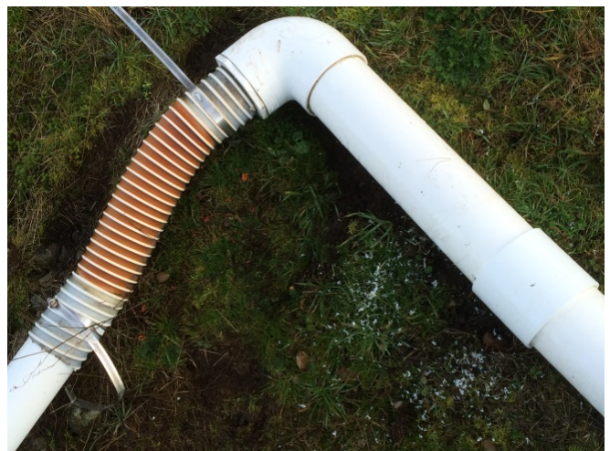
10-inch diameter header relocation between N-33 & N-36.
