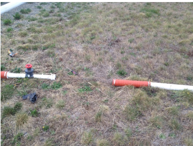
N27 pre-repair of lateral.
