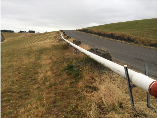
After collapsed header repair between wells N-29 and N-30
