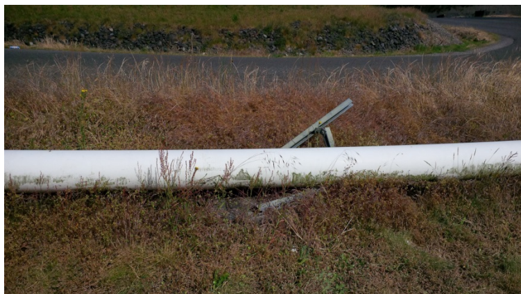
Before collapsed header repair between wells N-29 and N-30
