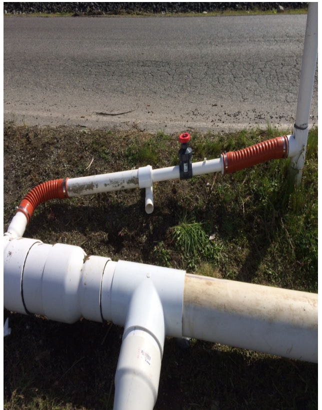
Wells N-27 & N-28 wellhead repairs
