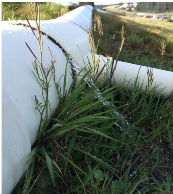
Before header repair between wells N-27 & N-28
