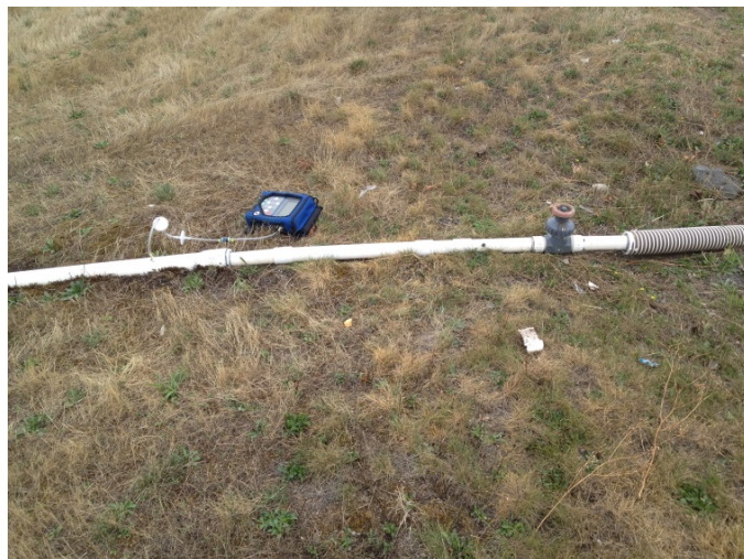
N63 after pipe replacement.
