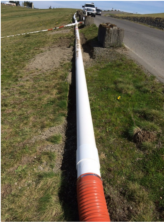
After header repair between wells N-27 & N-28
