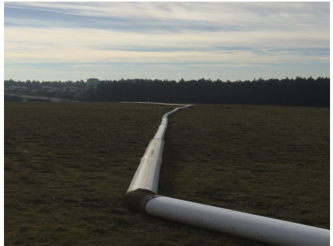
10-inch diameter header relocation between N-33 & N-36.
