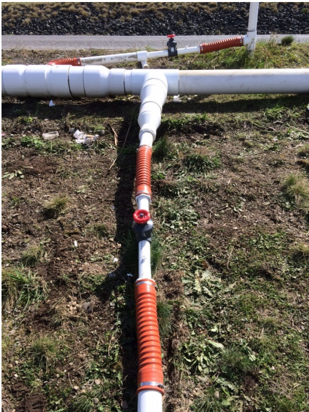
Wells N-27 & N-28 wellhead repairs
