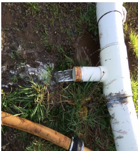
Before header repair between wells N-27 & N-28
