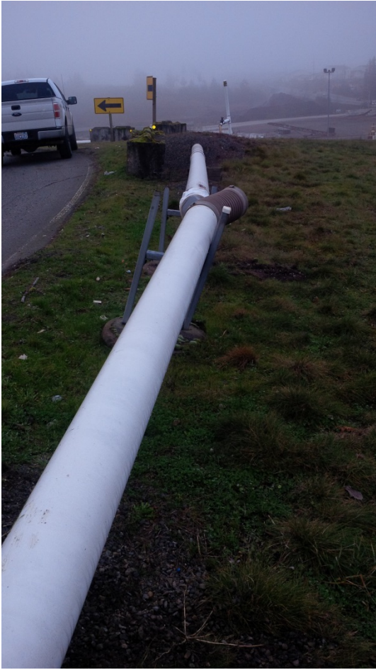
8-Inch Header Pipe damaged by a vehicle
