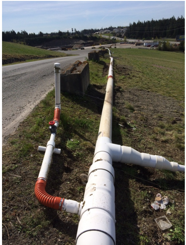
After header repair between wells N-27 & N-28
