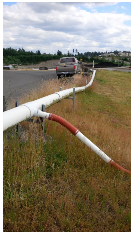
Before collapsed header repair between wells N-29 and N-30
