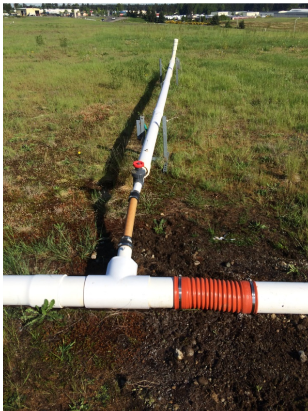
After header repair at well E-42
