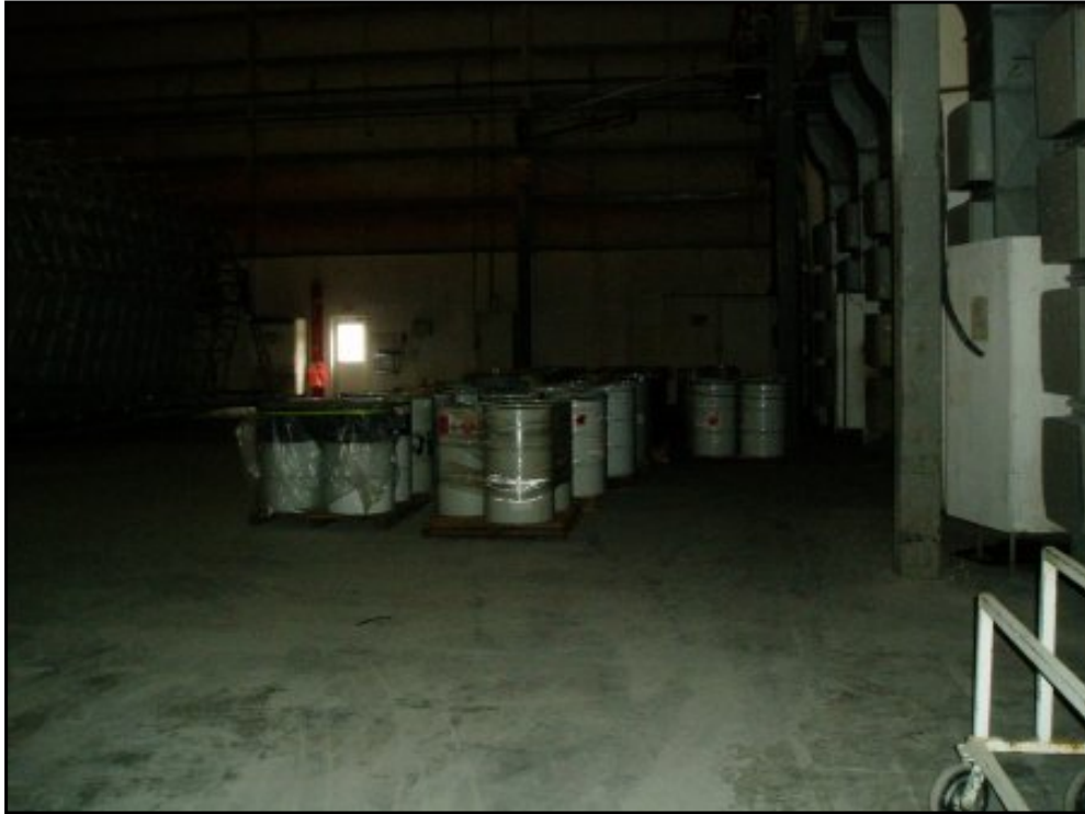
View of hazardous materials stored in Building 16.
