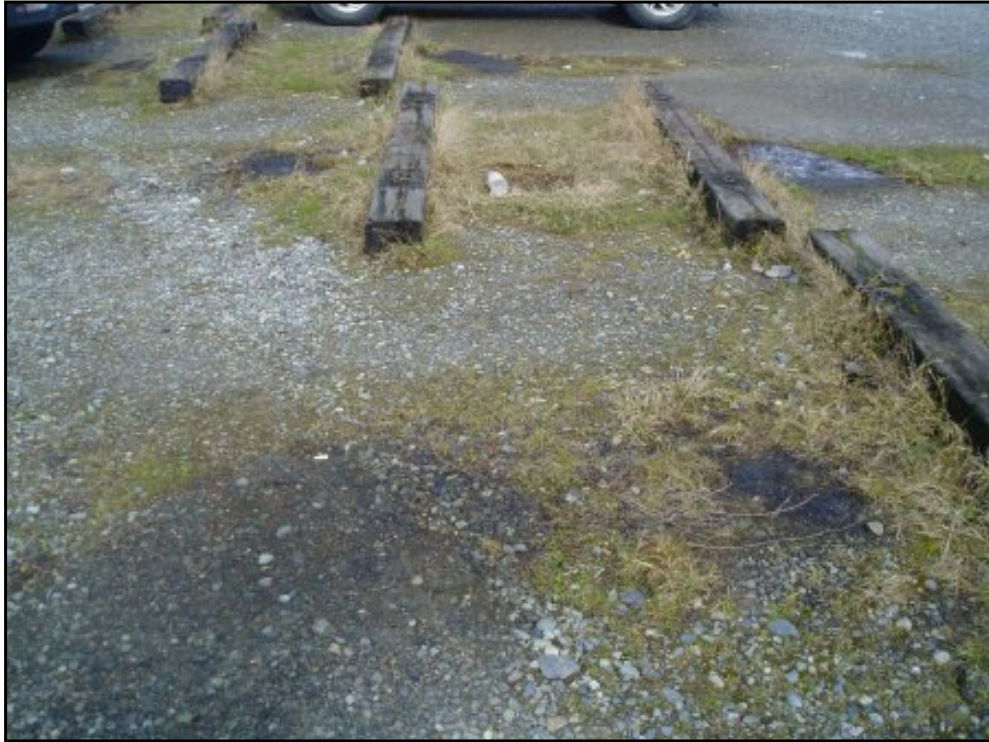
View of typical oily stained gravel observed in the employee parking lot on the east side of the subject property.
