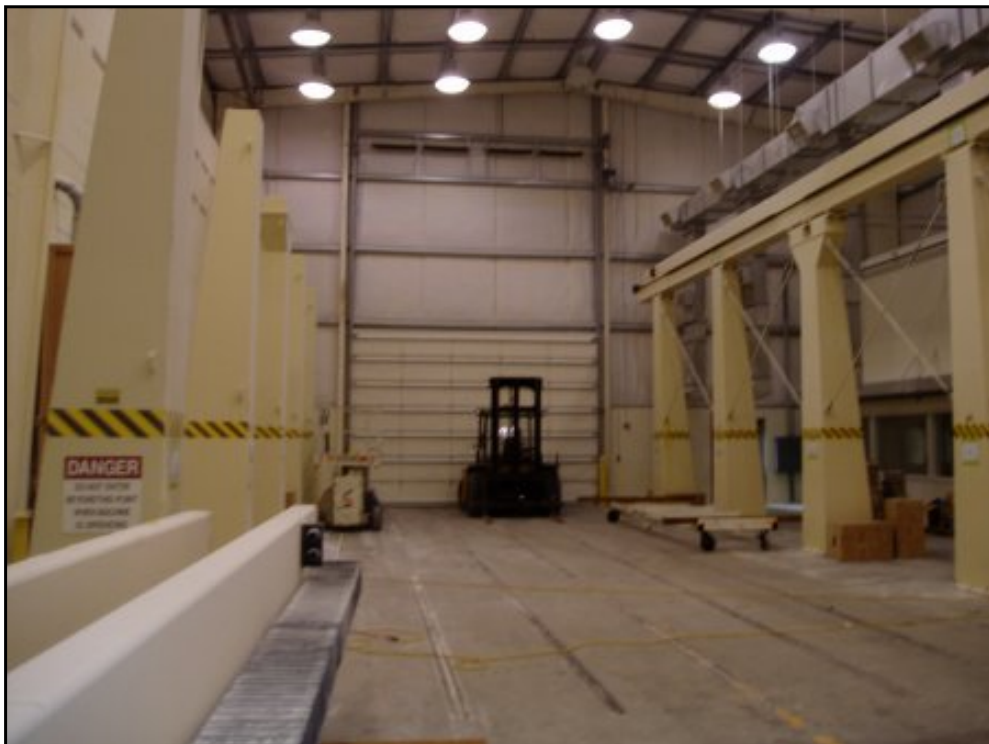
View of Building 12A, the former foam cutting building.
