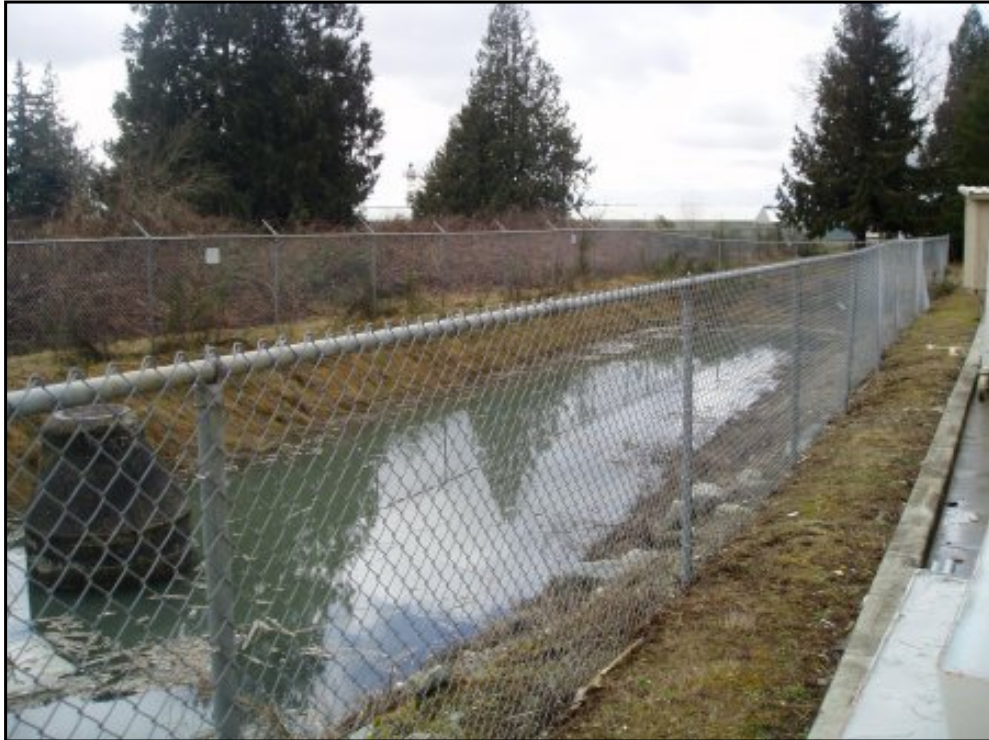
View of retention pond one located southwest of Building 16.
