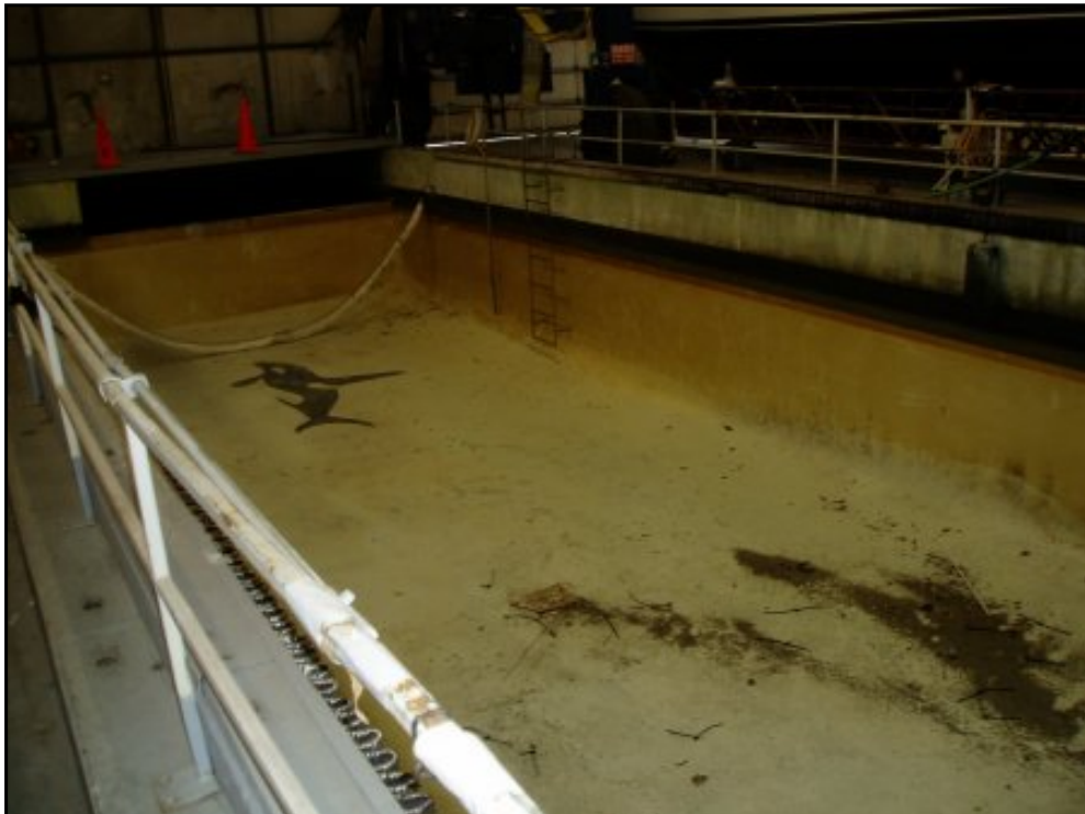
View of the testing pool in Building 4.
