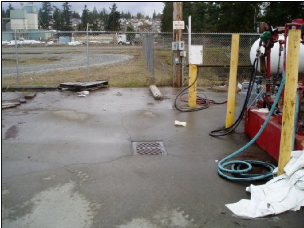
View of a stormwater drain and the diesel and gasoline dispenser island located northeast of Building 14.
