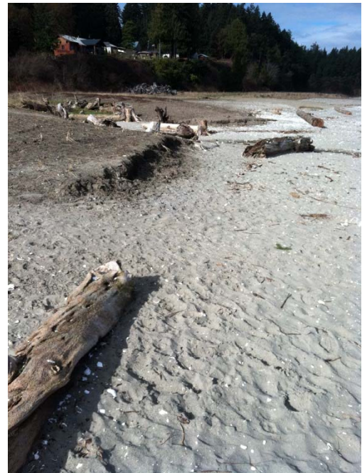
Photograph 11 King tides following shoreline LWD installation resulted in several logs being relocated.
