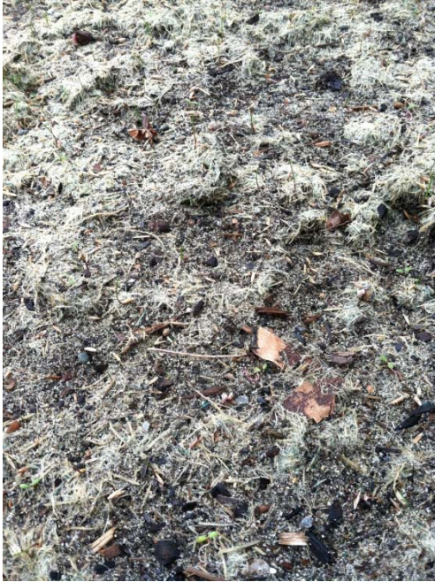
Photograph 1 Hydroseed area of upland soil cap showing new germination.
