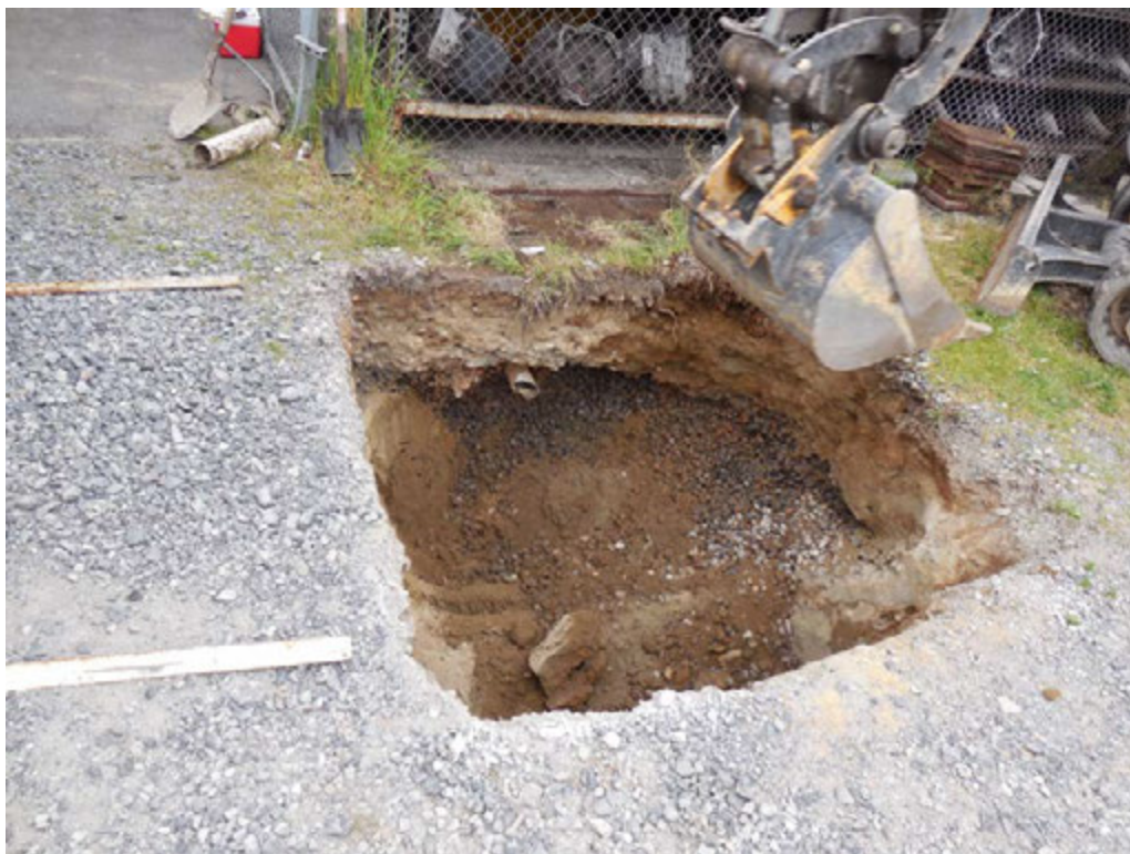
Photograph 1: Perforated drainpipe extending west from Site building.
