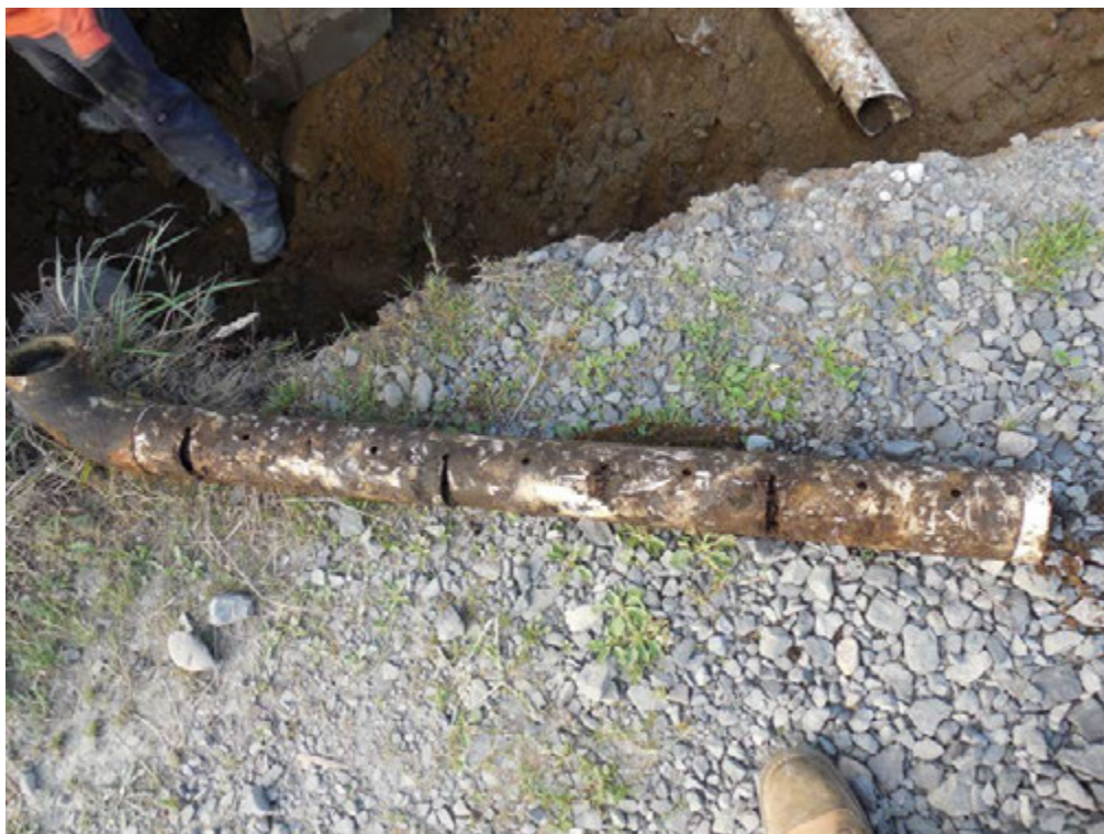
Photograph 5: Removed section of perforated drainpipe.
