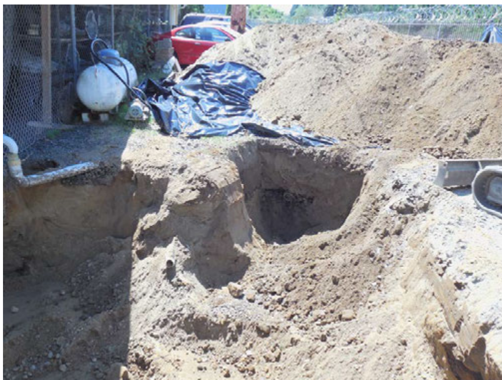
Photograph 6: Septic drainpipe and perforated drainpipe extending south.
