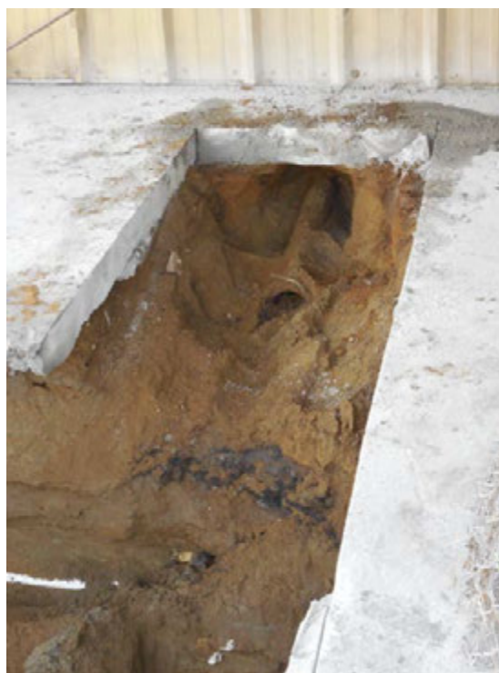
Photograph 2: Metal drainpipe extending west from unknown location inside the Site building that was connected to the perforated drainpipe.
