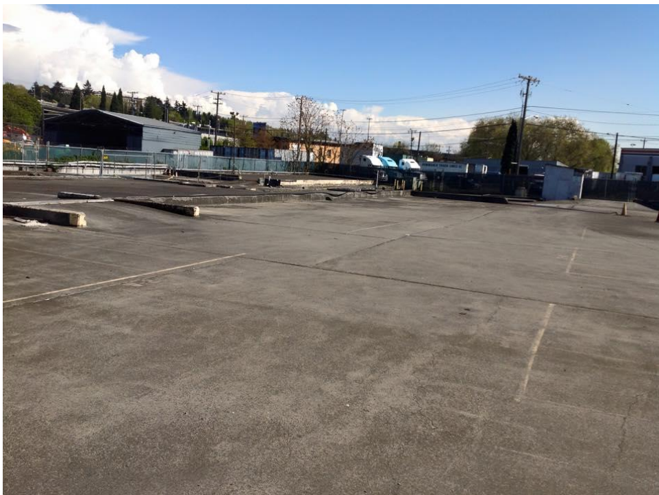
Photo 14: PSC facility property, looking southeast
