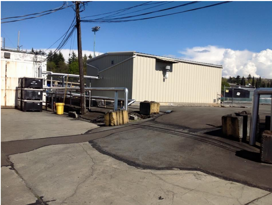
Photo 3: 5400 Denver property, looking east towards the groundwater extraction treatment building.
