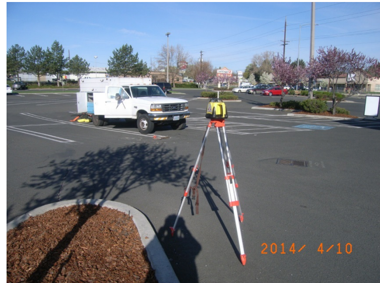
Surveying top-of-casing elevations for Safeway UST observation wells – view west.
